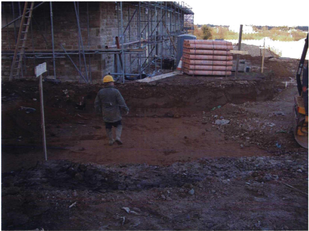
Plate 4. Stripping of Road. Facing North.
