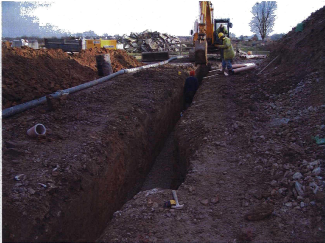
Plate 1. Service Trench. Facing East.
