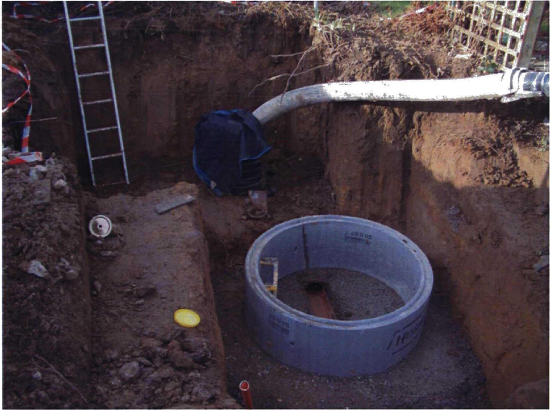
Plate 3. Manhole. Facing West.
