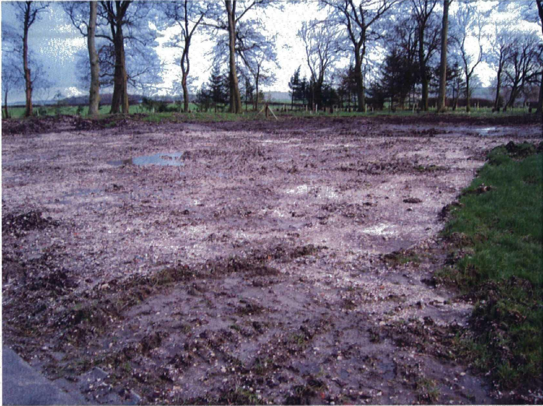
Plate 1. Pre-Excavation View of Site. Facing North East
