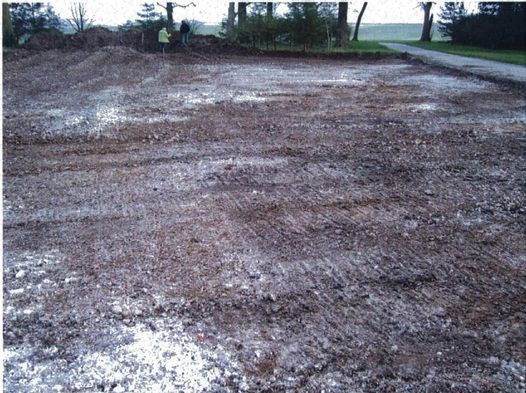
Plate 2. Site Strip. Facing South
