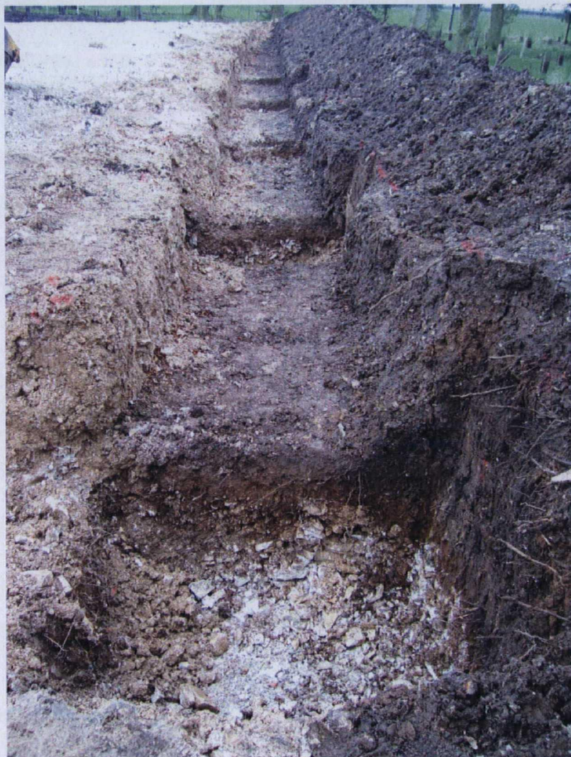
Plate 4. Stanchion Pits. Facing North
