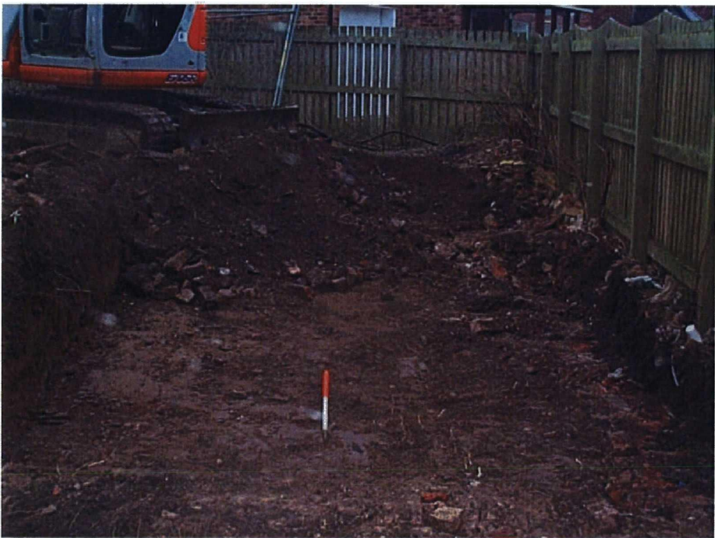
Plate 6. Foundation Strip. Facing South
