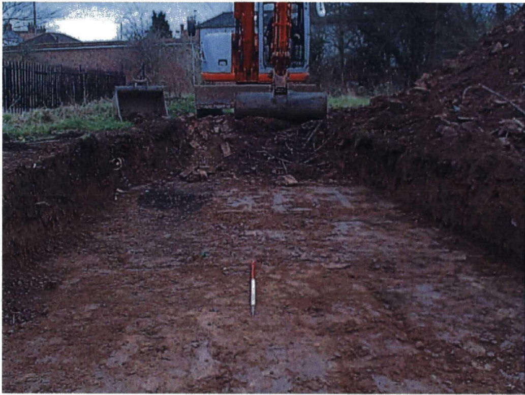
Plate 5. Foundation Strip. Facing East
