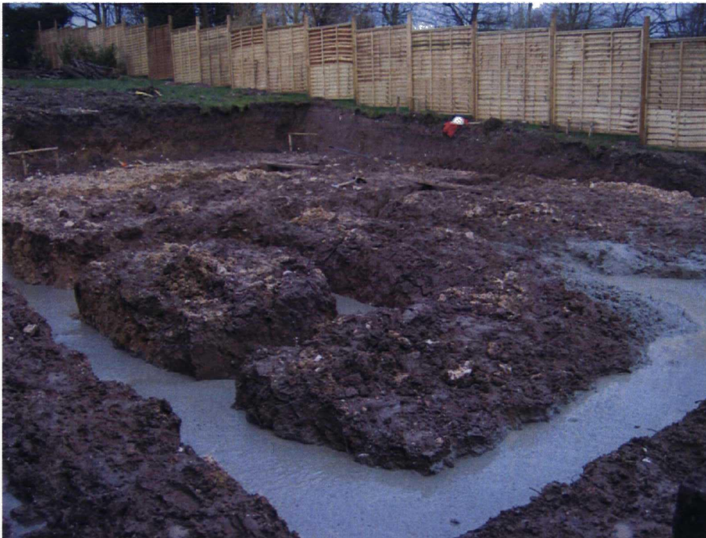
Plate 6. Completed House Footing Excavation. Facing North West
