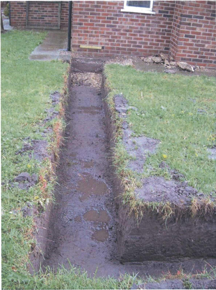
Plate 3. Western Foundation, Facing East.
