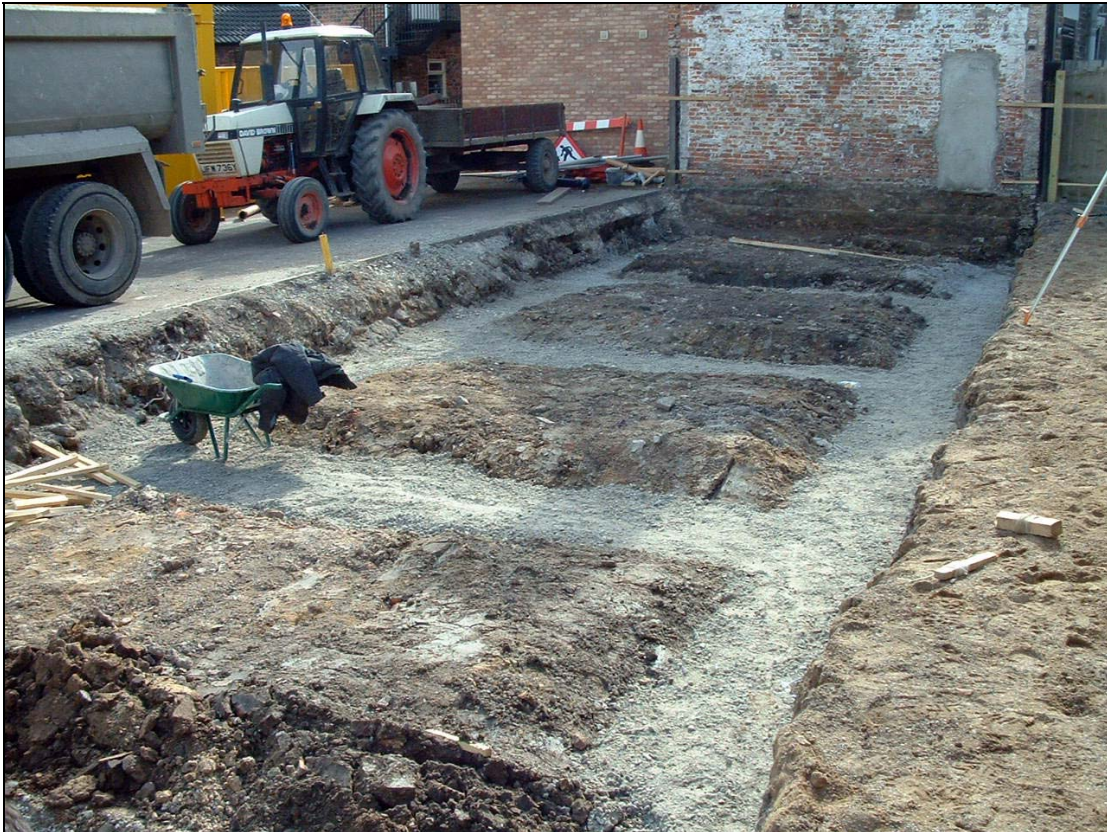
Plate 1. Photo showing the shallow nature of the raft foundation.
