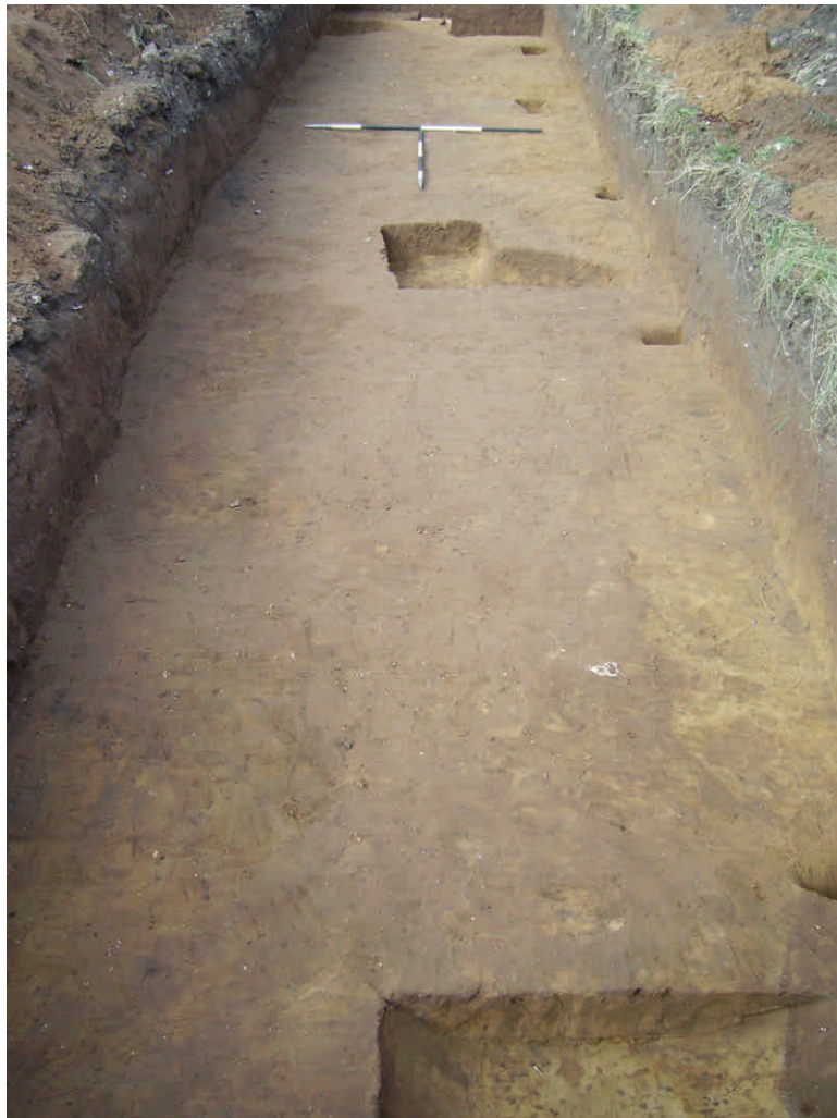
Plate 2. Trench 2 - Post-Excavation. Facing North
