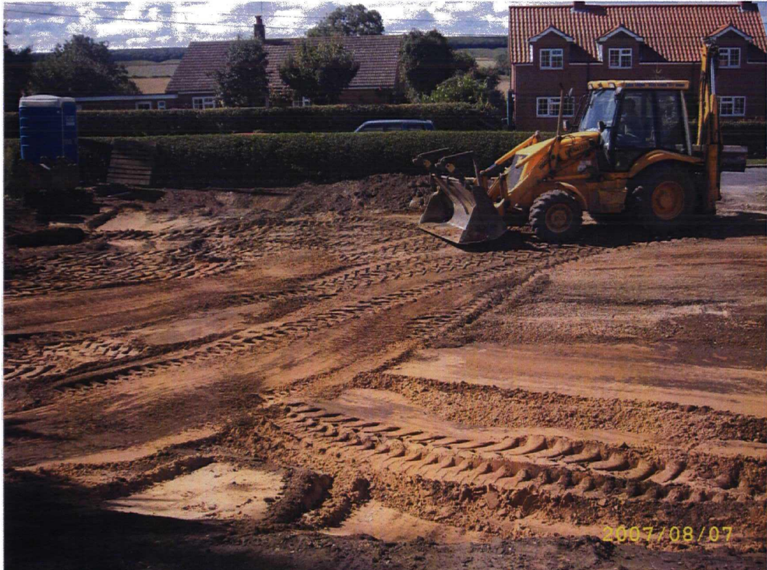
Plate 2. Area of proposed development following excavation. Facing South-west.
