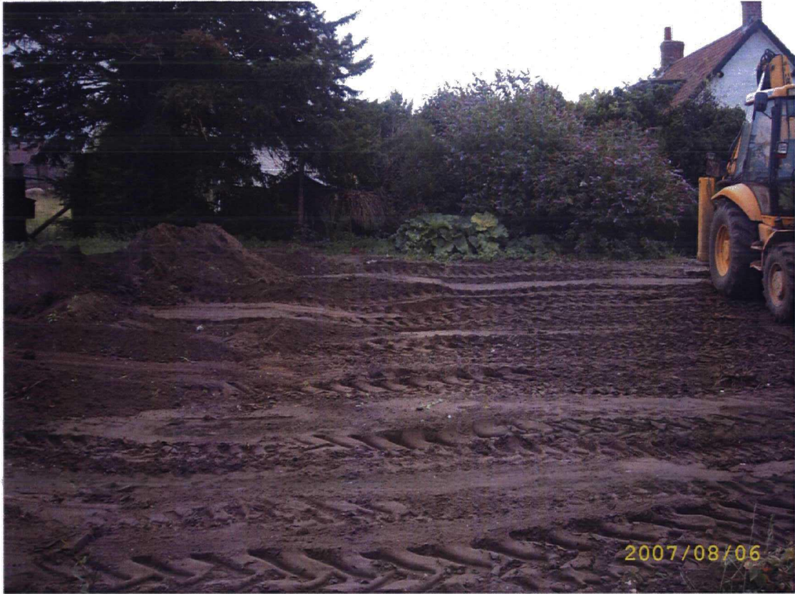
Plate 1 Initial vegetation clearance prior to excavation. Facing East.
