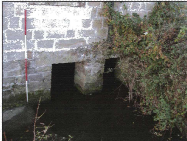
Plate 5 (144: 1/18) exterior, north elevation: view of the culvert, from the north north-east
