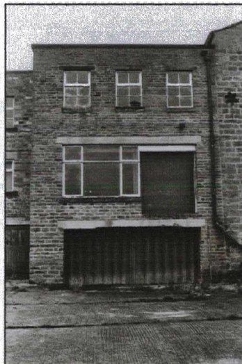
Plate 3 (134:1/31-2) exterior, north elevation: view of the phase 8 extension, from the north
