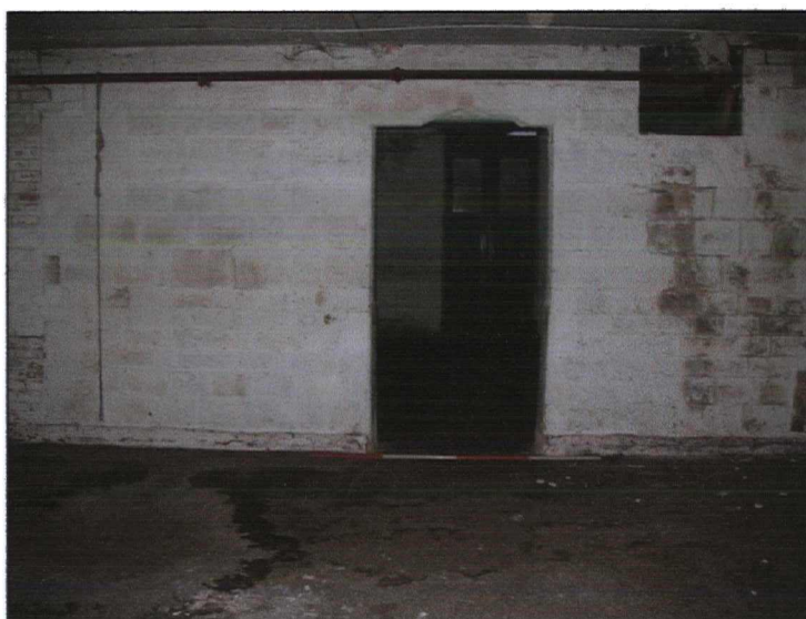
Plate 75 (106: 5/33) Room 2/5: general view, from the west
