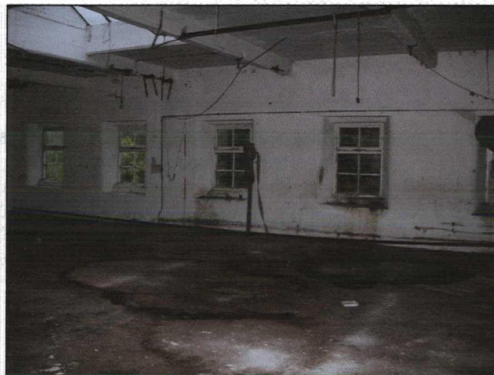
Plate 69 (99: 4/5) Room 2/1: general view, from the north-west
