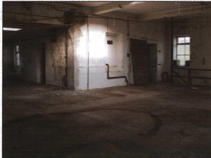
Plate 68 (76: 4/29) Room 2/1: general view, from the south-west
