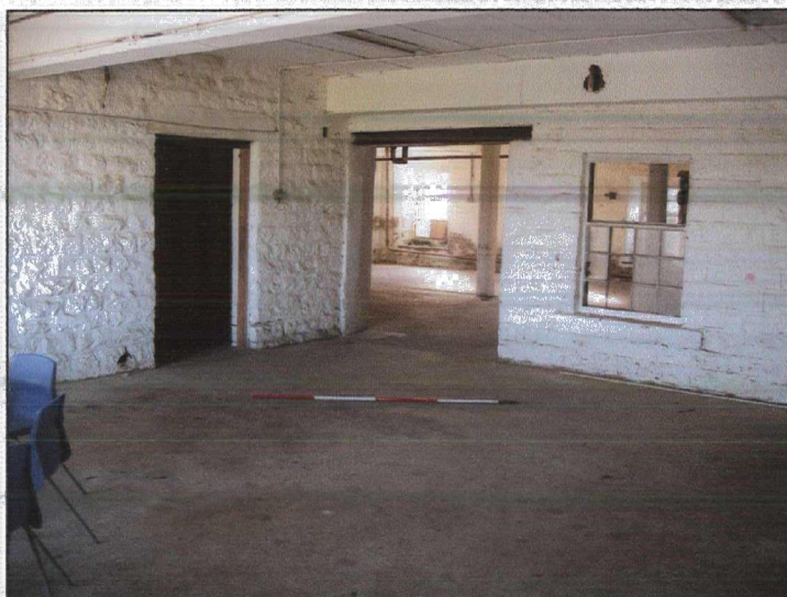
Plate 64 (16: 2/25) Room 1/7: general view, from the north-east
