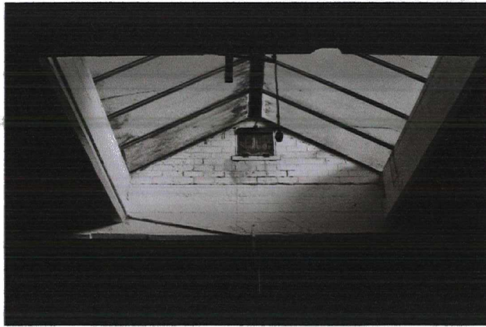
Plate 70 (100: 4/4) Room 2/1: view of the central triangular skylight, from the east
