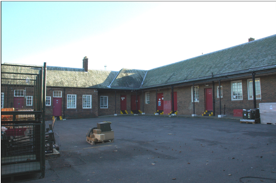
Figure 8 Building 16; courtyard, looking south-east
