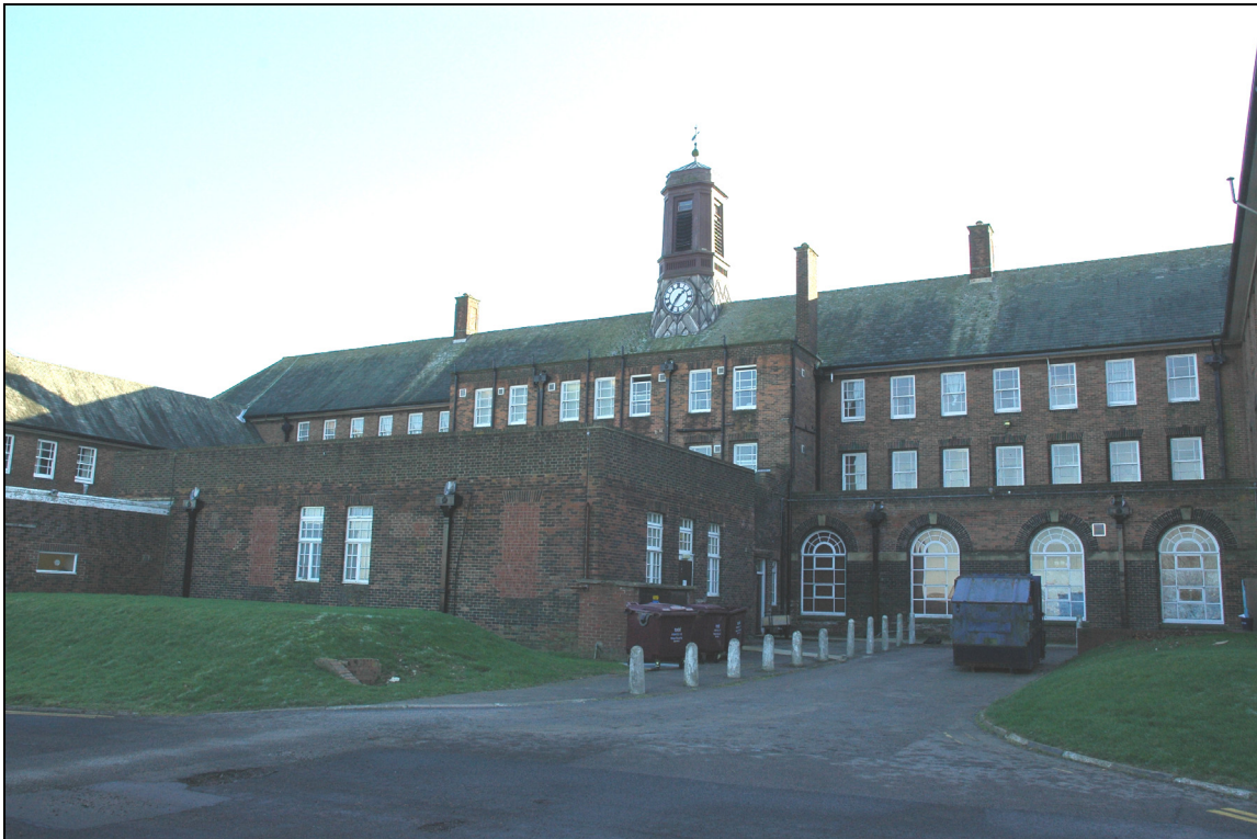
Figure 20 Rear view of the central block of building 22, looking south-east
