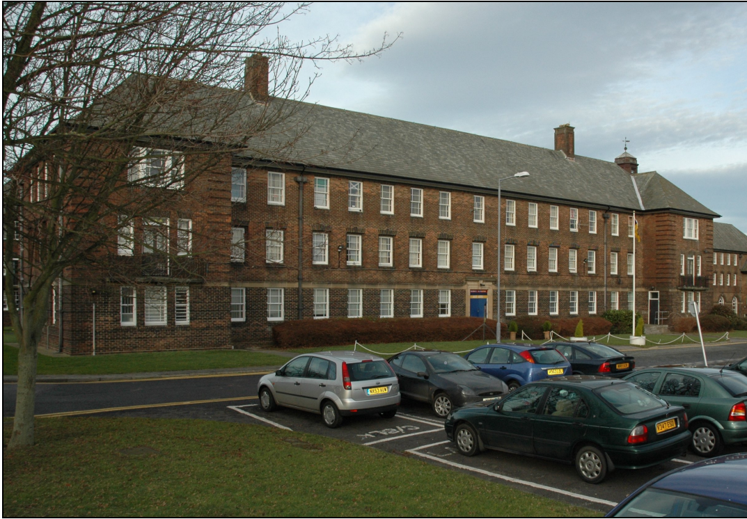
Figure 17 Sandhurst Block, 22. The south-west range, looking north-east
