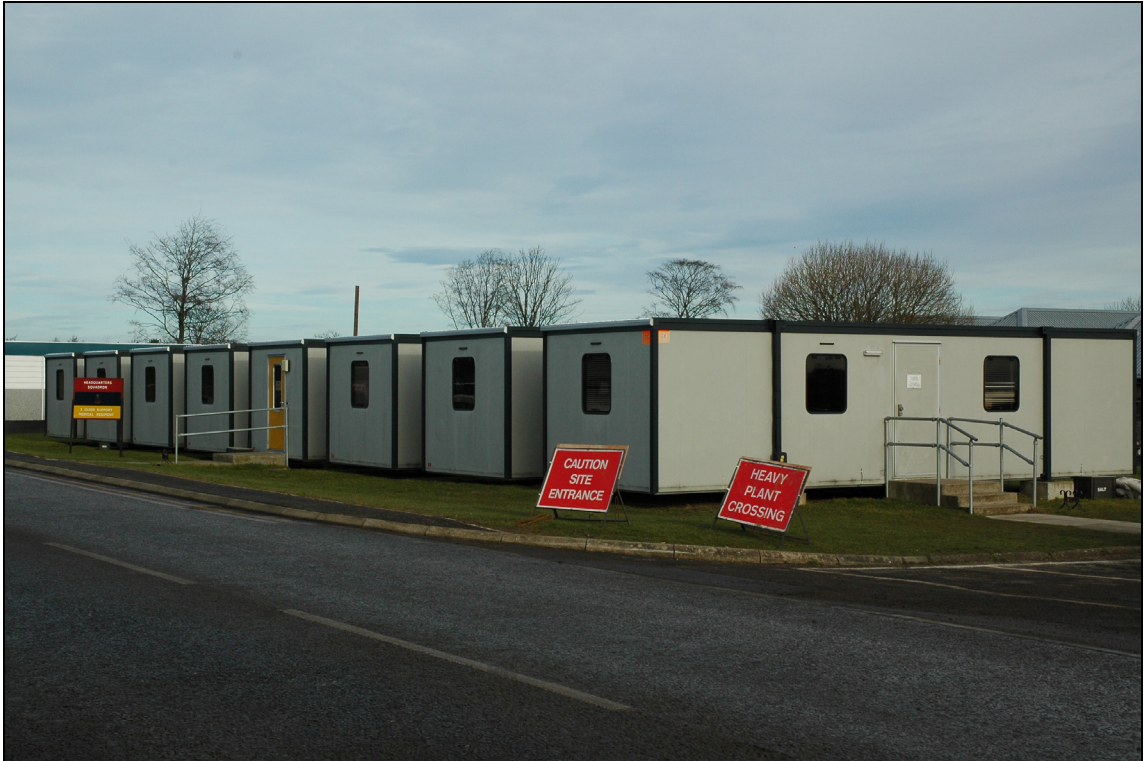
Figure 47 Portakabins, building 38, looking north-east
