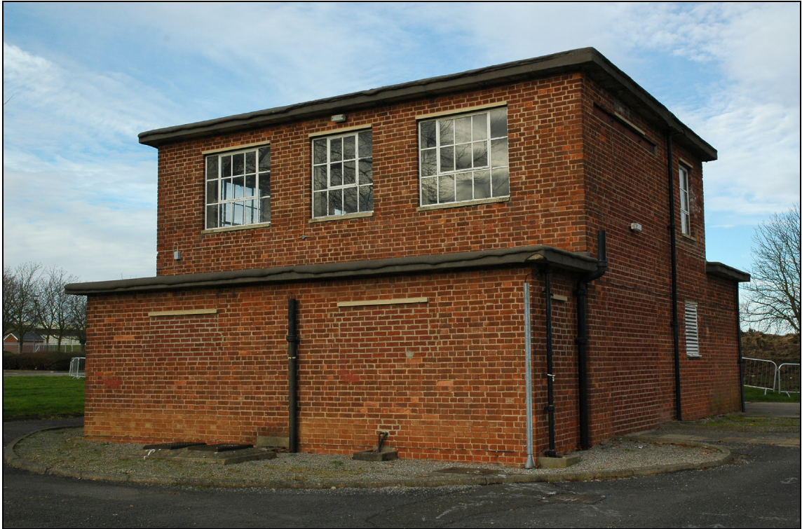
Figure 61 Pump house building 74, looking north-west
