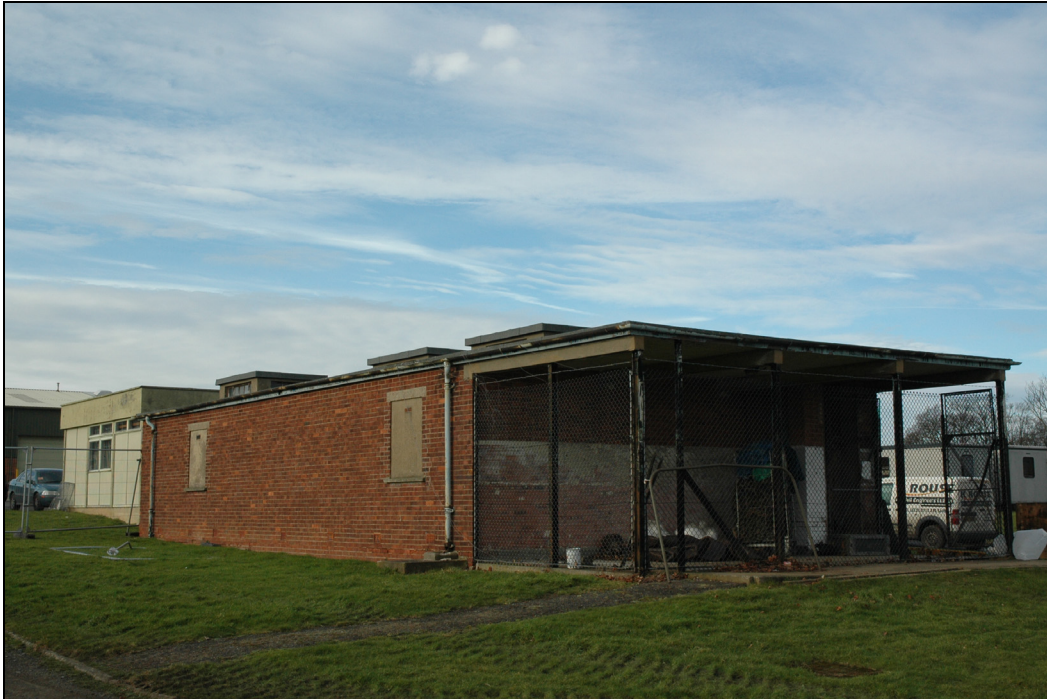
Figure 49 Building 48 looking north-west, showing screened porch used for storage
