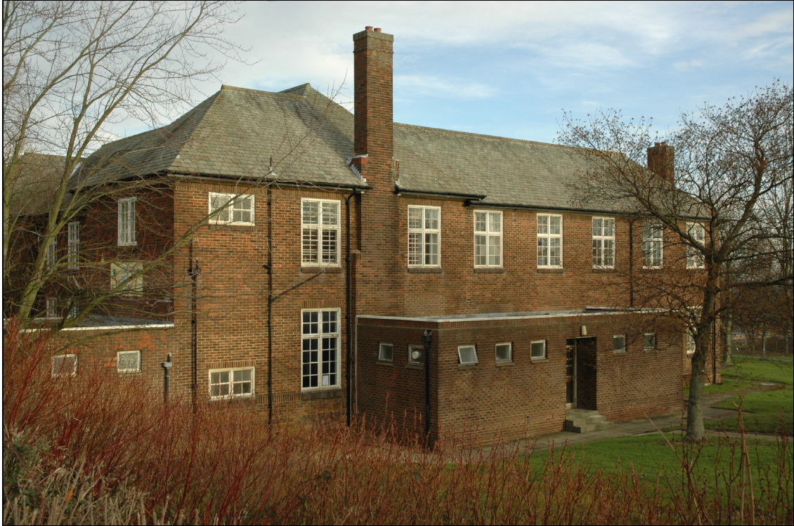
Figure 31 Building 23, the Gaza Club; looking north-east, showing flat-roofed extensions
