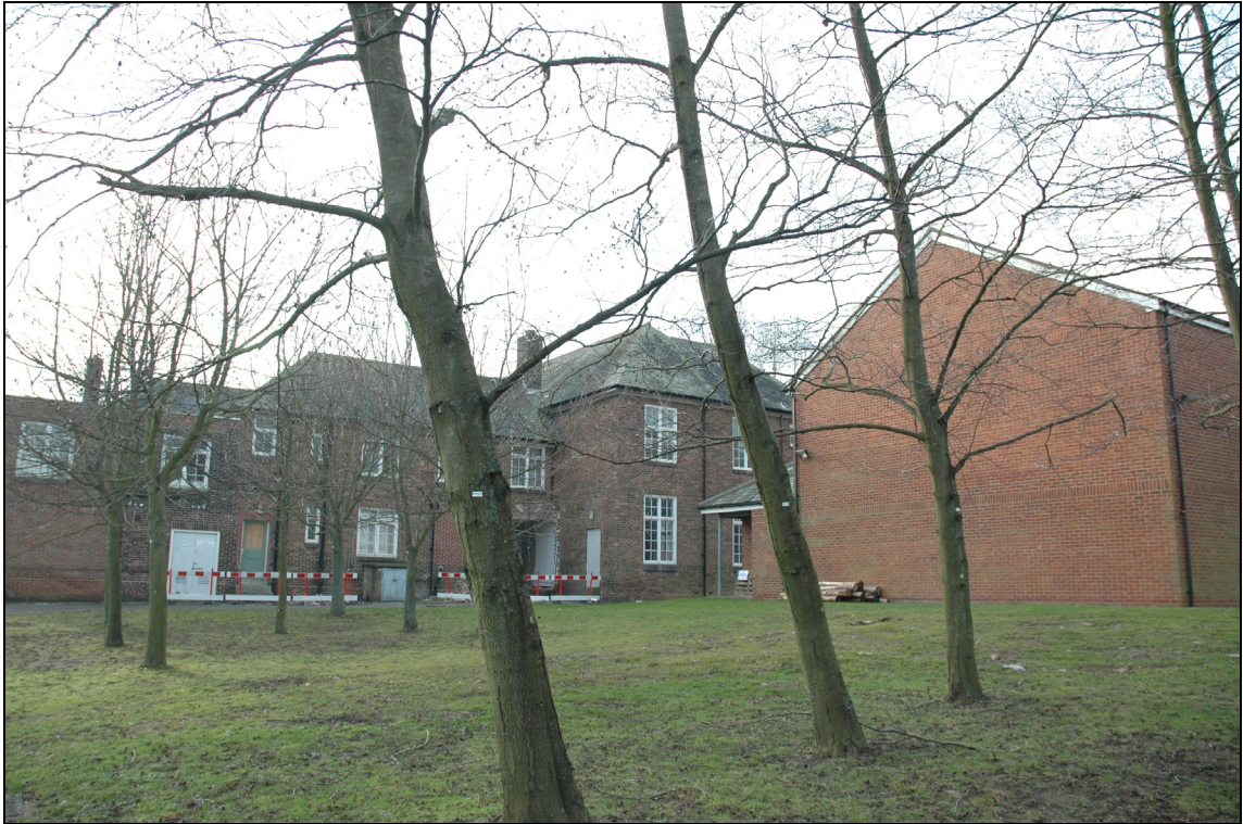
Figure 33 Building 23, the north wall and the rear of Building 104, looking south
