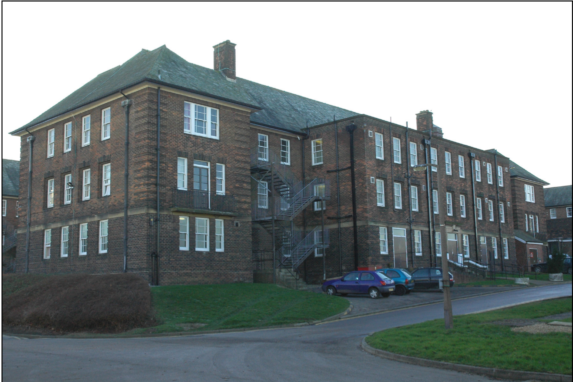
Figure 19 Building 22, looking SW at the rear of the NE range. Note the typical flat-roofed extension
