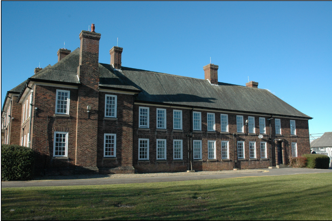
Figure 37 Building 28; the Officers' Mess; the east range, looking north-west
