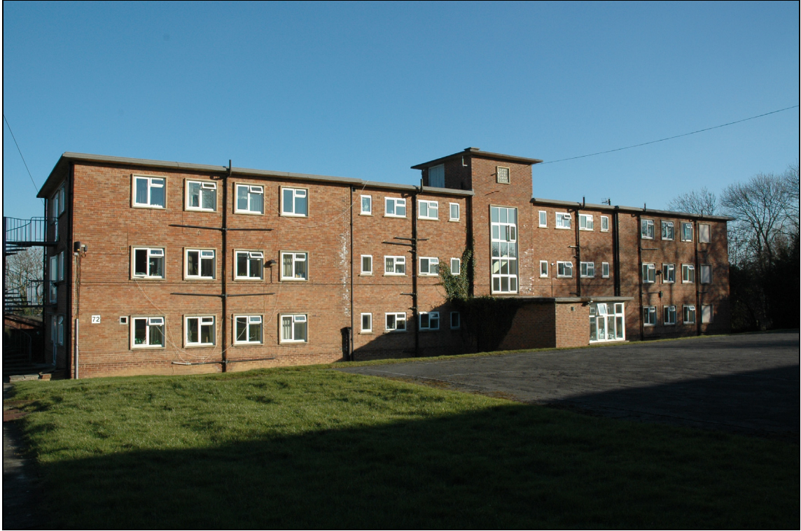
Figure 55 Rear of building 72, looking north-west
