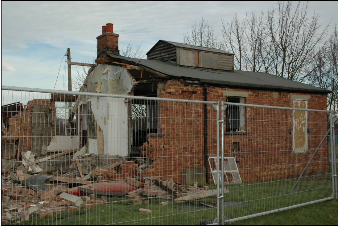
Figure 3 Building 14, during demolition, looking south-west
