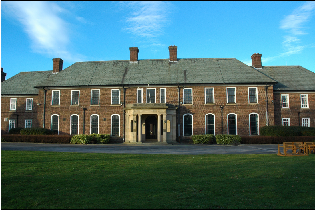
Figure 35 Principal front of building 28; the Officers' Mess, looking north
