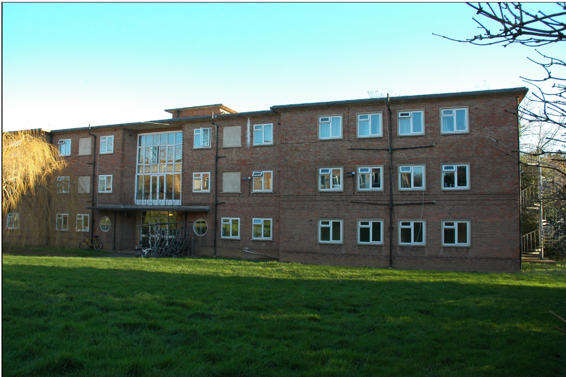
Figure 54 Building 71, looking north-east
