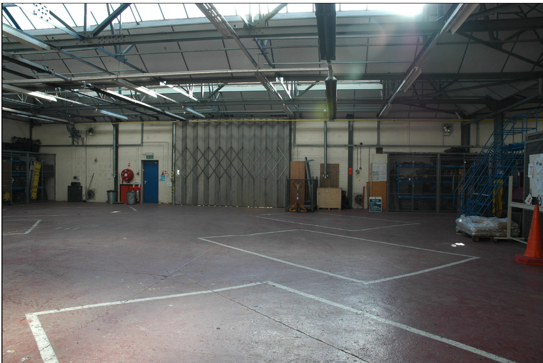
Figure 14 Interior, garage building 17
