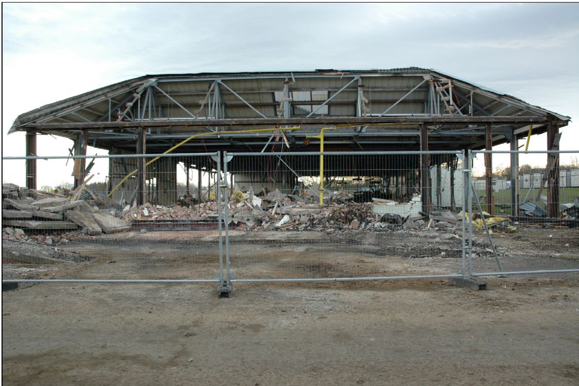
Figure 46 Metal-clad shed, building 37, during demolition. View looking south
