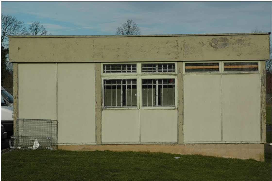
Figure 64 Portakabin M5, looking north
