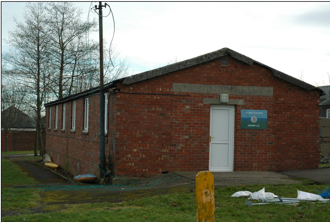
Figure 6 Brick hut, building 15, looking south-west
