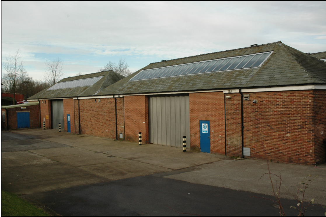
Figure 13 Garage building 17, looking west
