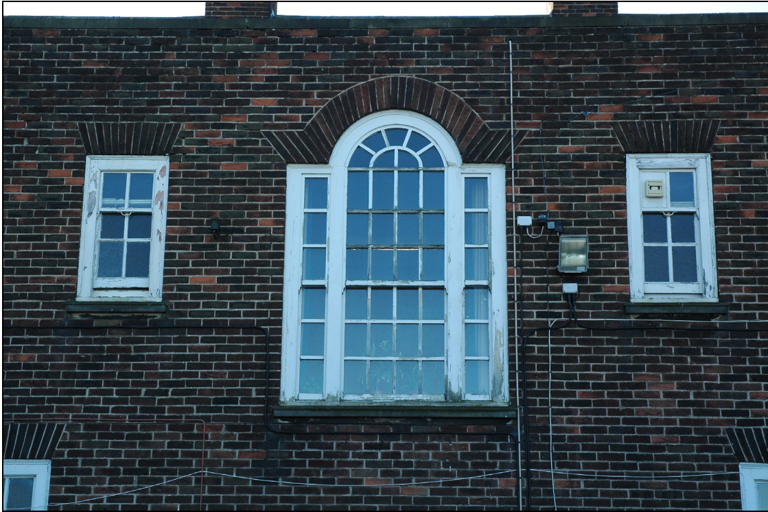
Figure 39 Officers' Mess; Venetian window on staircase
