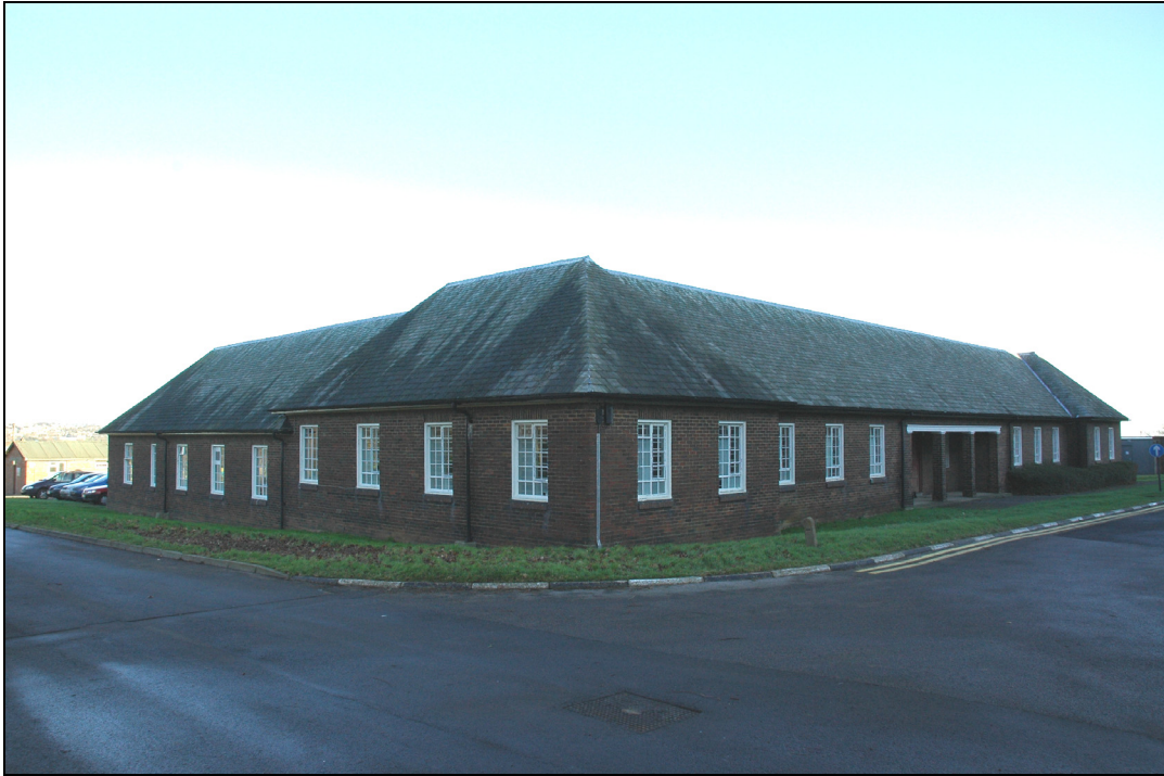
Figure 7 QM Stores, Building 16, looking north-east
