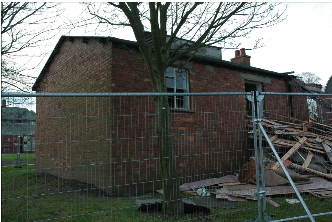
Figure 4 Building 14 during demolition, looking north-east
