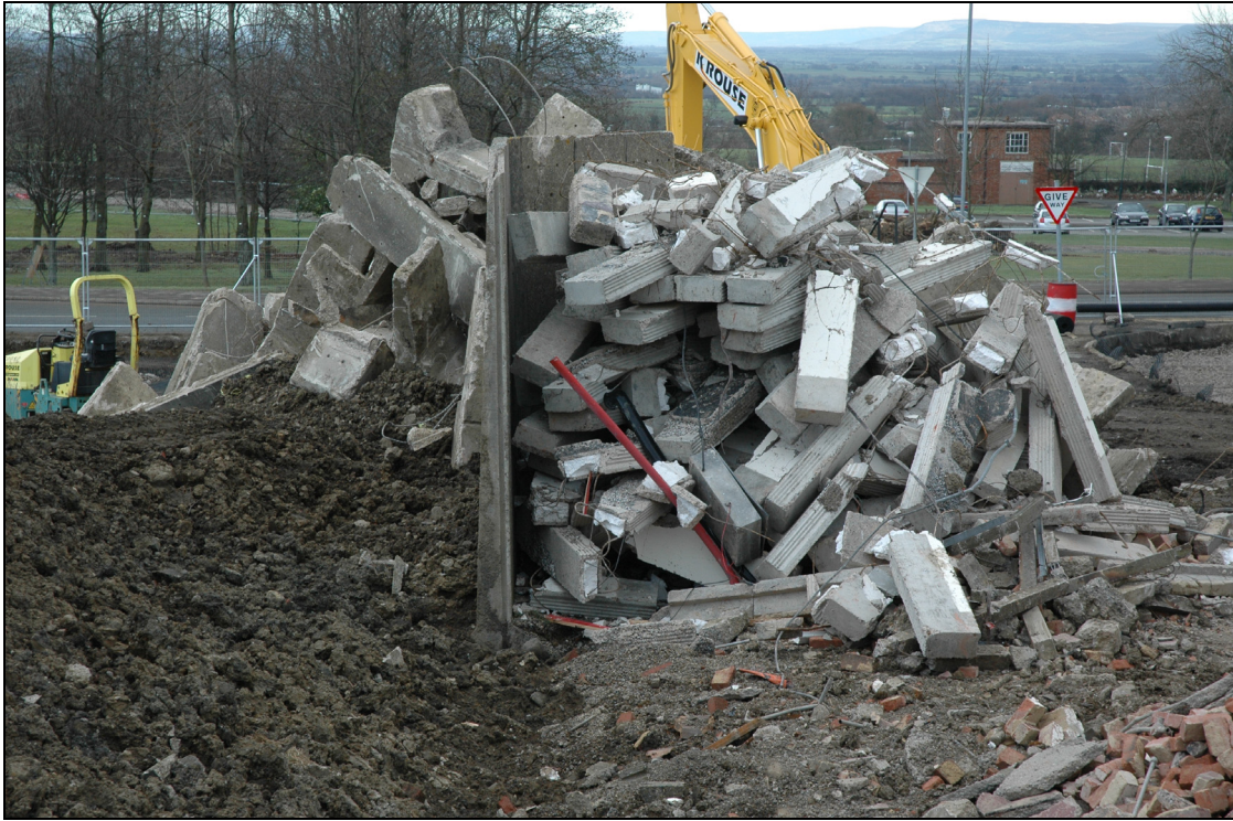
Figure 51 Demolished remains of the ammunition bunker, building 50, looking east
