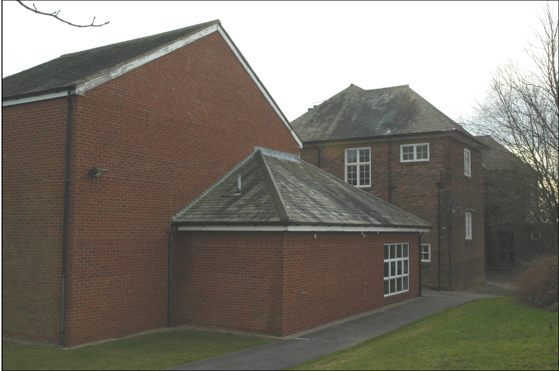
Figure 63 Squash court 104 and NW corner of the Club, building 23, looking south
