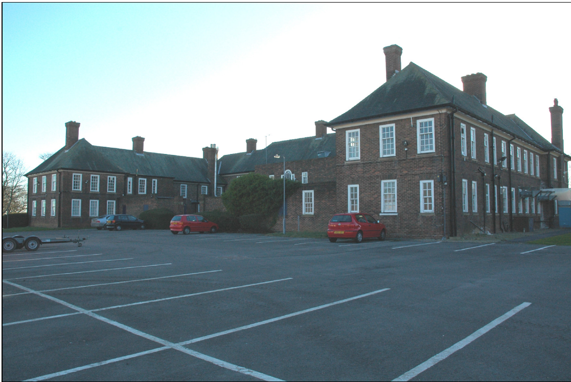
Figure 38 Building 28; the Officers' Mess, looking south-east across the rear courtyard
