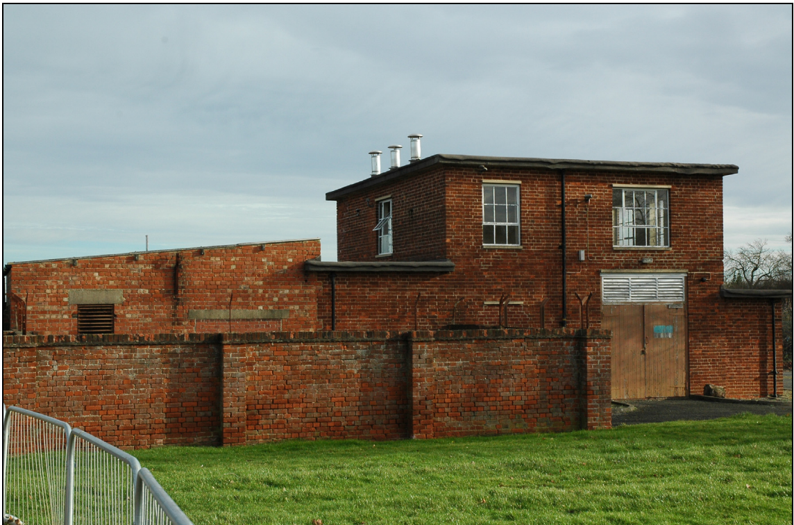
Figure 62 Pump house building 74, looking east
