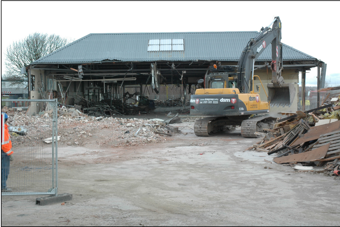
Figure 45 Metal-clad shed, building 37, during demolition. View looking north
