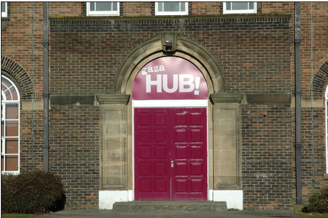
Figure 16 Sandhurst Block, 22; detail of main door
