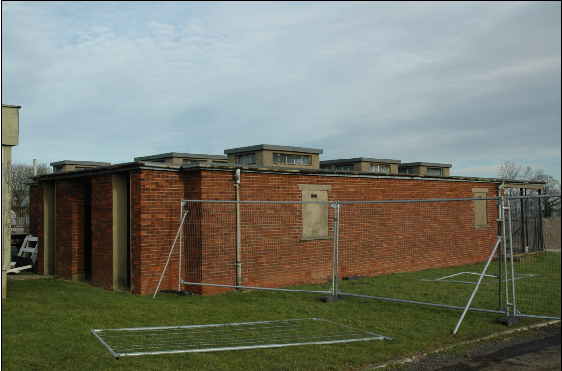
Figure 48 Brick store, building 48, looking north-east. Note the clearstorey windows
