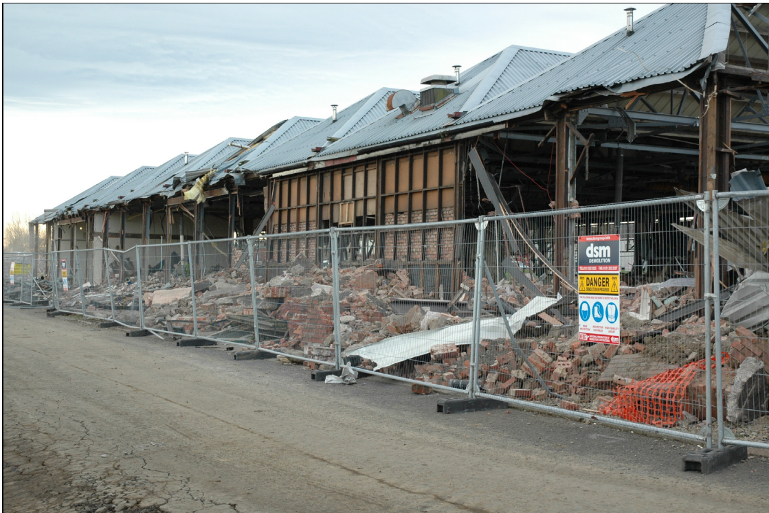
Figure 44 Metal-clad shed, building 37, during demolition. View looking south-west
