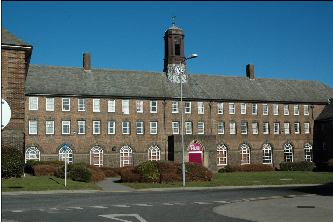
Figure 15 Sandhurst Block, 22, looking north at the central range
