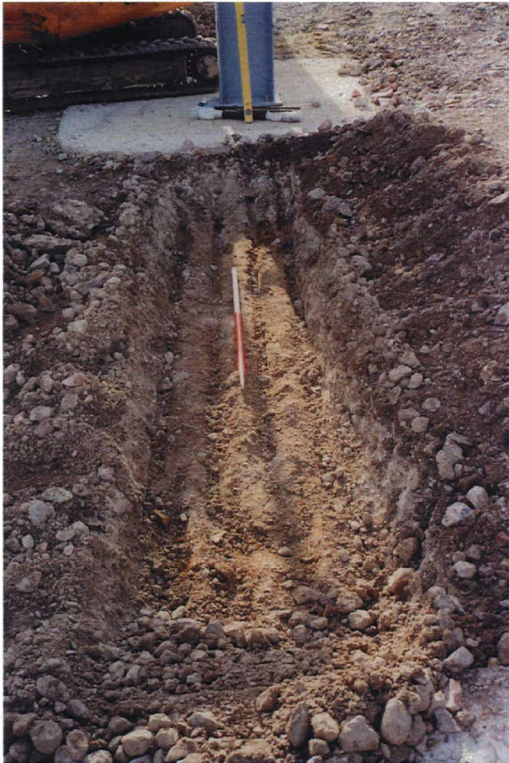
Plate 3. View of Foundation Trenches. Facing North
