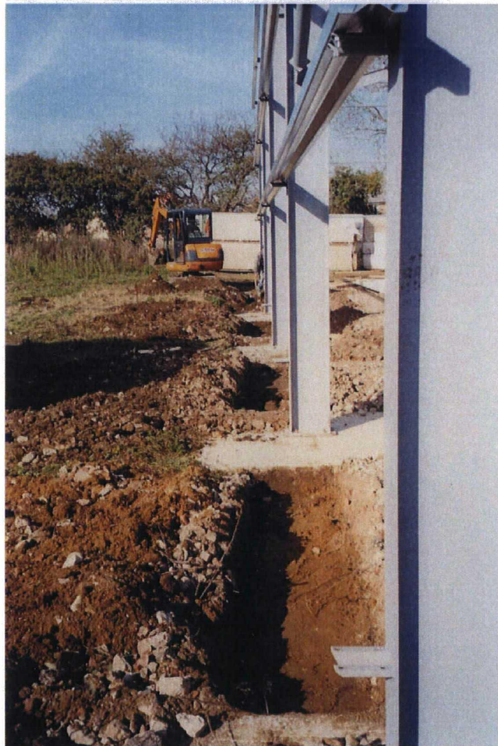
Plate 2. View of Foundation Trenches. Facing North
