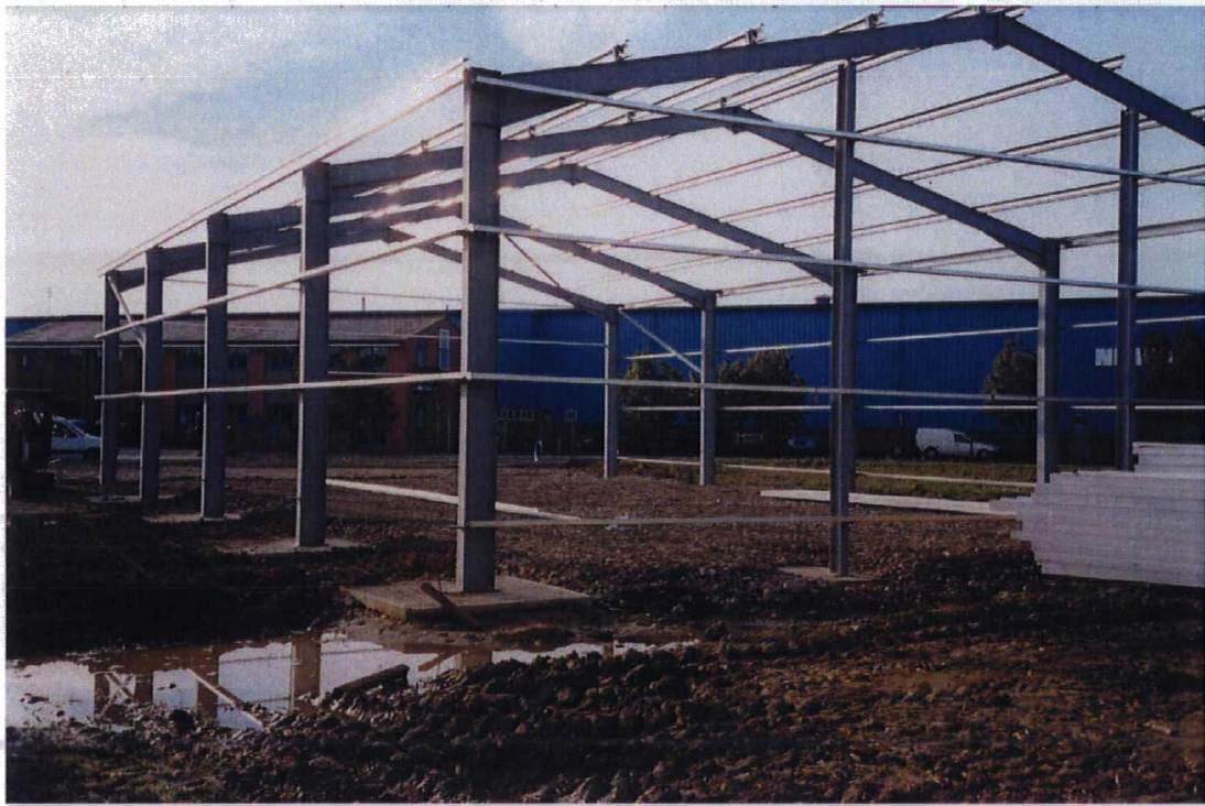
Plate 1. General View of Site. Facing South West
