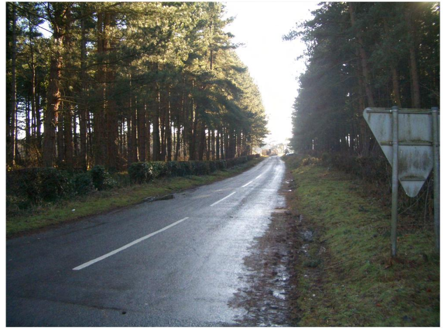
Plate 4. Wintringham Road. Facing South-west.
