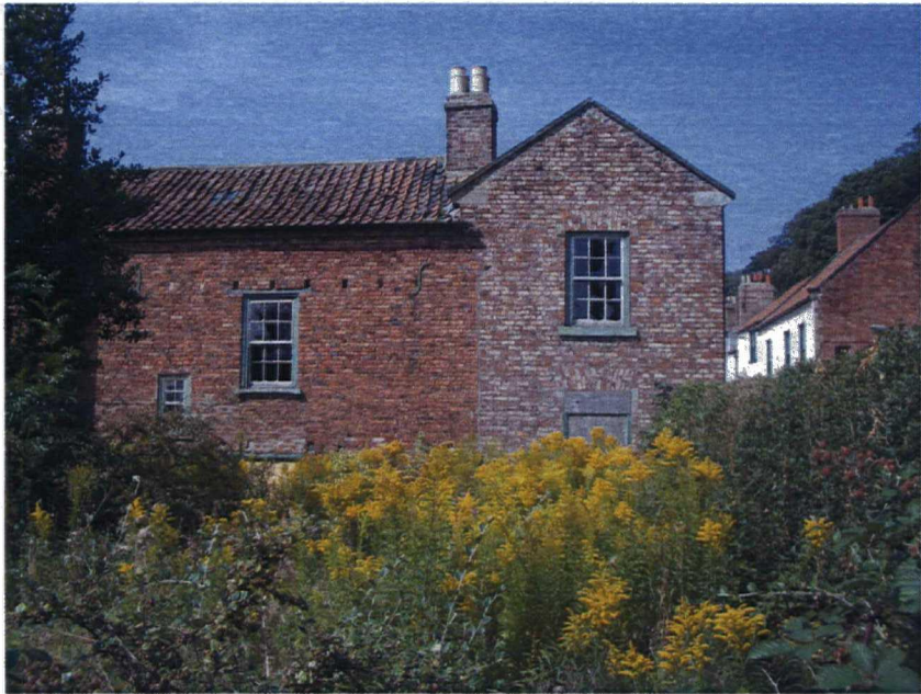
Plate 13. Site 5. 104 Sheepfoot Hill. Facing West.
