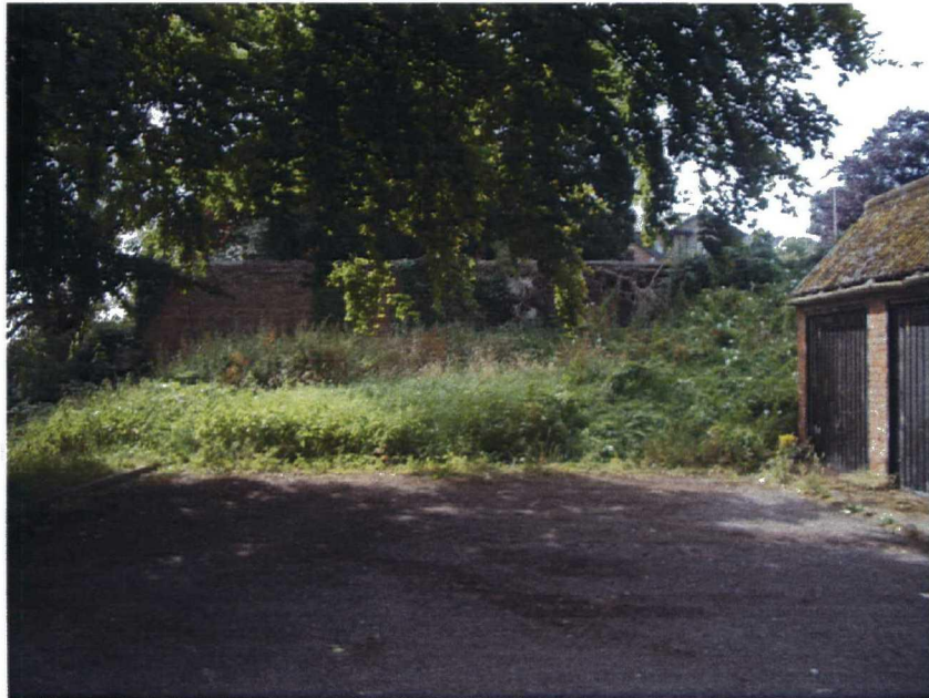
Plate 9. Site 2. Garden Wall. Facing West.
