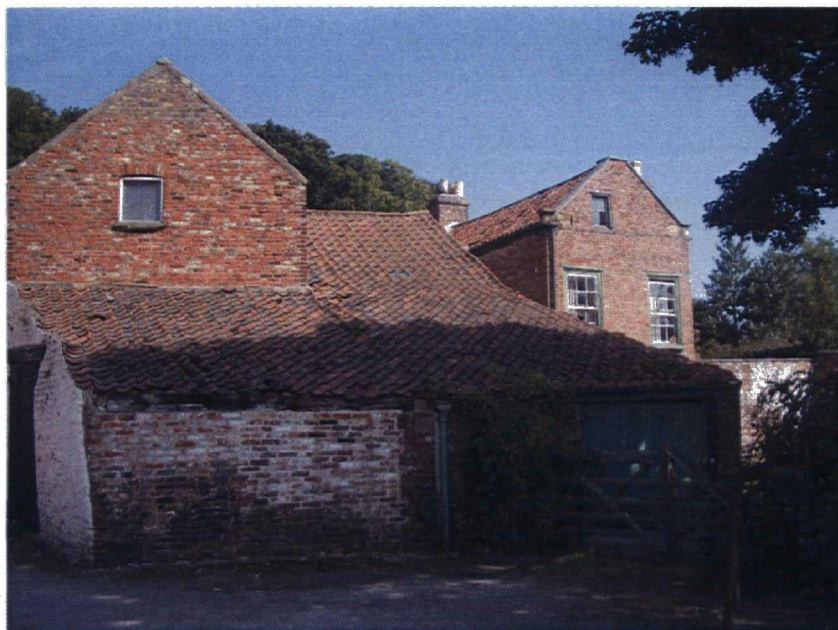
Plate 11. Site 5. Rear of Warehouse. Facing North-east .
