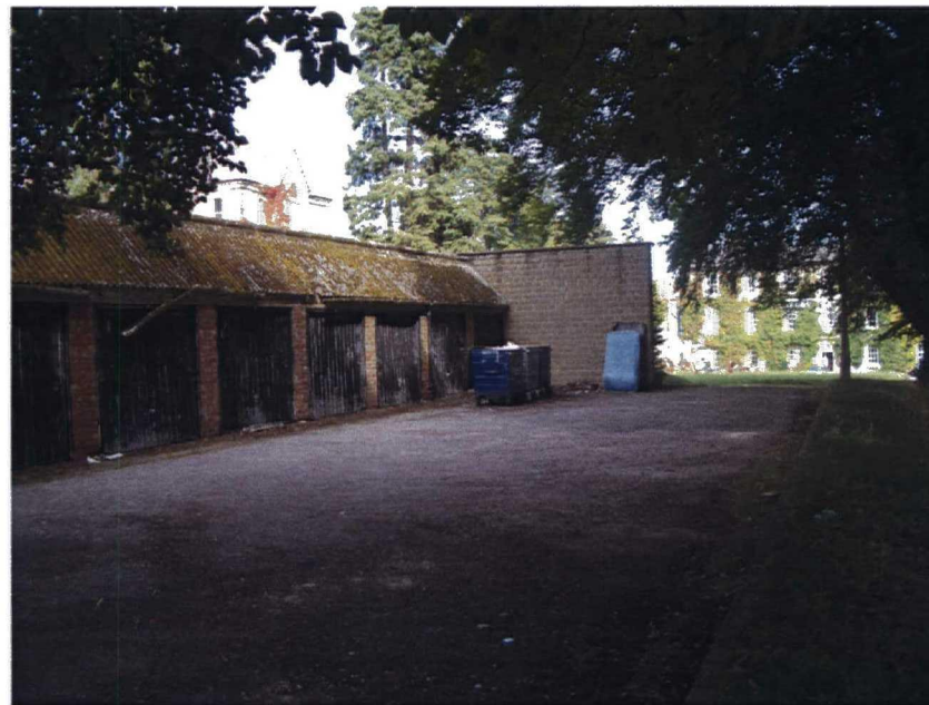
Plate 6. Site 2. Garages. Facing East.
