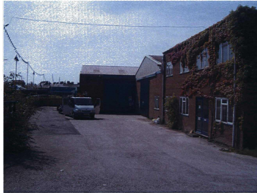
Plate 20. Site 6. General View of Riverside Works. Facing South.
