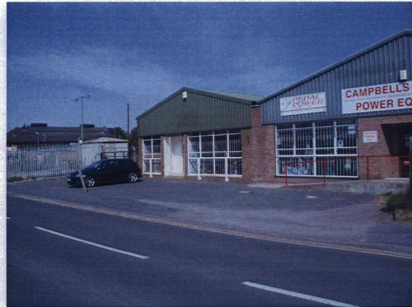
Plate 40. Site 25. General View of Retail Units. Facing North-west.
