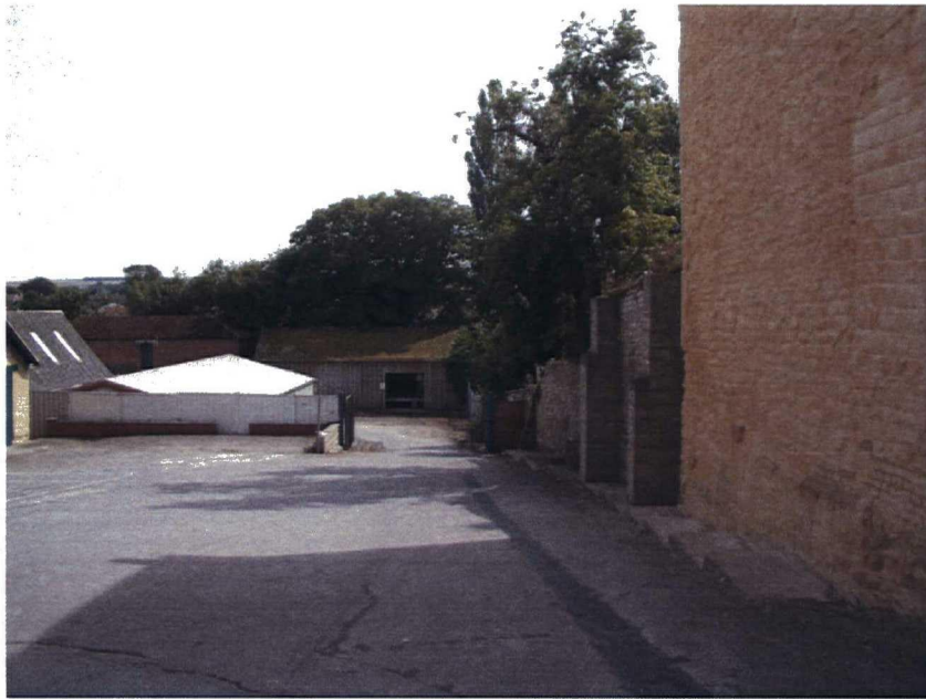
Plate 1. Site 1. General View from Yorkersgate. Facing South.
