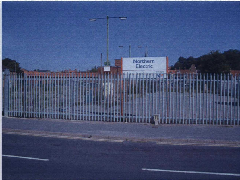
Plate 39. Site 25. General View of Depot. Facing North.
