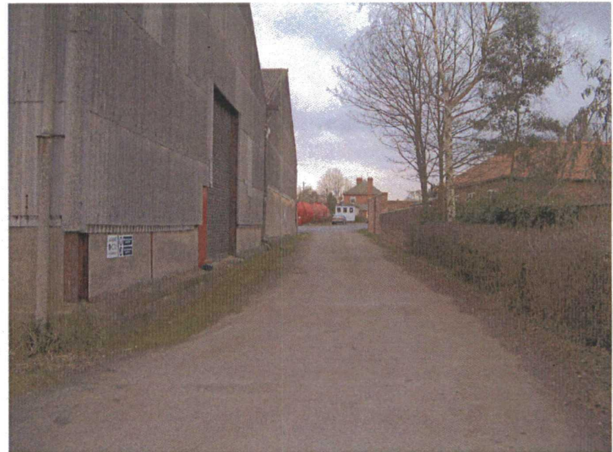
Plate 10. General View of Site. Facing South.
