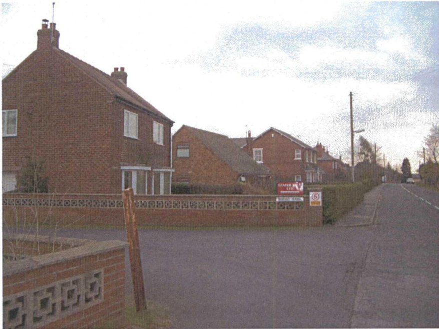
Plate 1. Entrance to the Site from Station Road. Facing East.
