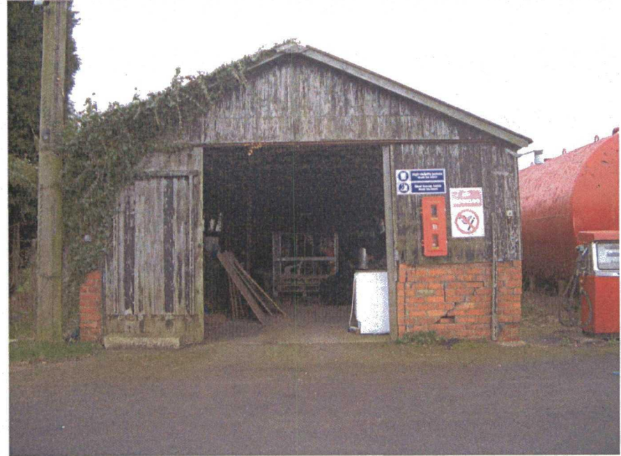
Plate 14. Brick and Timber Garage. Facing East.
