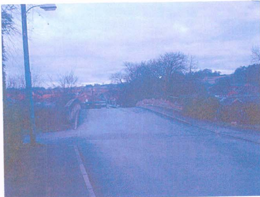
Plate 7. View of Railway Bridge on Ings Lane. Facing North
