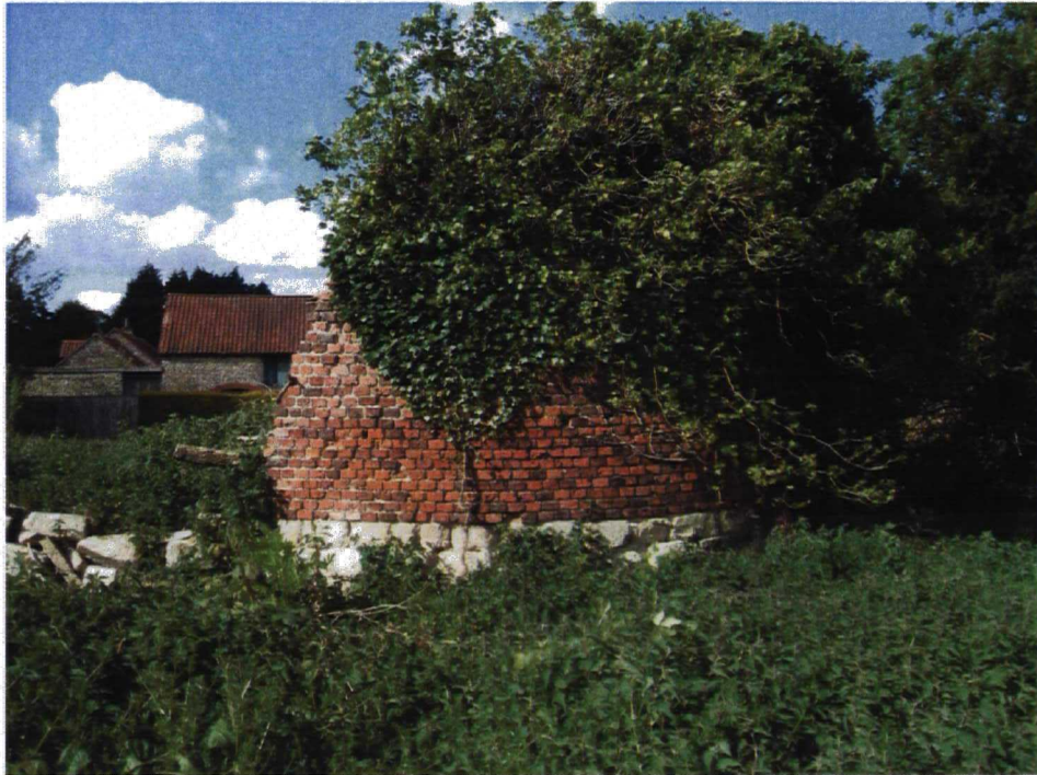
Plate 1, stone and brick walling of boundary (B), looking north
