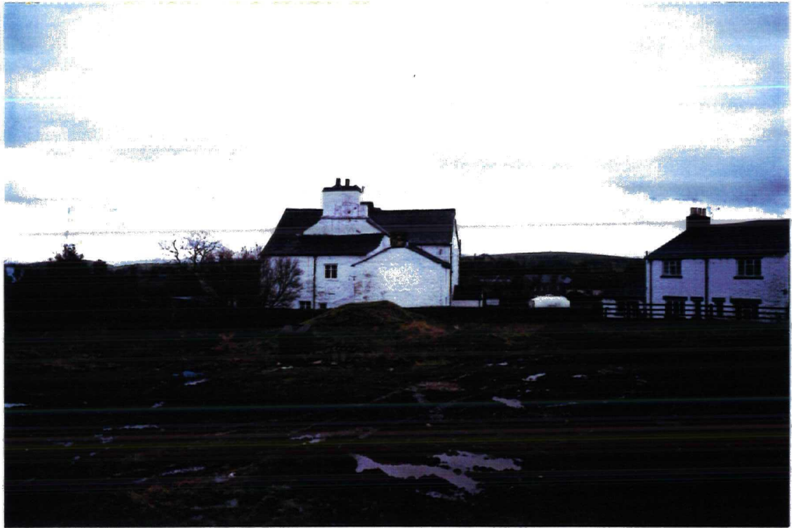
Plate 3. General view of Old Hall. Facing south.
