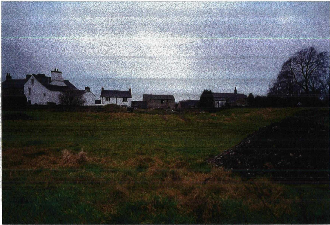
Plate 1. General view of site. Facing west.
