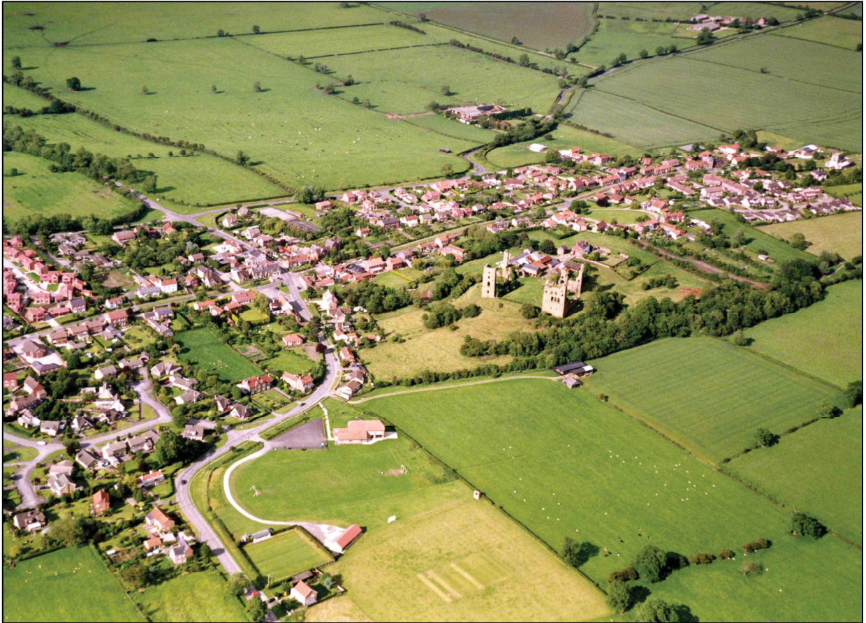
Plate 1: Aerial view of Sheriff Hutton Castle and village, taken June 1991 (Aeroscene Ltd, AJC 260/22).
