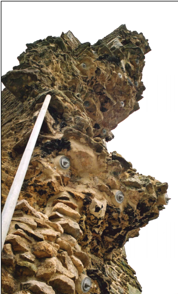
Plate 46: Structural ties inserted to support overhanging masonry.
