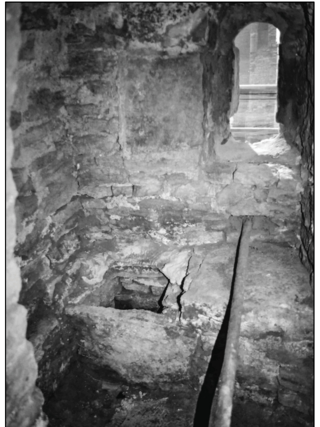
Plate 24: Third floor garderobe seat (L2/3), chute (C2/2) and window (W2/8) with tie bar.
