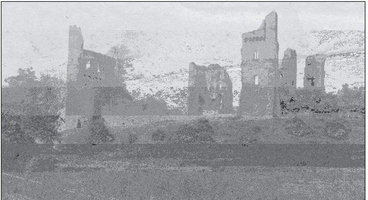
Plate 12: Photograph taken between 1875 and 1887, showing collapse of the NE tower (Tony Wright collection) (NE tower on extreme right).
