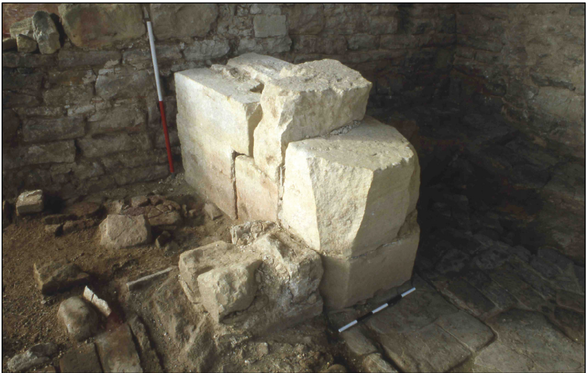
Plate 33: Excavation Area D - detail of ashlar wall (context 005), showing burning on south side.
