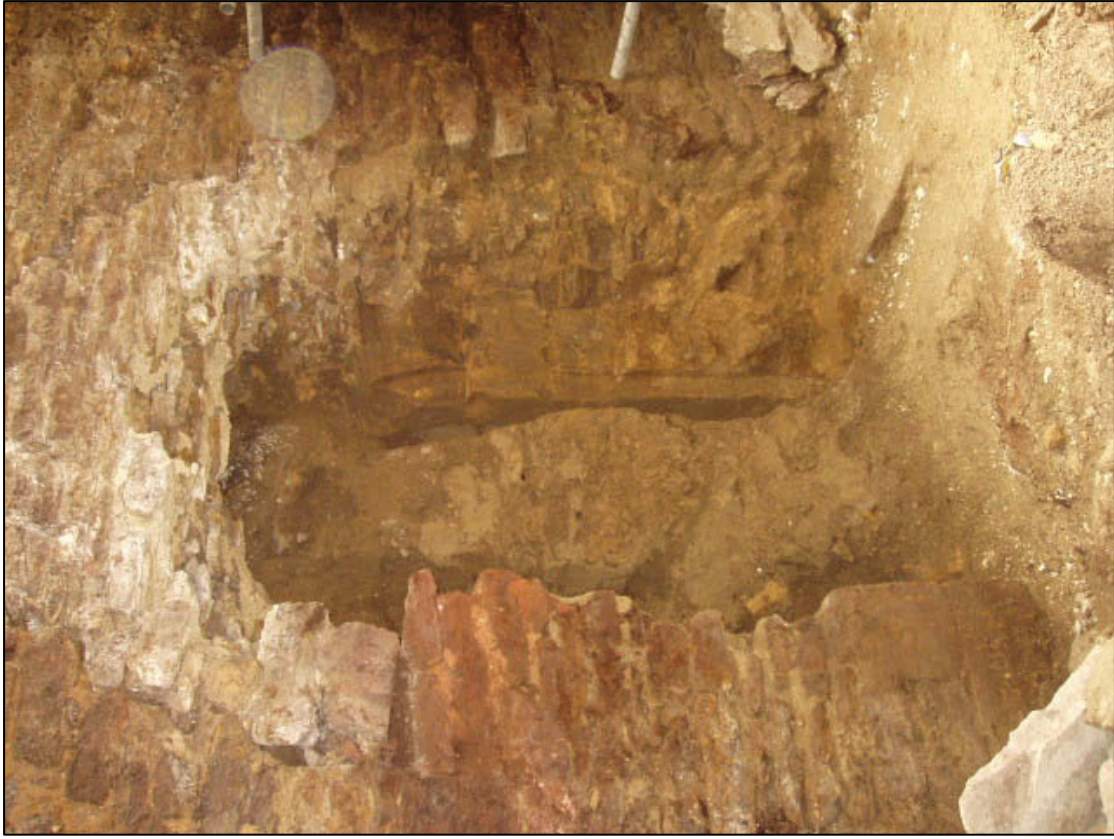
Plate 19: Newly exposed door opening (D2/3) in south wall of basement, prior to consolidation.
