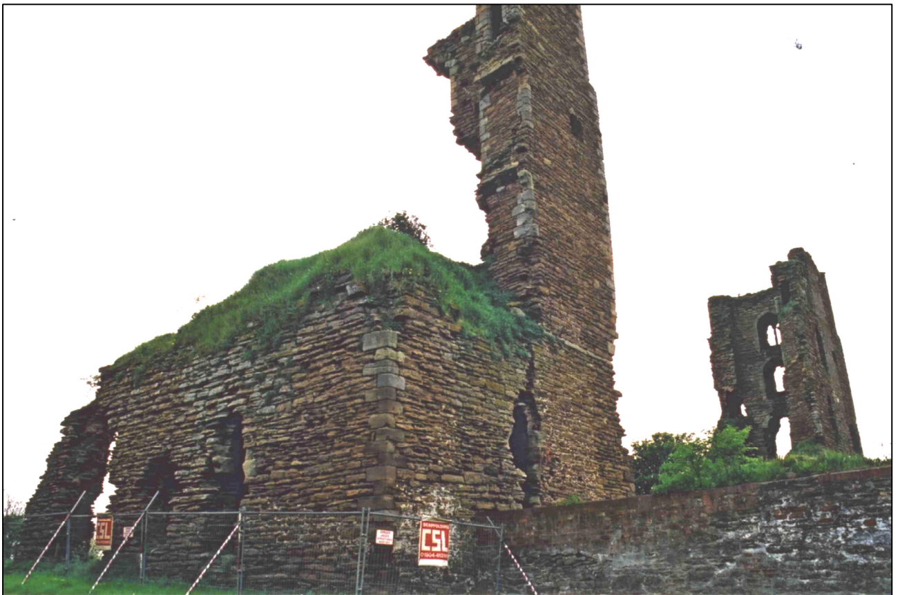
Plate 4: North-east tower, looking SW, prior to repair and consolidation (September 2001).
