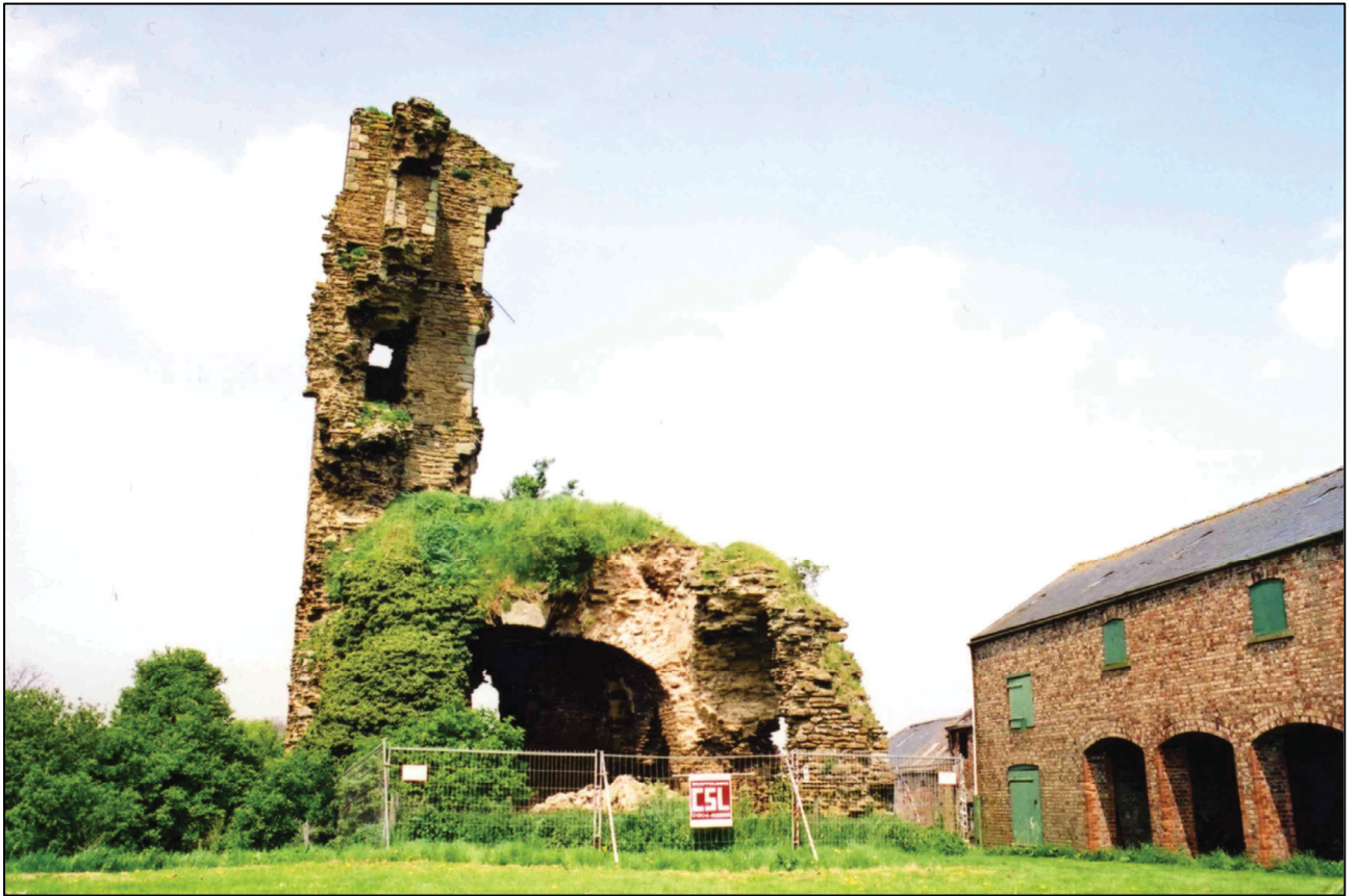
Plate 3: North-east tower, looking N, prior to repair and consolidation (September 2001).
