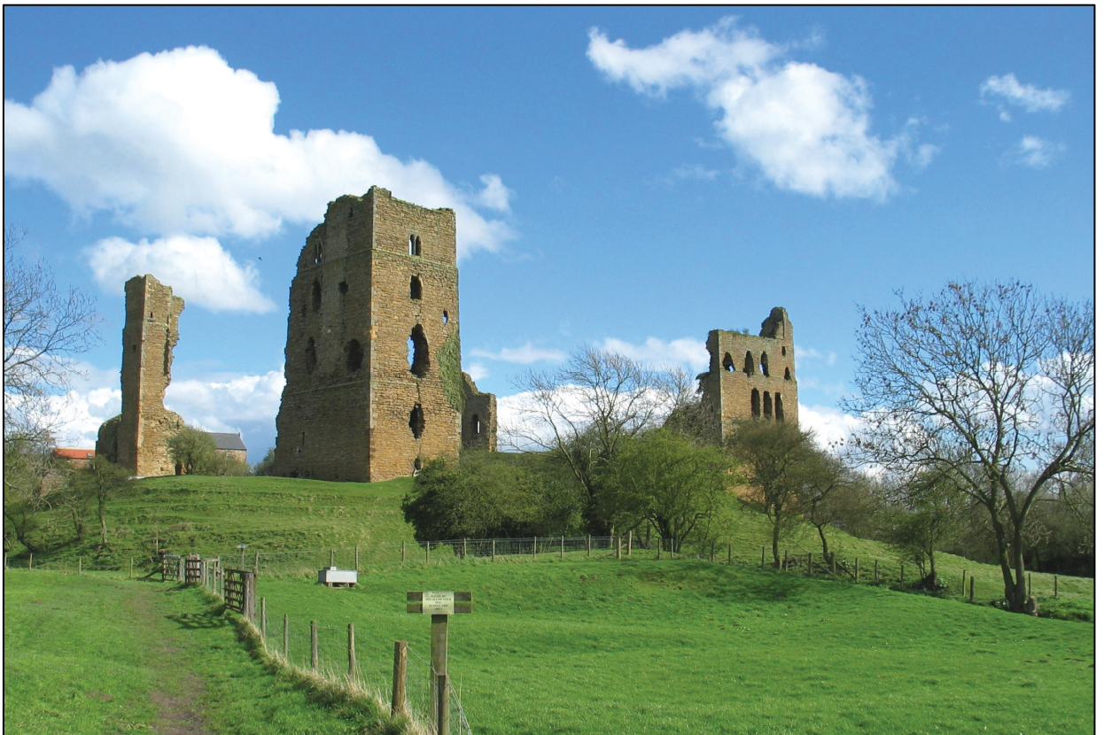
Plate 2: Sheriff Hutton Castle, looking SE (NE tower on left).
