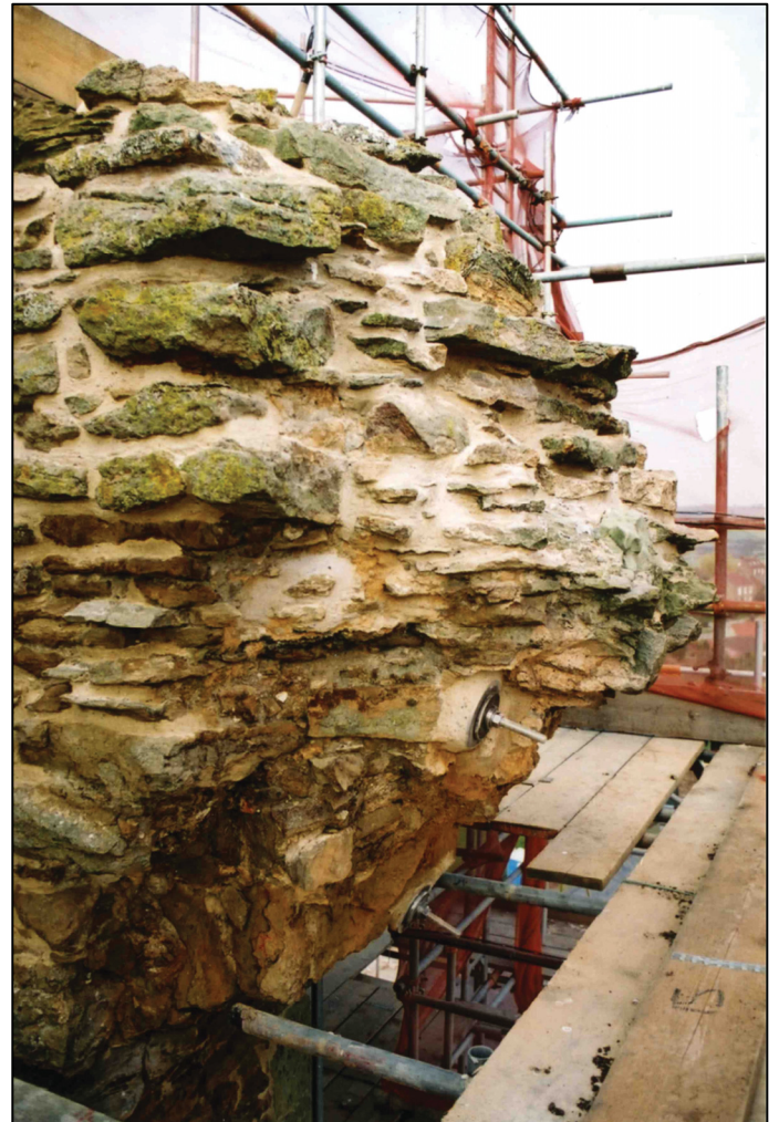
Plate 47: Detailed view of structural ties.
