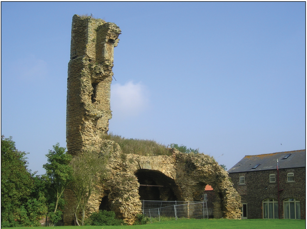
Plate 51: Consolidation and repair work complete.
