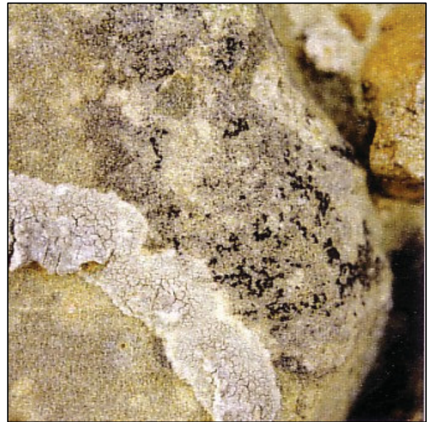
Plate 41: Detail of lichen Haematomma ochroleucum (left) and Verrucaria muralis (right) on a quoin on the north elevation.
