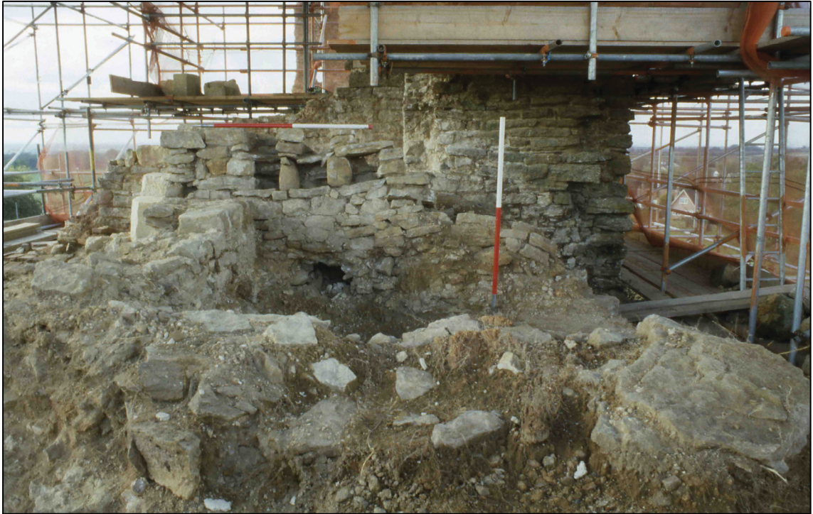
Plate 30: Excavation Area D - rubble wall (context 006) showing nesting boxes, looking W.
