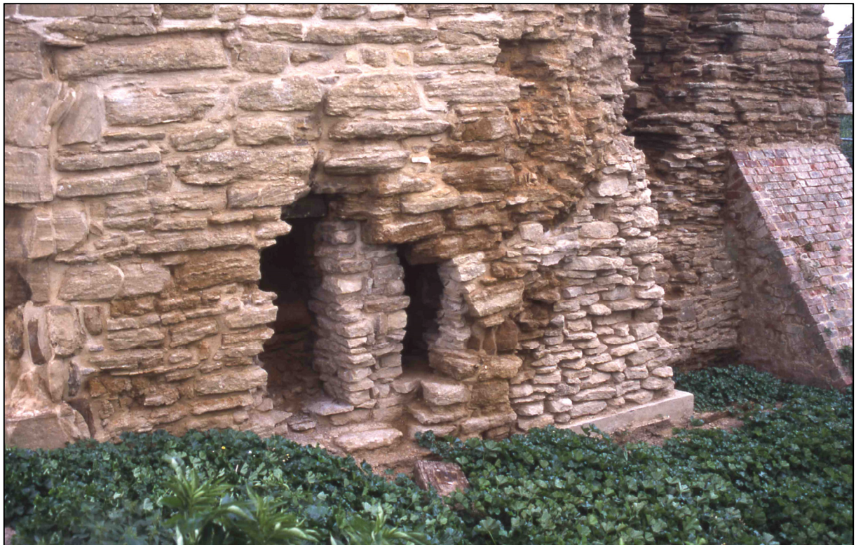
Plate 18: Garderobe chutes (C2/2 & C2/3) in west external elevation, after selective rebuilding and consolidation.
