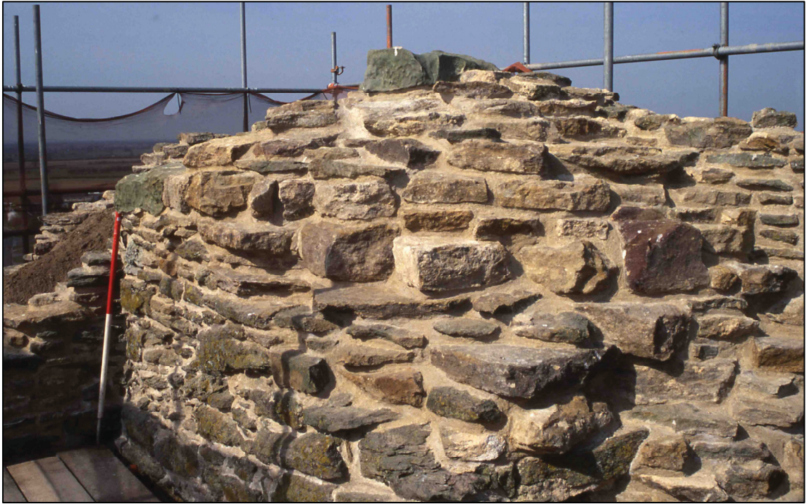
Plate 45: Rebuilt and reset stonework at the top of the north-east tower (compare with plate 37).
