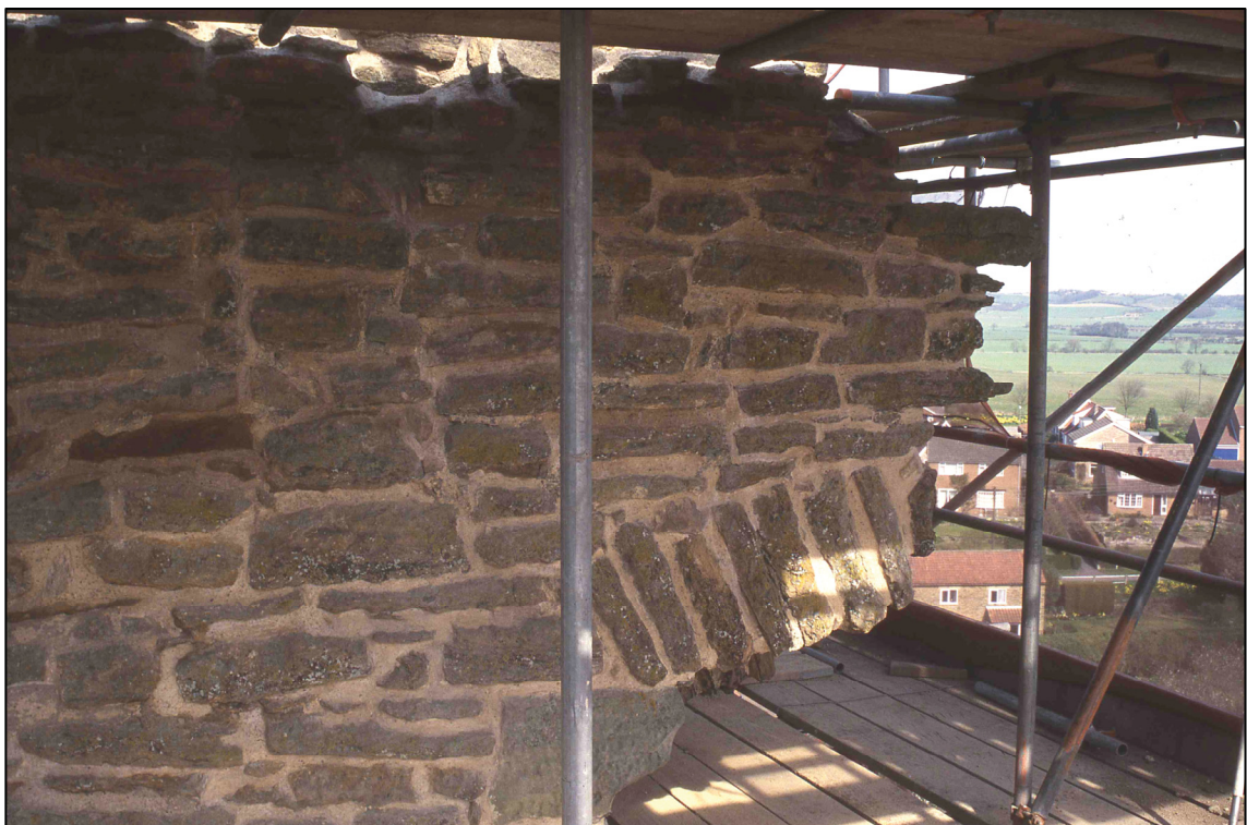
Plate 44: Area of repointed masonry, third floor, north internal elevation.
