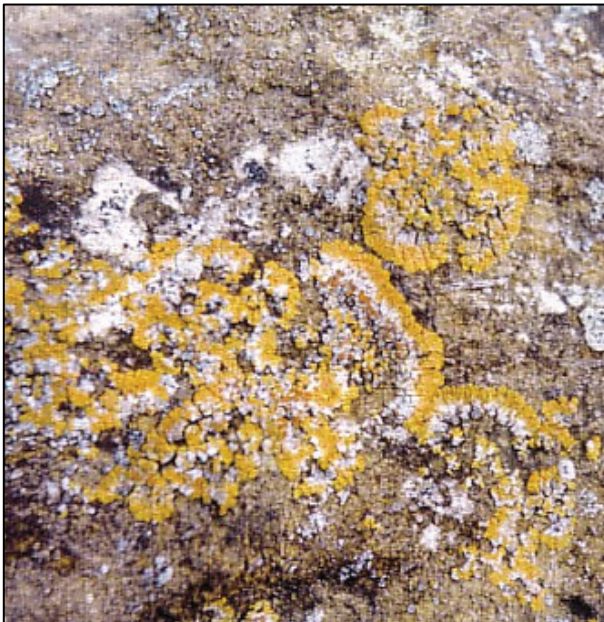
Plate 40: Detail of lichen Caloplaca flavescens with Lecanora dispersa on the north elevation.
