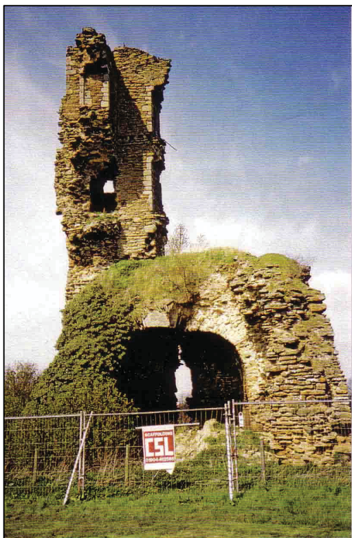
Figure 1 Sheriff Hutton Castle: north-east tower viewed from the south
