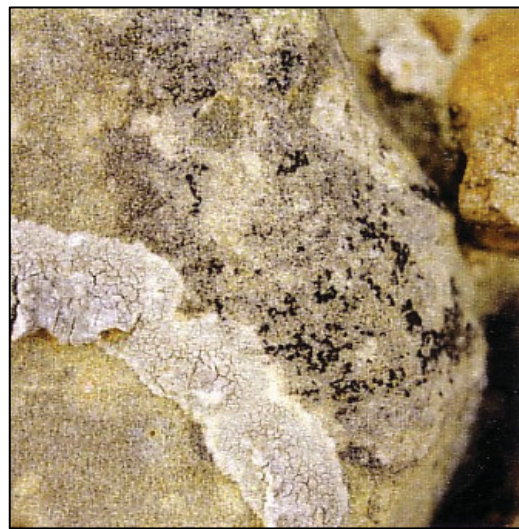
Figure 8 detailed appearance of Haematomma ochroleucum (left) and Verrucaria muralis (right) on a quoin stone on the north elevation
