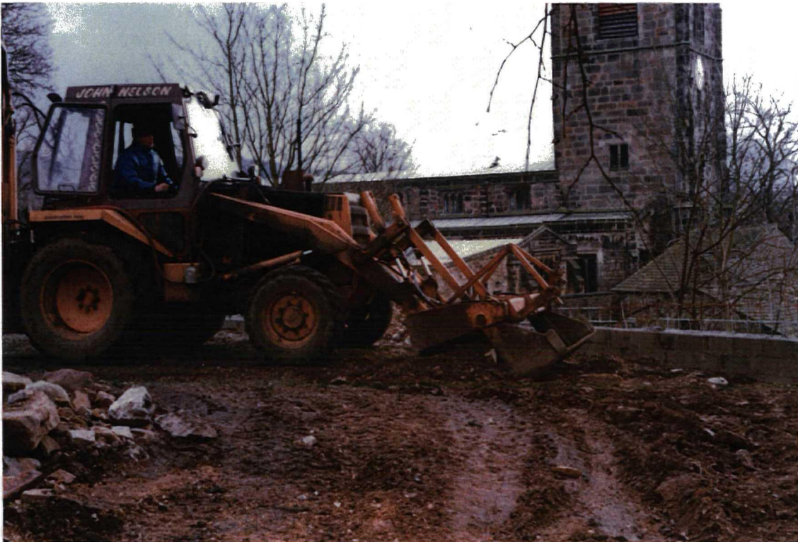
PLATE 4 ST. JOHN'S TERRACE, GROUND LEVELLING
