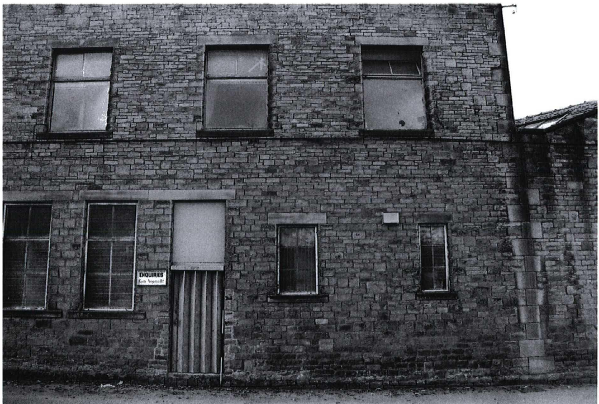
Photograph 6 9984/17 NE Buildings join at quoined corners with windows to two floors
