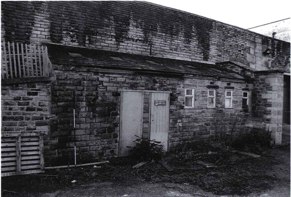
Photograph 21 9984/5 NE Single-storey lean-to store and toilet block
