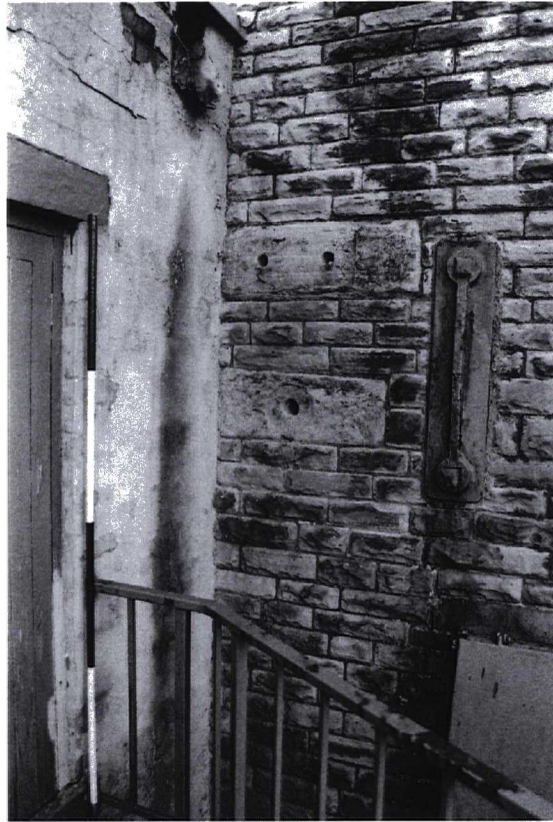
Photograph 12 9984/23 N Cast-iron plates and evidence of previous wall fixings
