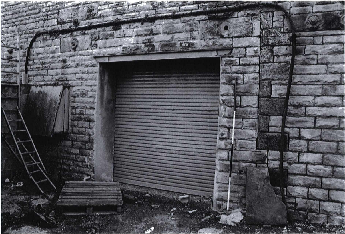
Photograph 17 9983/8 NW Modern roller-shutter door
