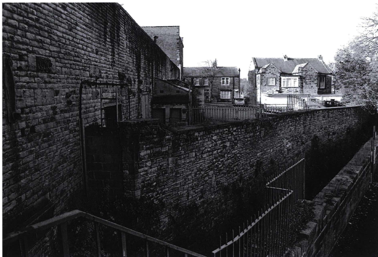
Photograph 14 9984/22 E Culverted watercourse
