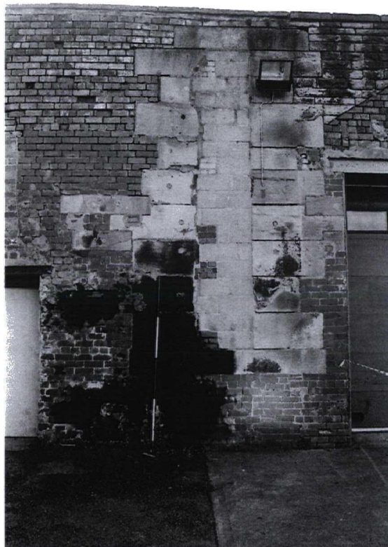
Photograph 22 9984/1 N Straight joint with ashlar quoins. Also, some later brick blocking
