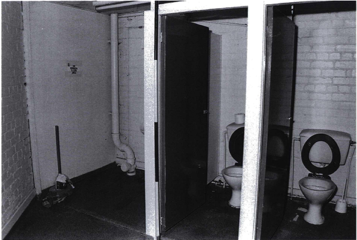
Photograph 30 9983/33 S Toilet area showing partitioned cubicles; all walls are of brick
