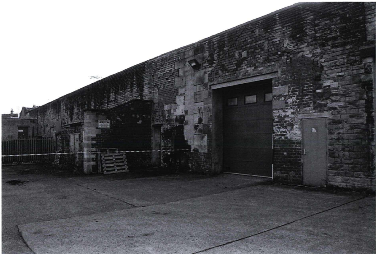
Photograph 24 9984/3 NW Oblique view across the face of the building
