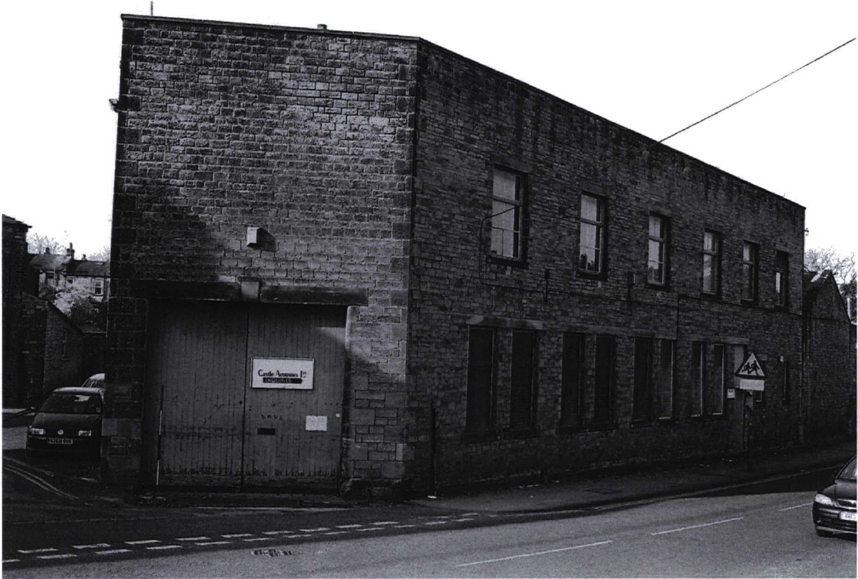
Photograph 7 9984/14 E Large loading doors in the corner elevation
