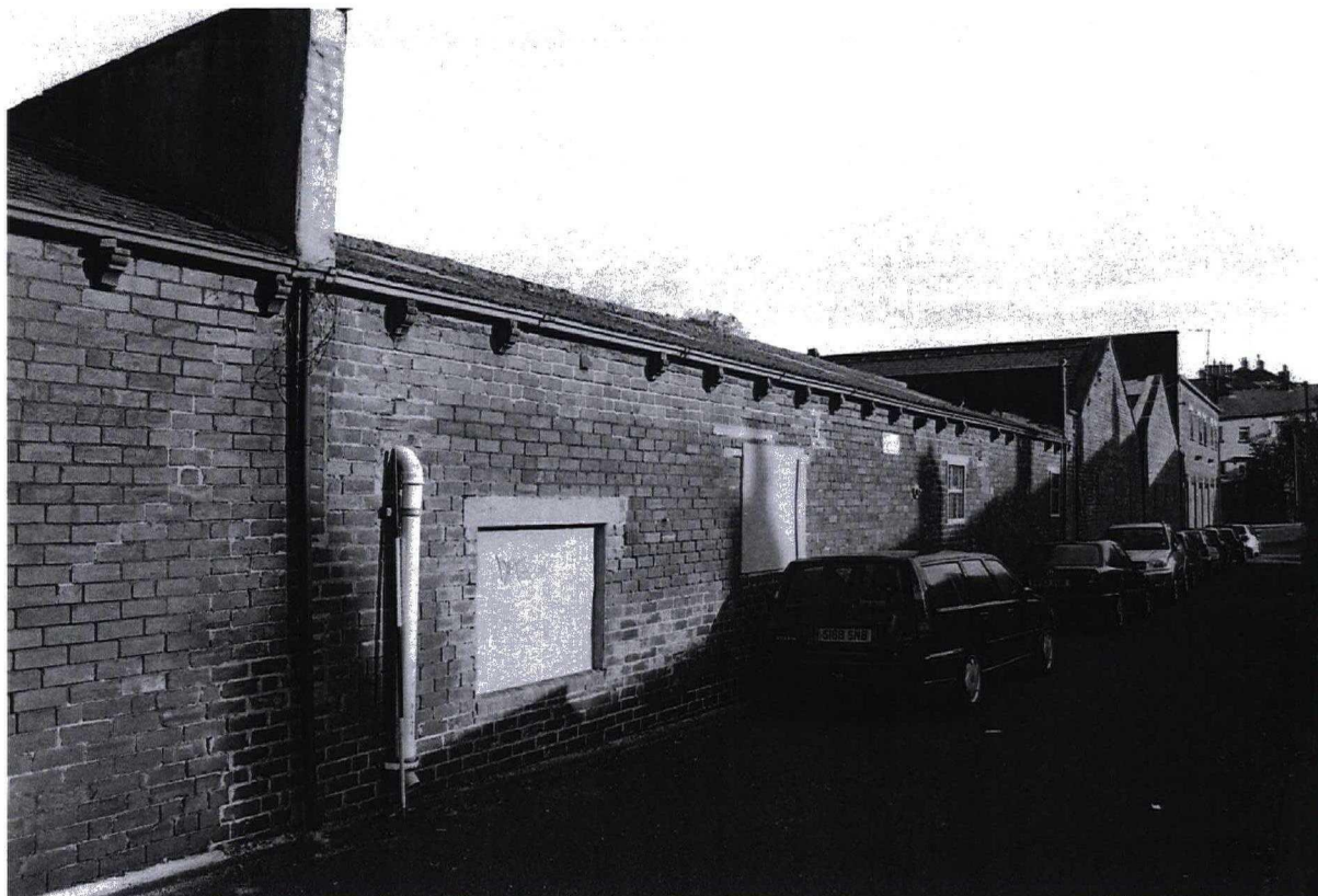
Photograph 26 9984/9 W Rear shed wall with window openings
