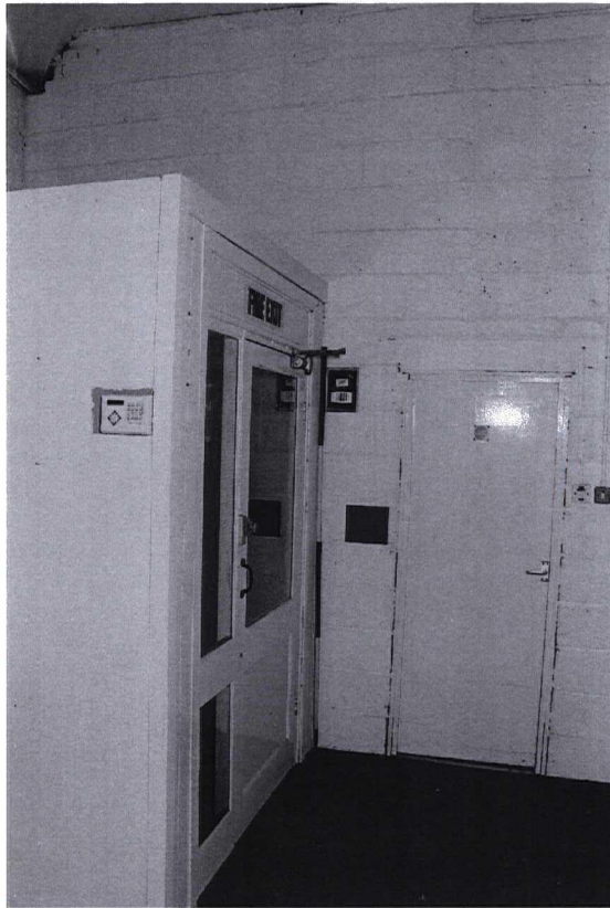
Photograph 33 9985/4 W Partitioned lobby leading to the fire exit
