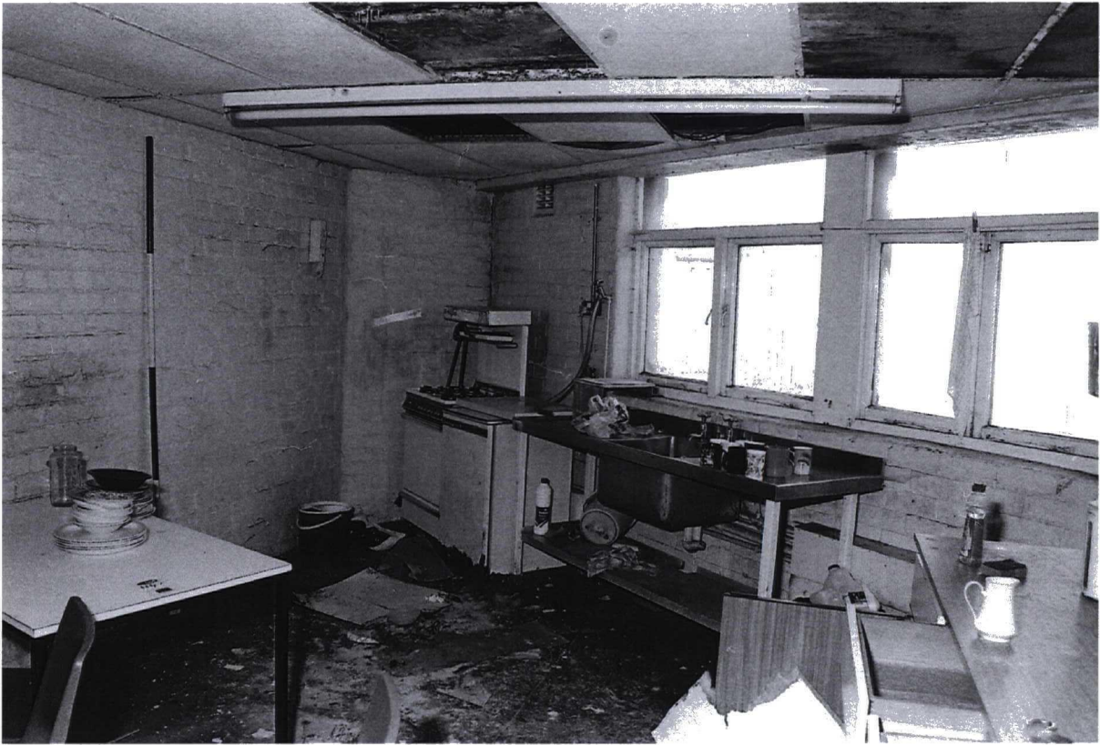
Photograph 28 9983/29 S First-floor area now used as a kitchen and rest room
