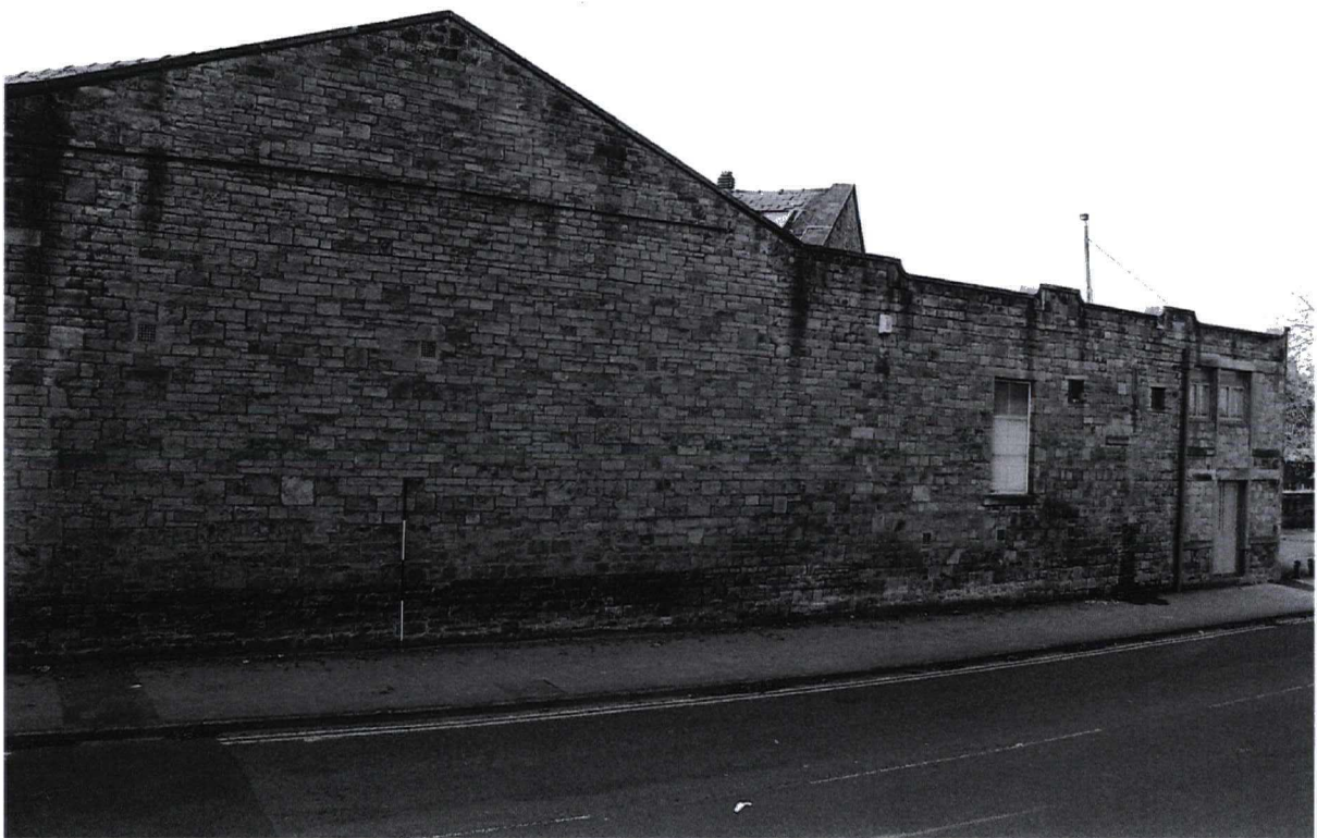
Photograph 4 9984/18 NE Angled gable wall
