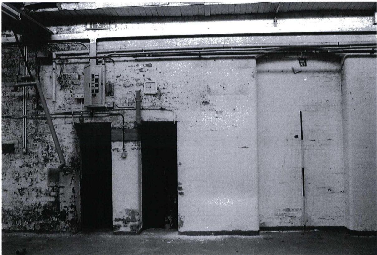
Photograph 64 9984/34 S View showing two small doorways and a large, segmental-arched, blocked opening
