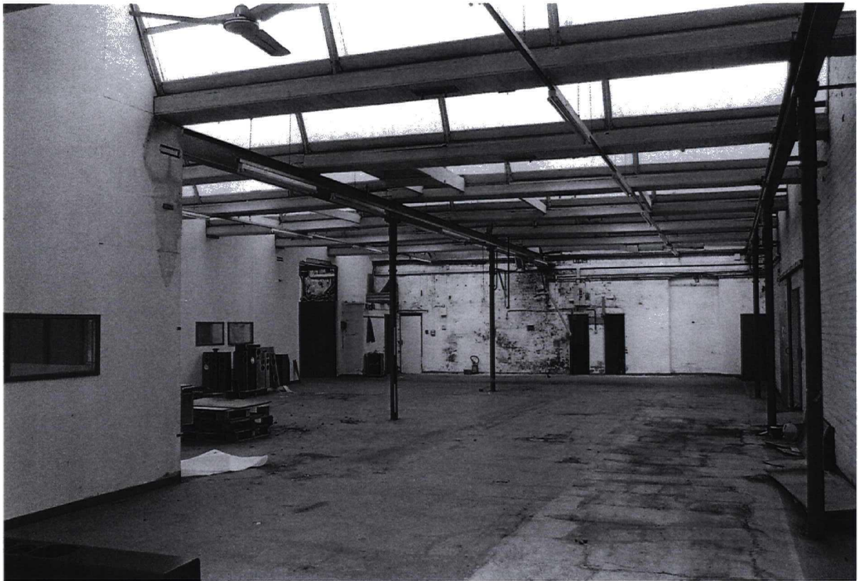
Photograph 55 9983/1 S General view showing cast-iron columns supporting steel beams
