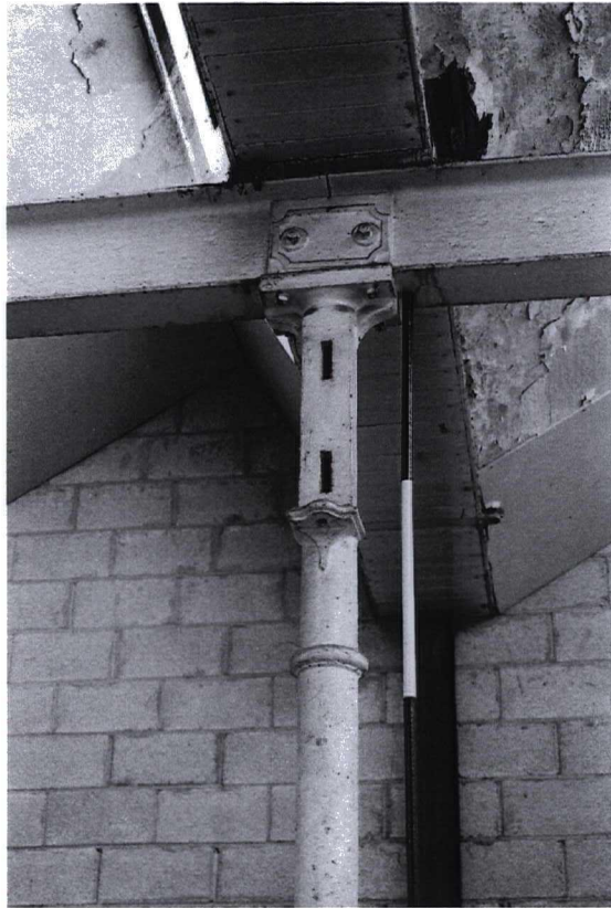
Photograph 57 9984/30 E Cast-iron column supporting steel beams
