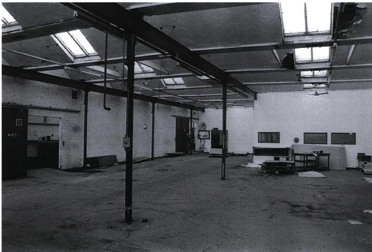
Photograph 60 9983/3 NW General view showing cast-iron columns and a later partitioned wall
