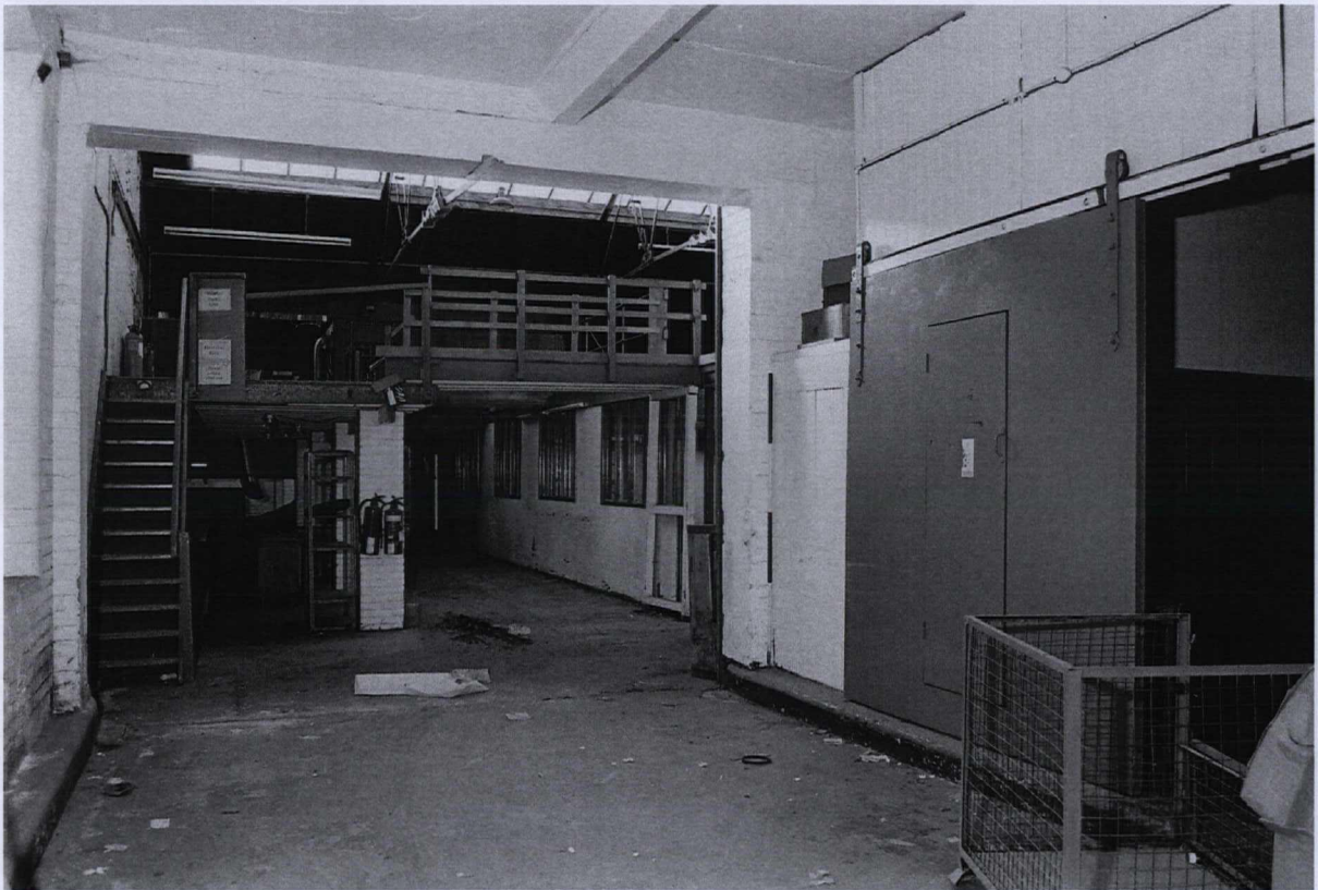
Photograph 42 9985/21 E A mezzanine floor supported on a row of brick columns
