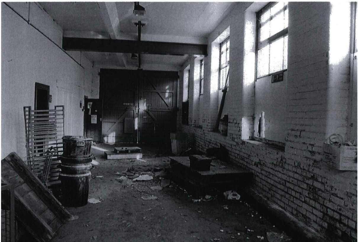
Photograph 40 9985/23 W A view of the loading bay
