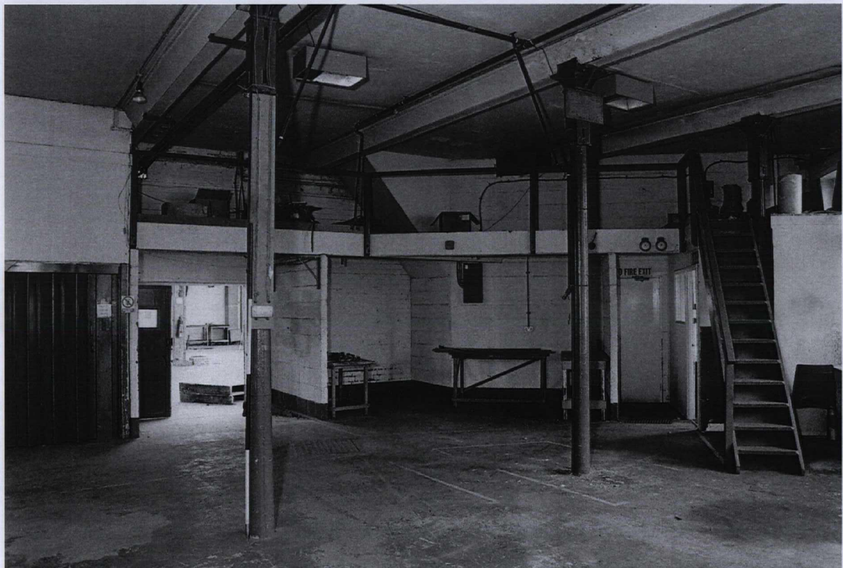
Photograph 36 9985/28 SE Cast-iron columns and a small mezzanine floor
