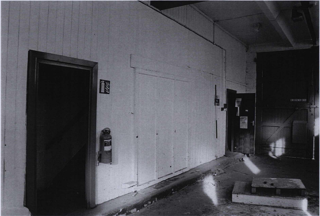
Photograph 41 W Partition wall to the side of the loading bay
