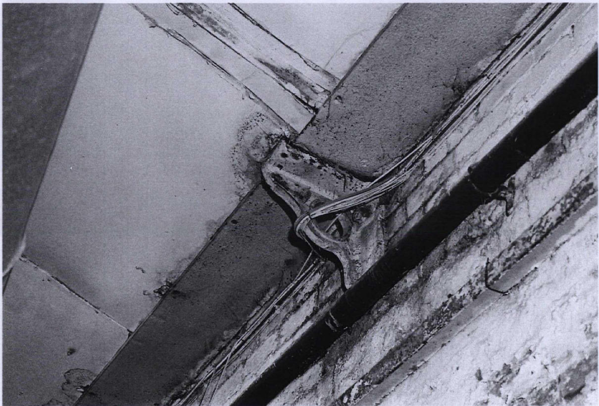
Photograph 70 9983/17 SE A cast-iron bracket supporting the side gutter
