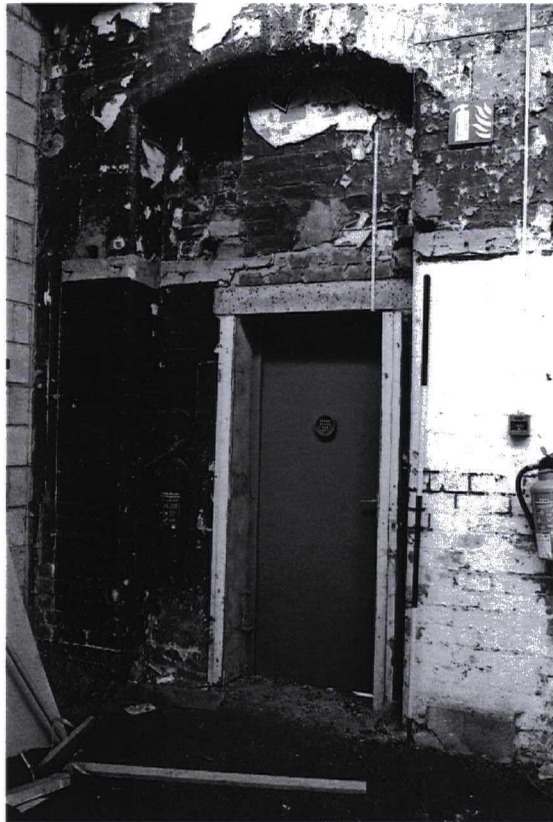
Photograph 59 9984/28 S A blocked, segmental arched, opening with a later doorway installed
