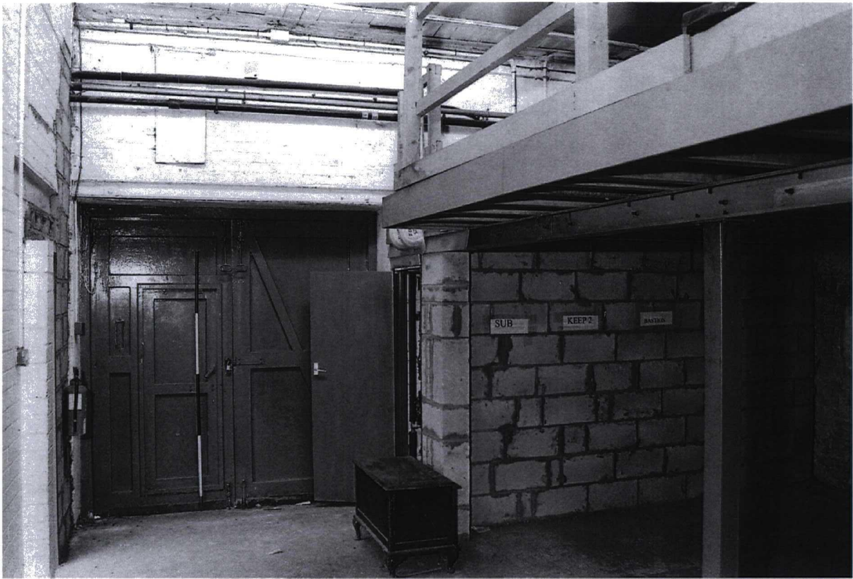
Photograph 67 9983/6 SW Large double door with a smaller door set within
