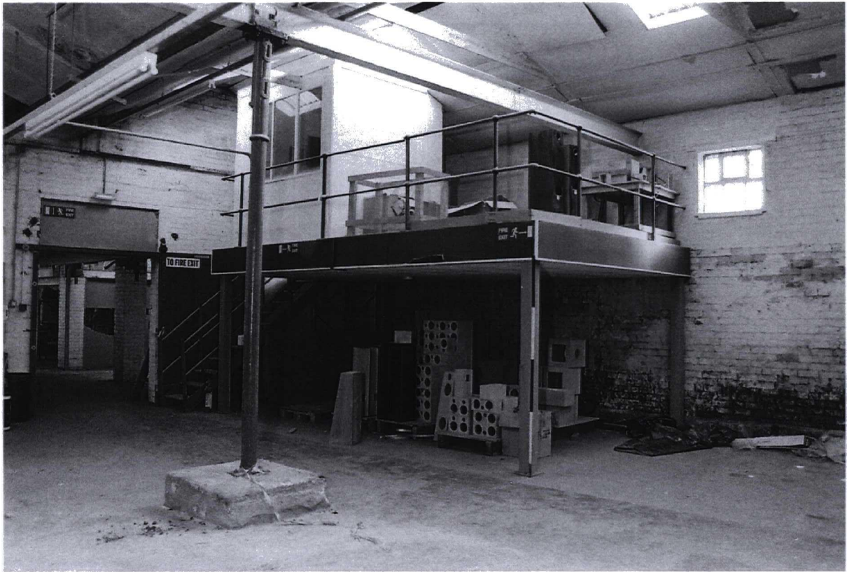
Photograph 49 9983/14 NW Mezzanine store supported on steel stanchions
