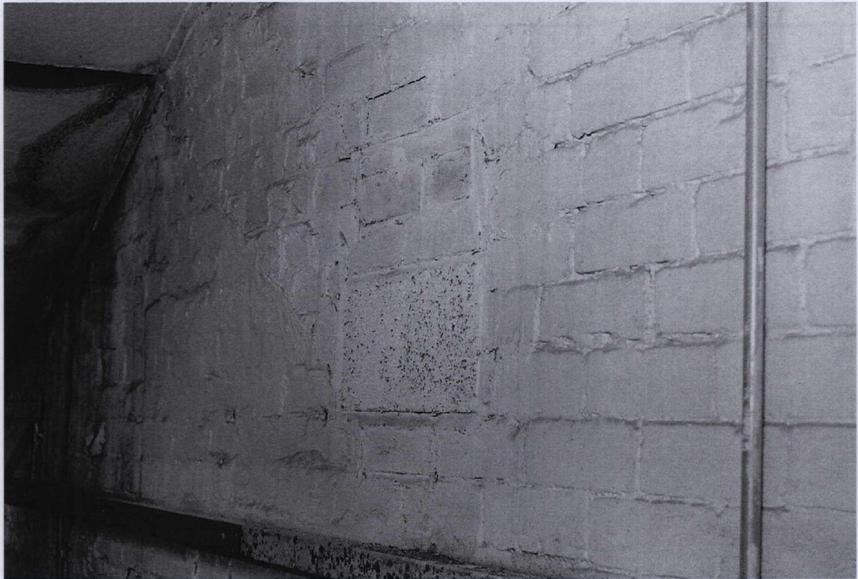
Photograph 43 9985/5 W A blocked opening, possibly a wall box
