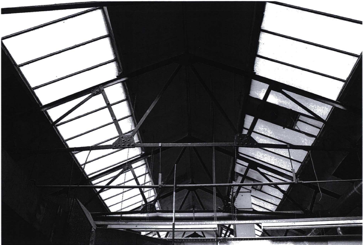
Photograph 45 9983/24 S Bolted steel roof trusses
