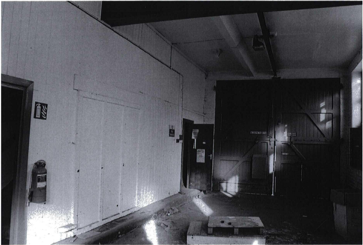
Photograph 39 9985/22 W Large double loading doors
