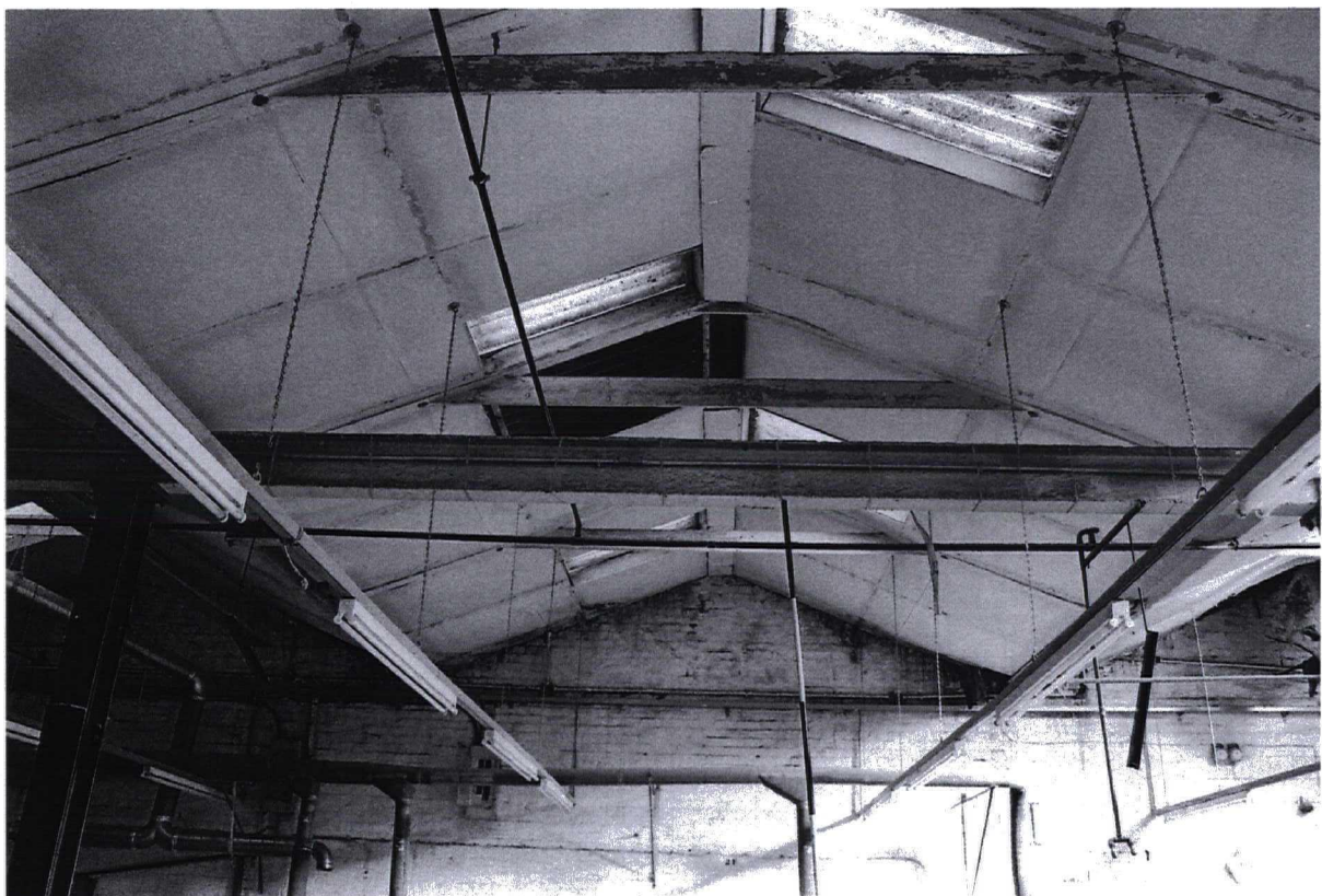
Photograph 80 9983/21 W Roof trusses and supporting detail
