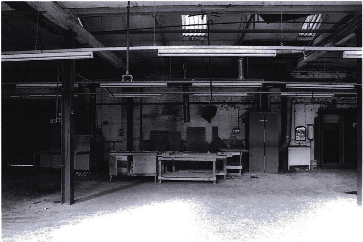
Photograph 79 9983/16 S View showing steel stanchions supporting riveted, steel, 'I' section beams
