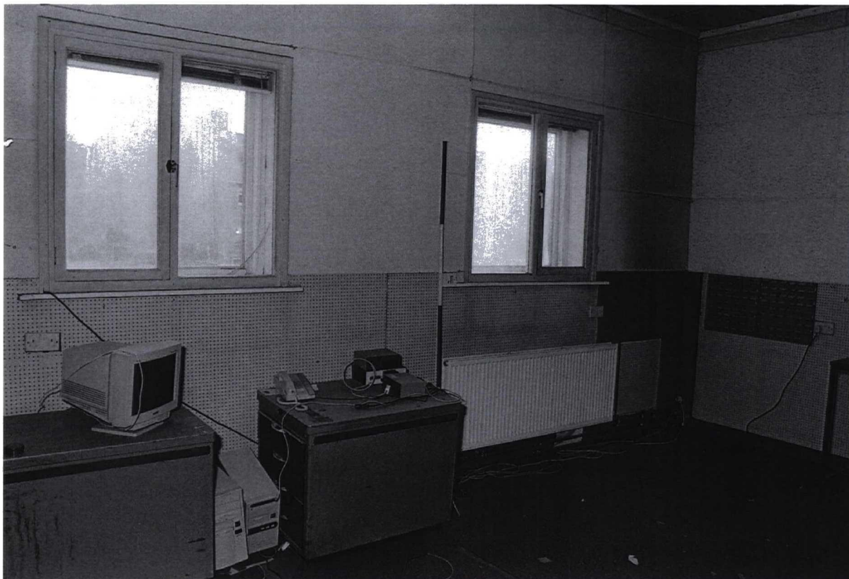
Photograph 91 9985/18 NE A pair of double side-opening casement windows
