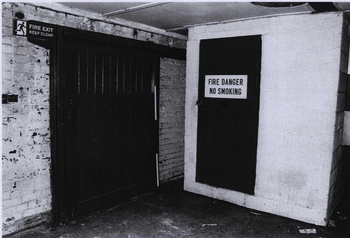
Photograph 71 9983/36 SE Large side-opening fire door with later breeze-block store room
