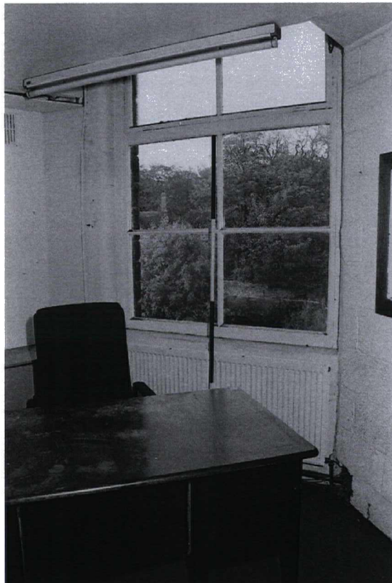
Photograph 88 9985/8 SW A two-over-three top-opening casement window
