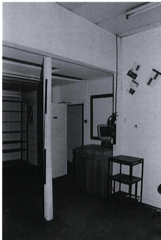
Photograph 86 9985/9 NW A cast-iron column encased in modern office partitions
