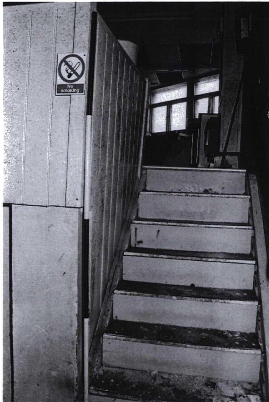
Photograph 75 9983/28 S Wooden stairs leading to the first floor
