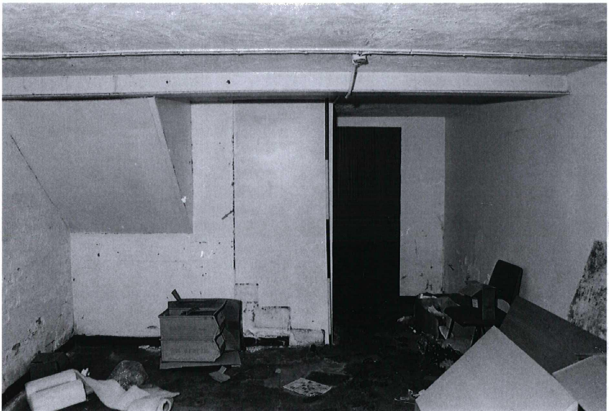
Photograph 74 9983/31 N Former office with hidden stair
