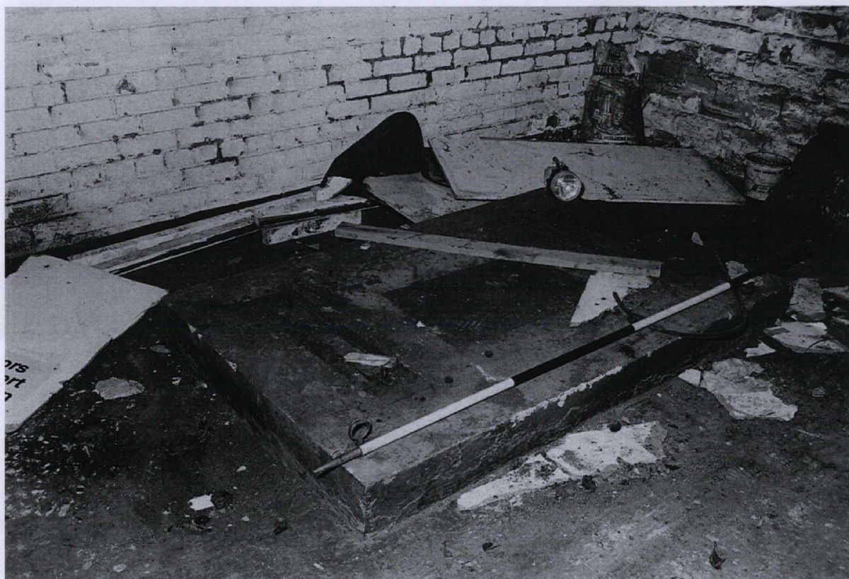
Photograph 72 9985/29 NW Concrete machine bed
