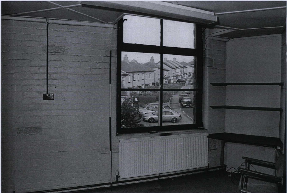
Photograph 90 9985/6 SW Detail of a casement window
