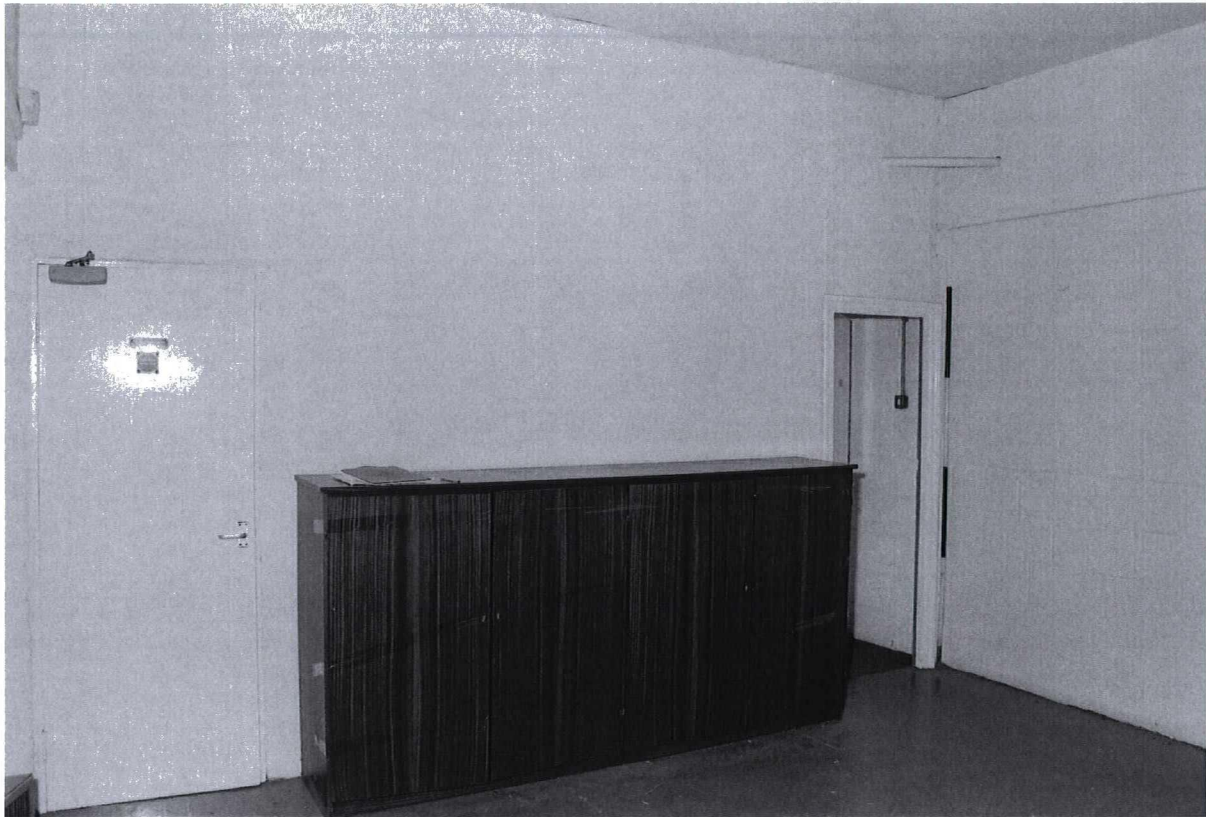
Photograph 85 9985/14 SW Two doorways within an internal partition
