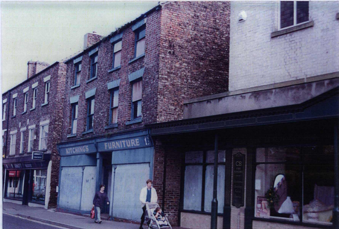
PLATE 1 FRONT OF 2A-4 CASTLEGATE BEFORE WORK STARTED
