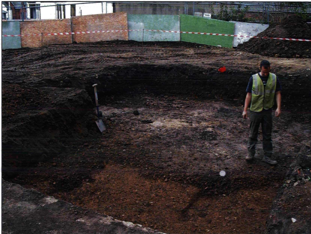
Plate 1. Trench 1 during clean up.
