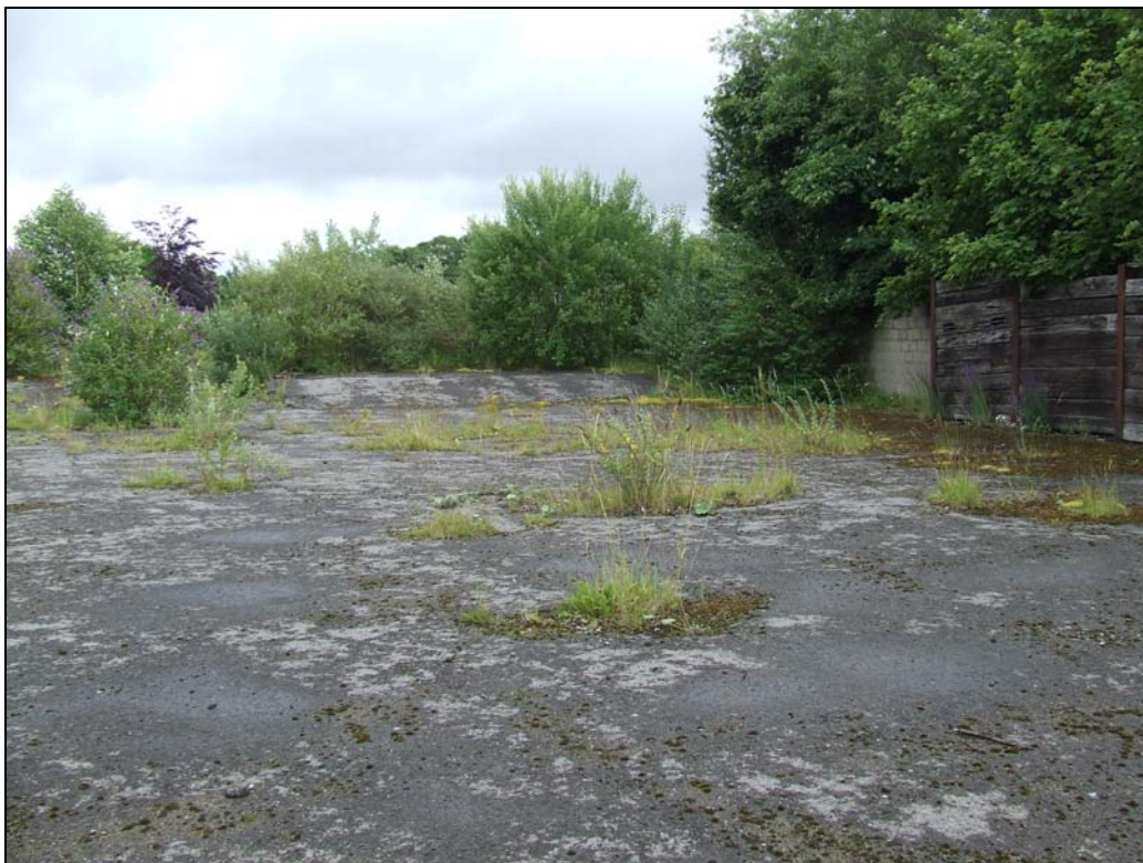
Figure 10 Interior of depot looking north
