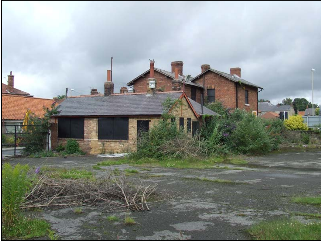
Figure 9 The buildings on site, looking northwest
