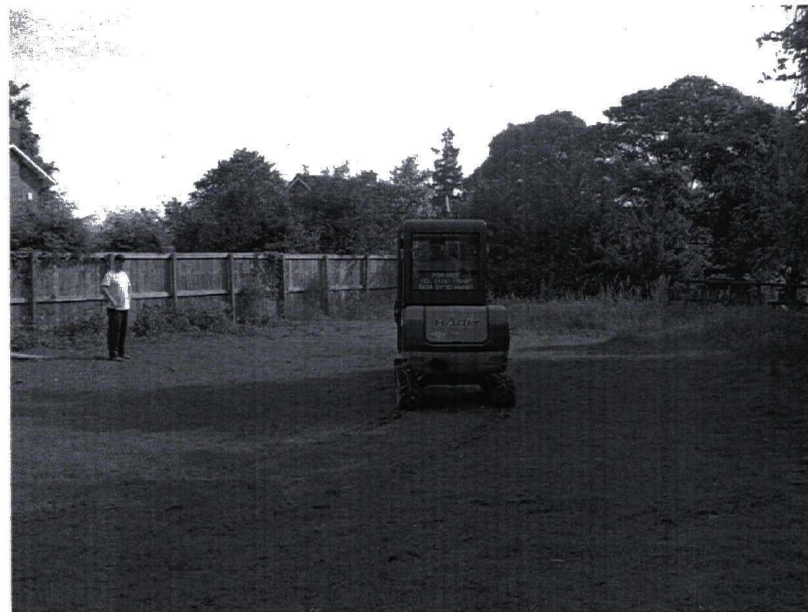
Plate 2. Area of Trench 3 before excavation. Facing North-east.
