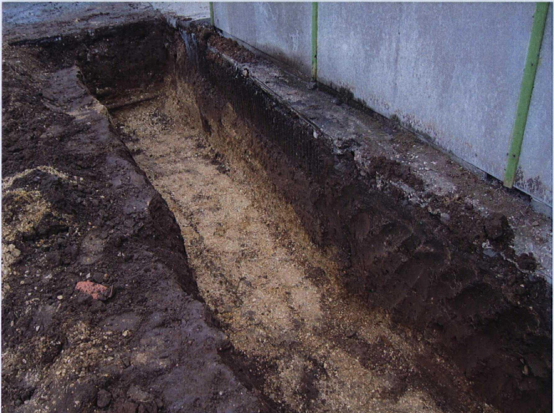
Plate 2: View of Foundation Trench. Facing South-east.
