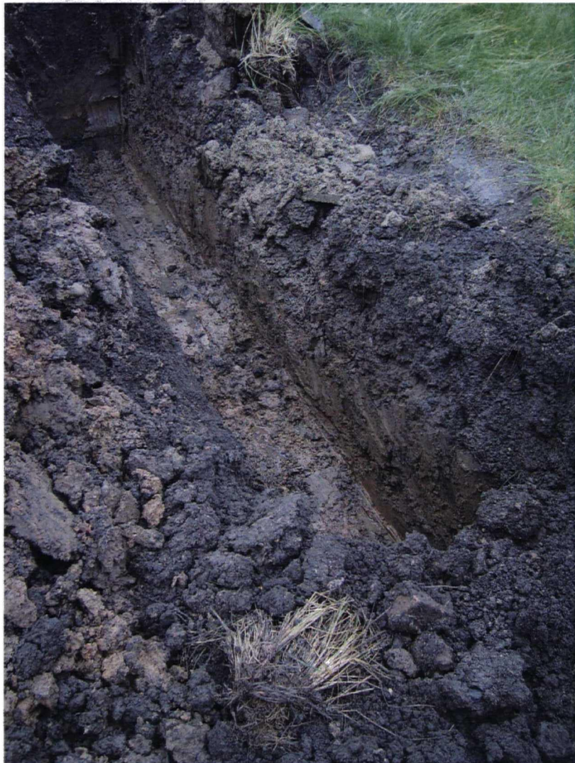
Plate 2: View of Foundation. Facing South-east.
