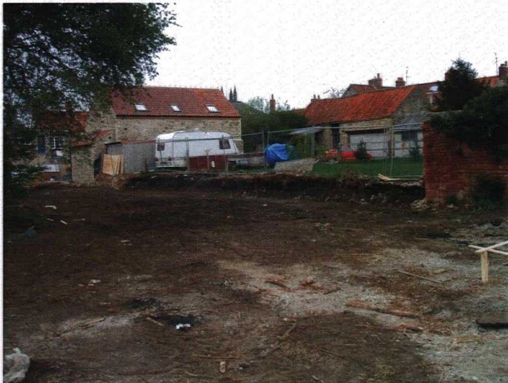
Plate 1 Site after vegetation/partial topsoil strip, looking W
