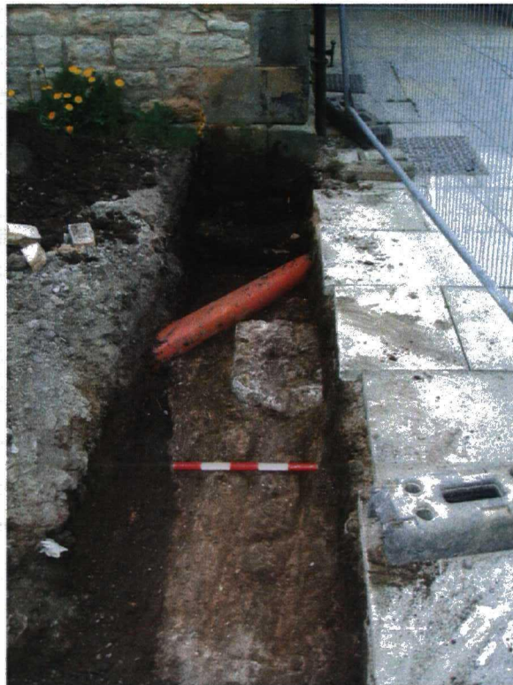
Plate 2 Wall foundations in S foundation trench, looking E
