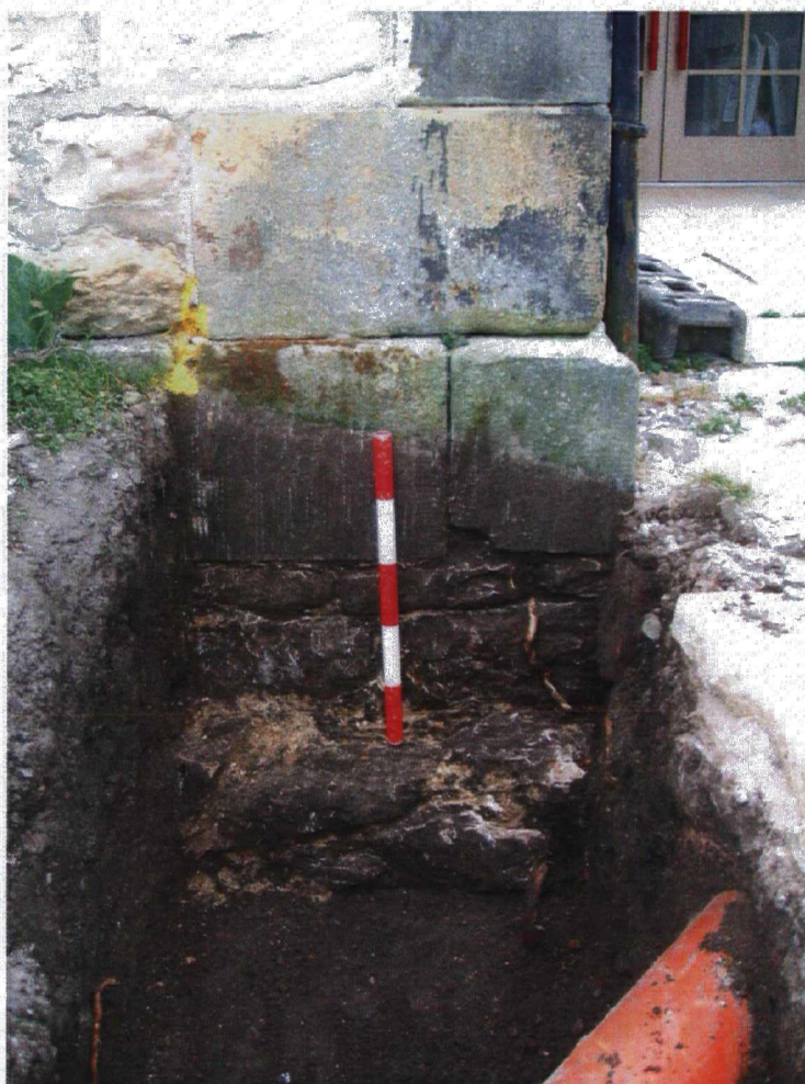
Plate 1 Foundations of SE corner of Meeting House in S foundation trench/column Pit 5, looking E
