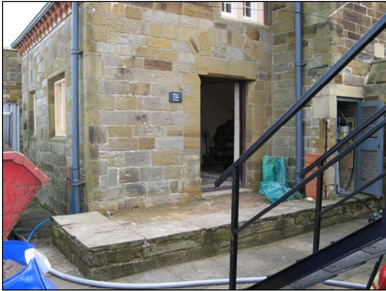
Figure 17: Lodge step before excavation. Looking south east.
