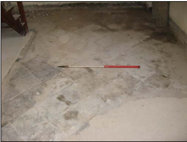
Figure 15: Stone flag floor F2 below concrete 1 (visible in foreground). Looking east.
