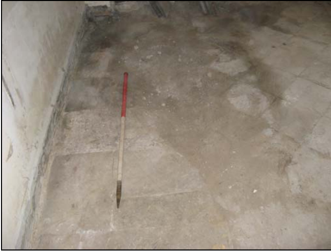
Figure 14: Cut for pipe F9 visible through floor F2. More coarse irregular paving to east and regular decorative paving to west – presumably reflecting earlier division represented by wall F5. Looking south.
