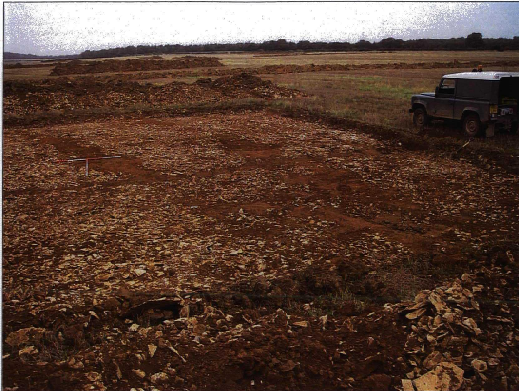
Plate 33. Trench 28 showing Gully 242, looking north-east
