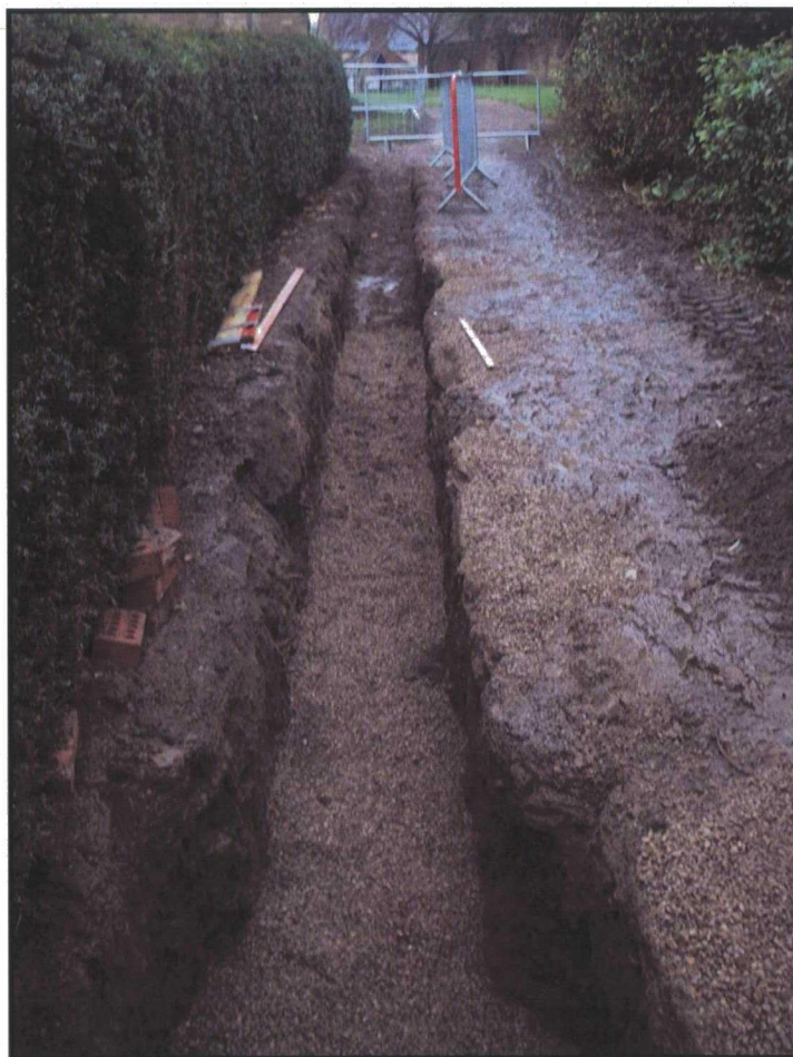
Plate 3. The pipe trench
