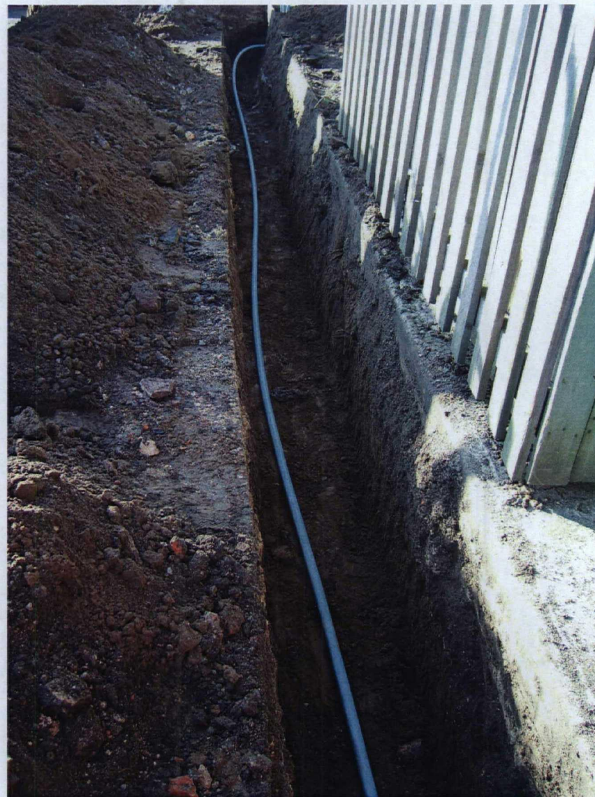
Plate 4: Water Pipe Trench. Facing West.
