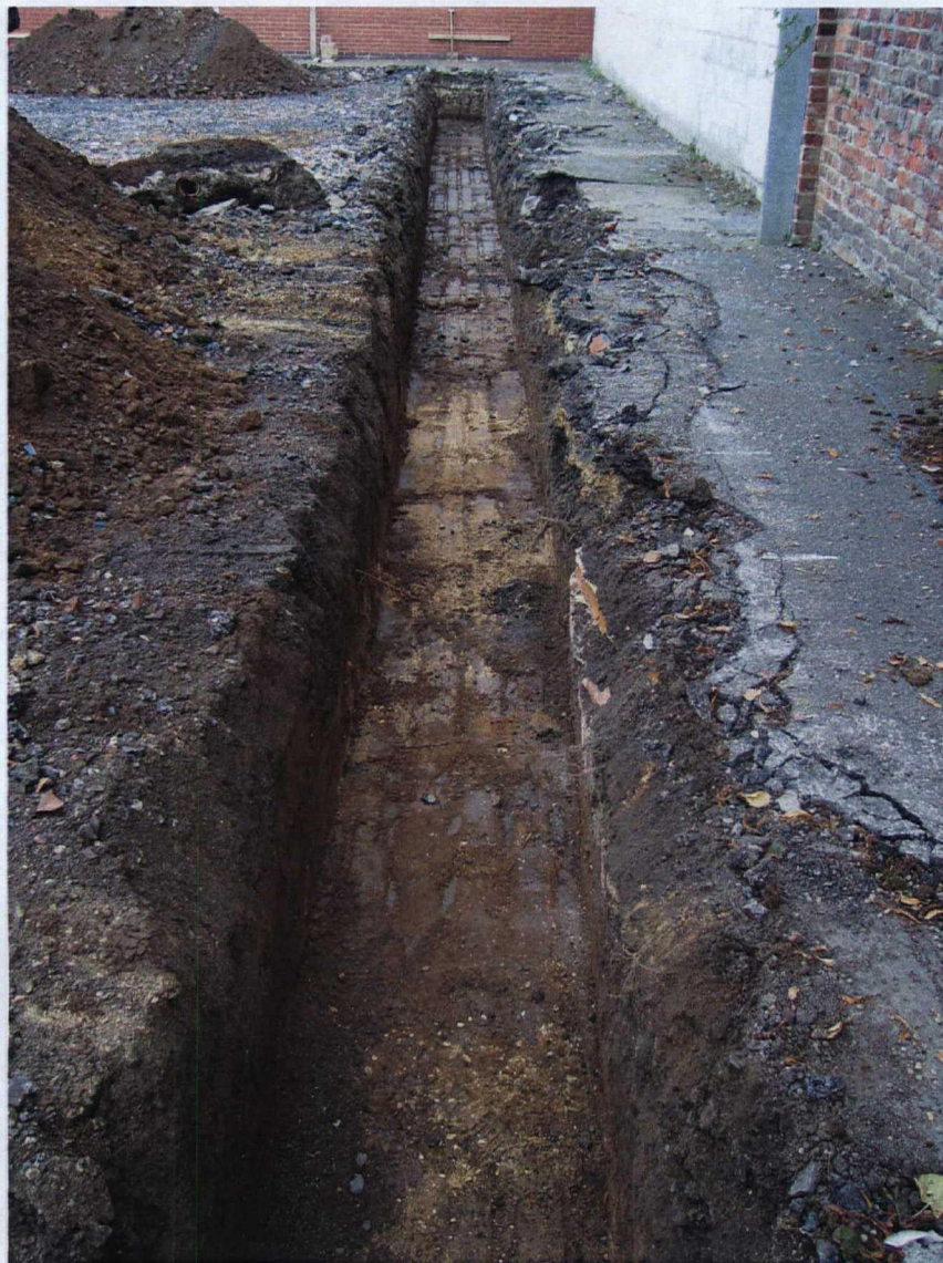
Plate 3: Eastern Foundation. Facing North.
