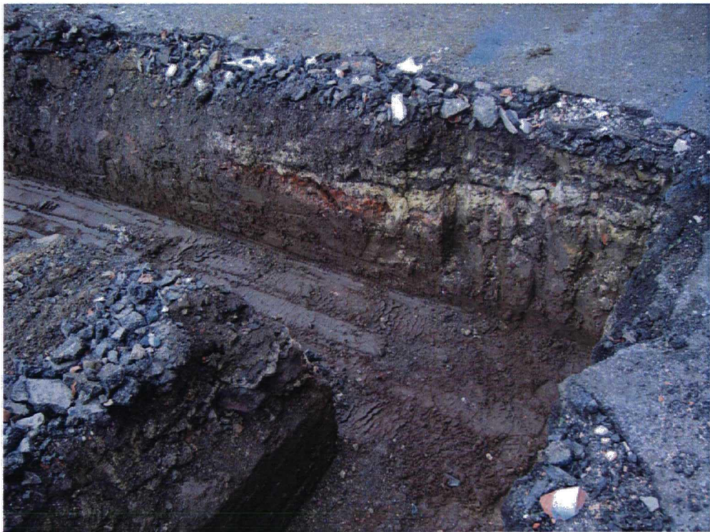
Plate 2. Foundation Detail. Facing North West
