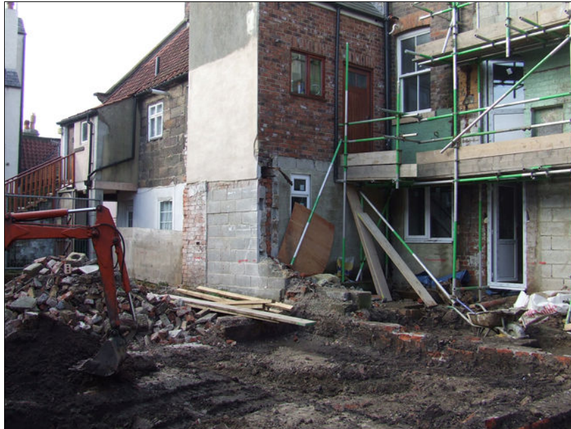
Plate 10 General view of the rear of 26a and 27a Silver Street
