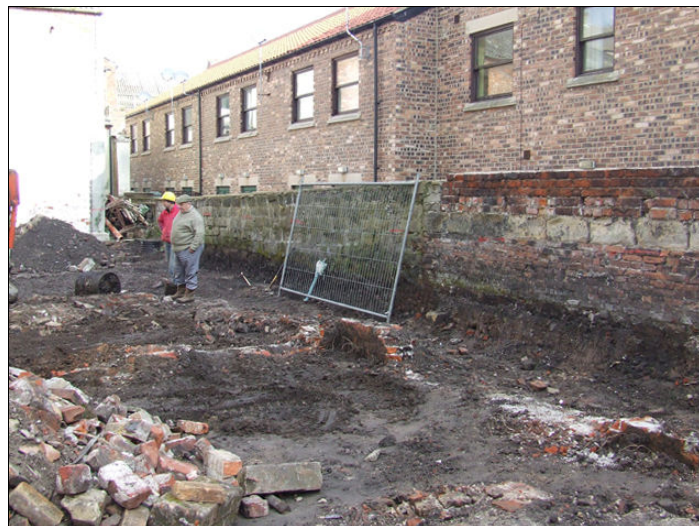
Plate 9 Eastern site boundary wall
