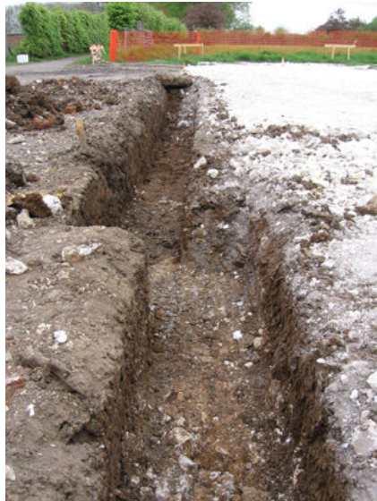
Plates 5 & 6 Northern and southern strip footings during excavation, looking east
