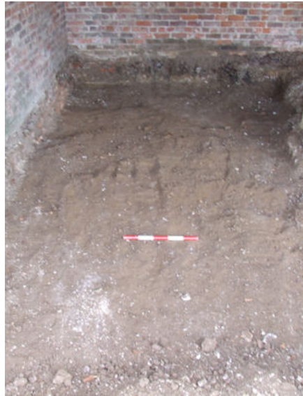
Plates 3 & 4 Exposed wall footings inside barn, after ground reduction and in strip footing
