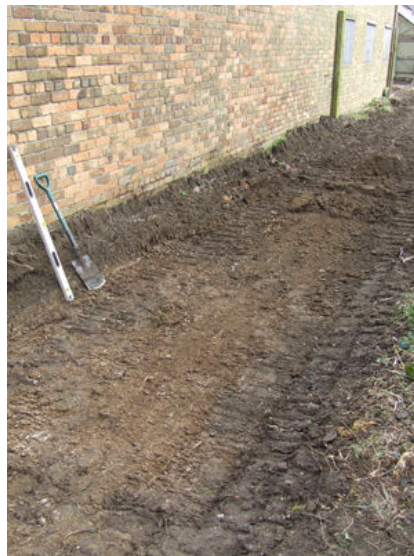
Plate 2 Final ground reduction behind barn, looking north-east
