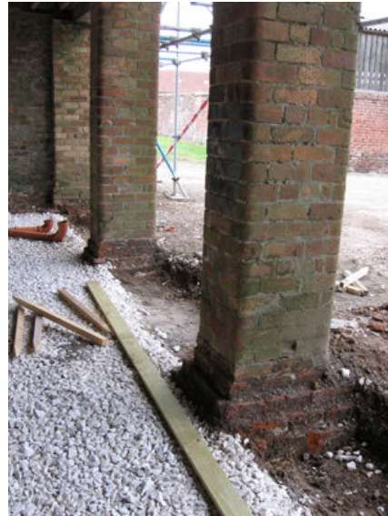
Plates 3 & 4 Exposed wall footings inside barn, after ground reduction and in strip footing
