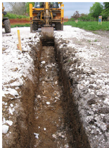
Plates 5 & 6 Northern and southern strip footings during excavation, looking east
