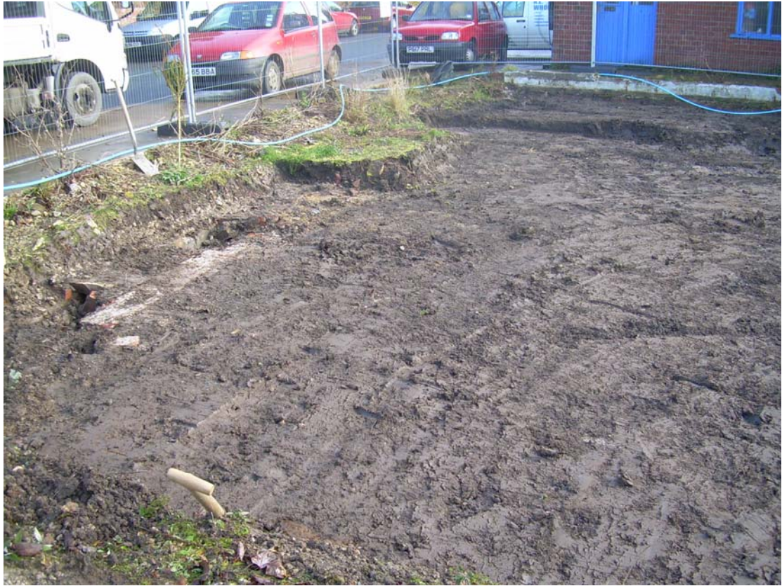
Plate 3. Slab Foundation Strip. Facing East.
