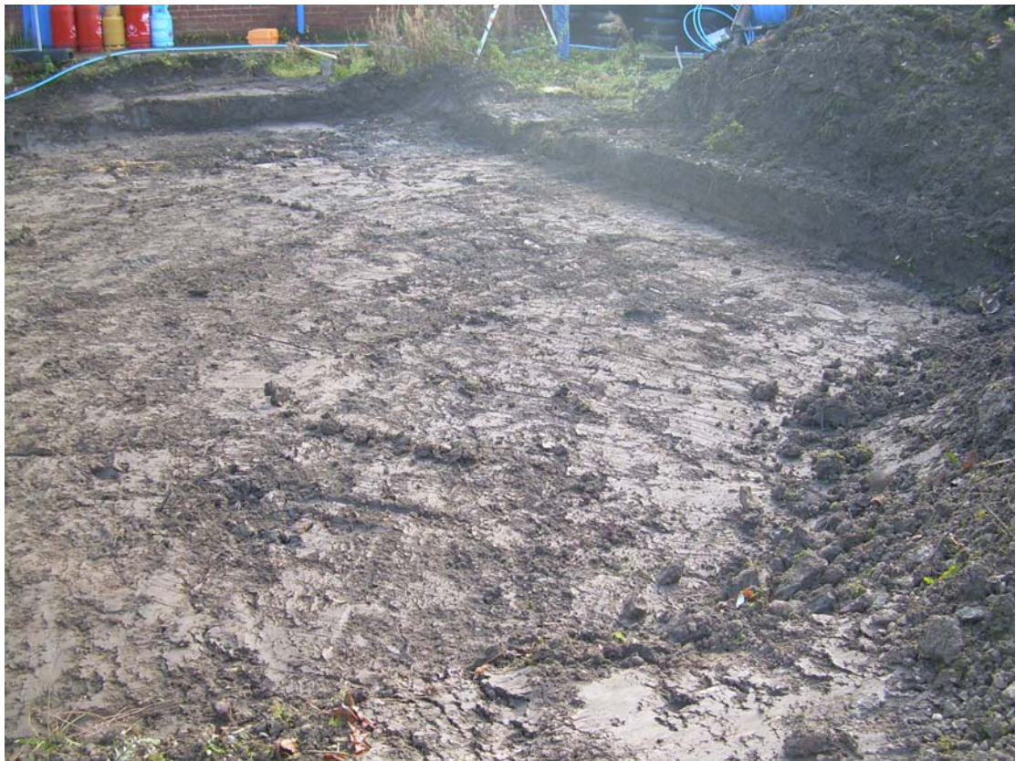
Plate 4. Slab Foundation Strip. Facing South-east.
