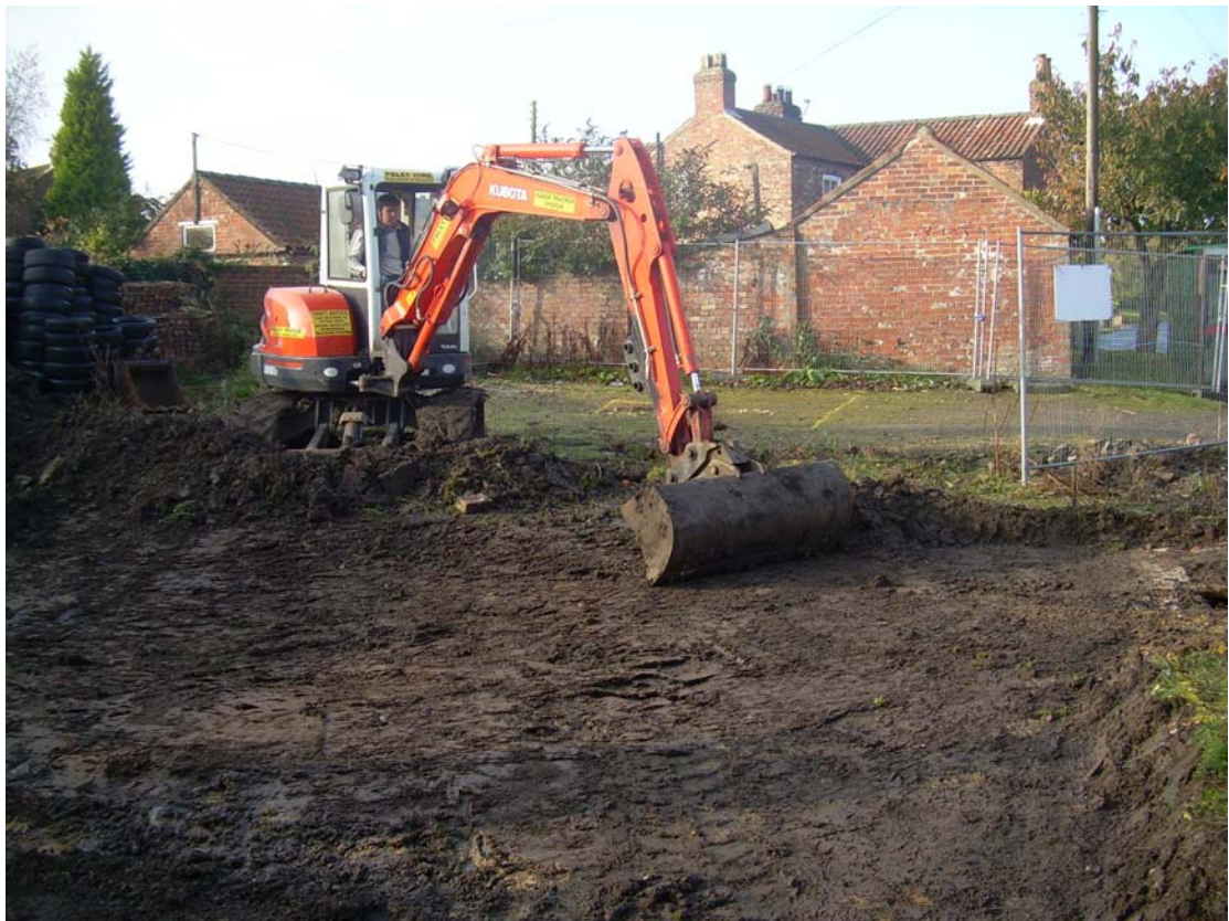
Plate 2. Slab foundation Strip. Facing West.
