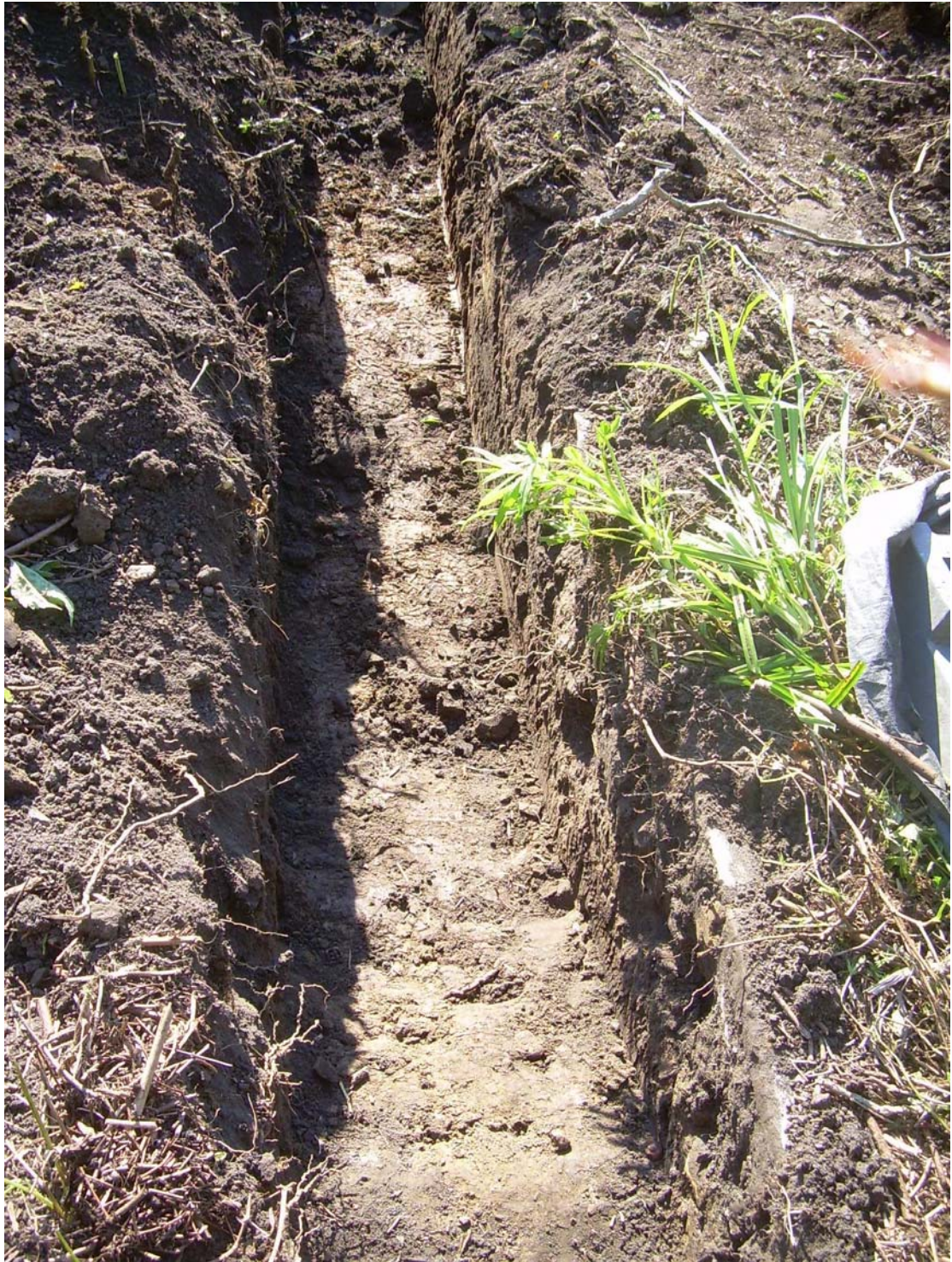
Plate 6. Area of Strip Foundation. Facing East.
