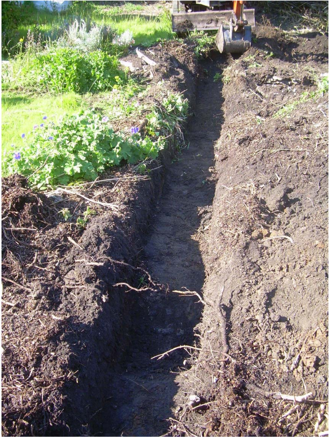
Plate 5. Area of Strip Foundation. Facing South.
