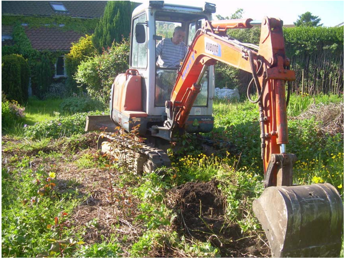
Plate 3. Site before vegetation strip. Facing East.
