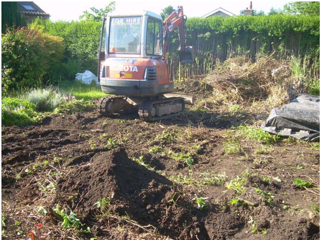
Plate 4. Site after vegetation strip. Facing South-east.
