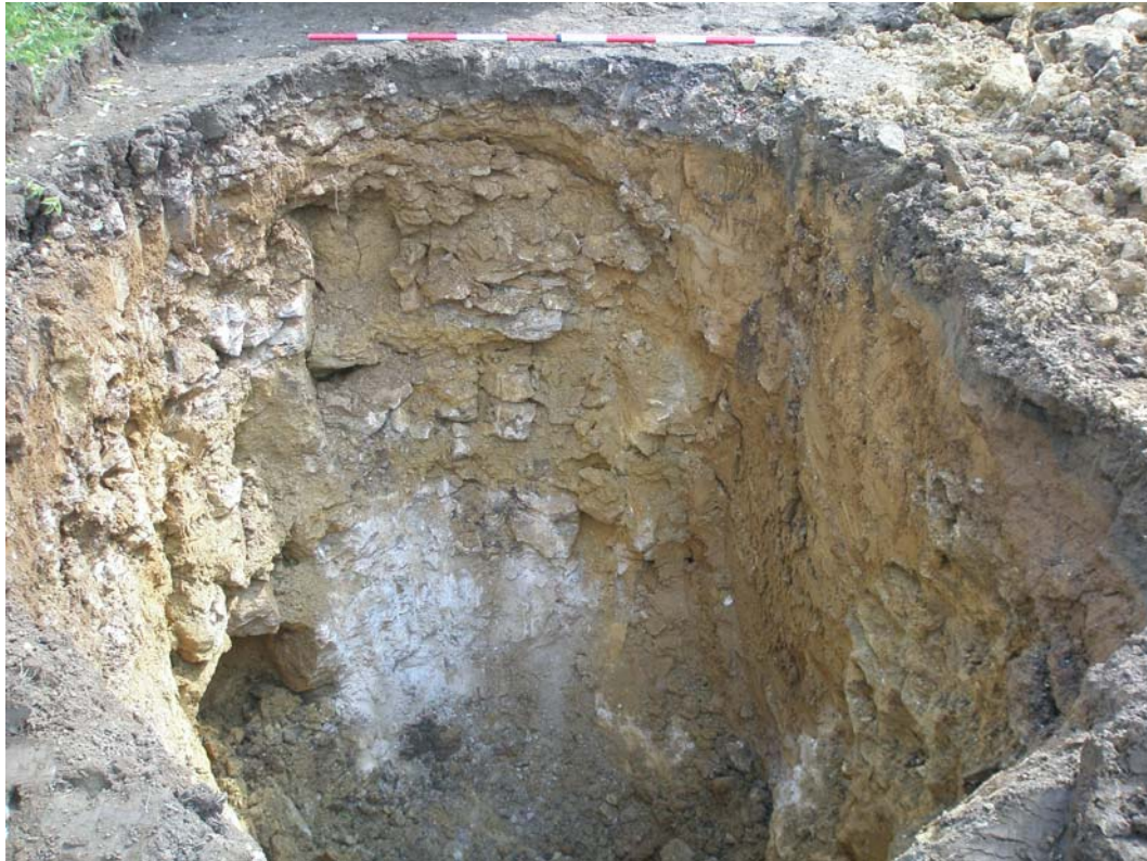
Plate 5 Contexts (1001)-(1003), septic tank excavation 1
