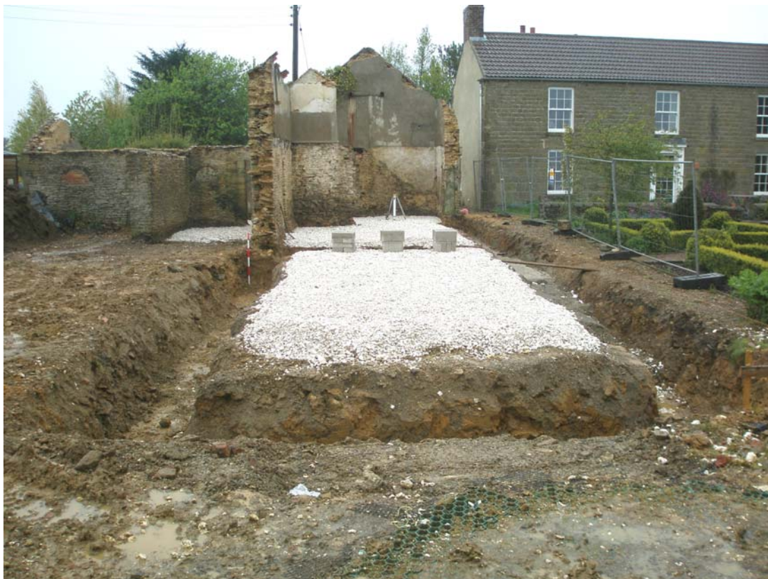
Plate 6 Foundation trenches for building B extension, viewed from the south
