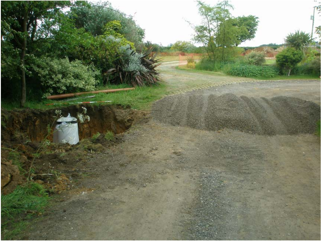
Plate 7 Septic tank excavation 2, viewed from the east
