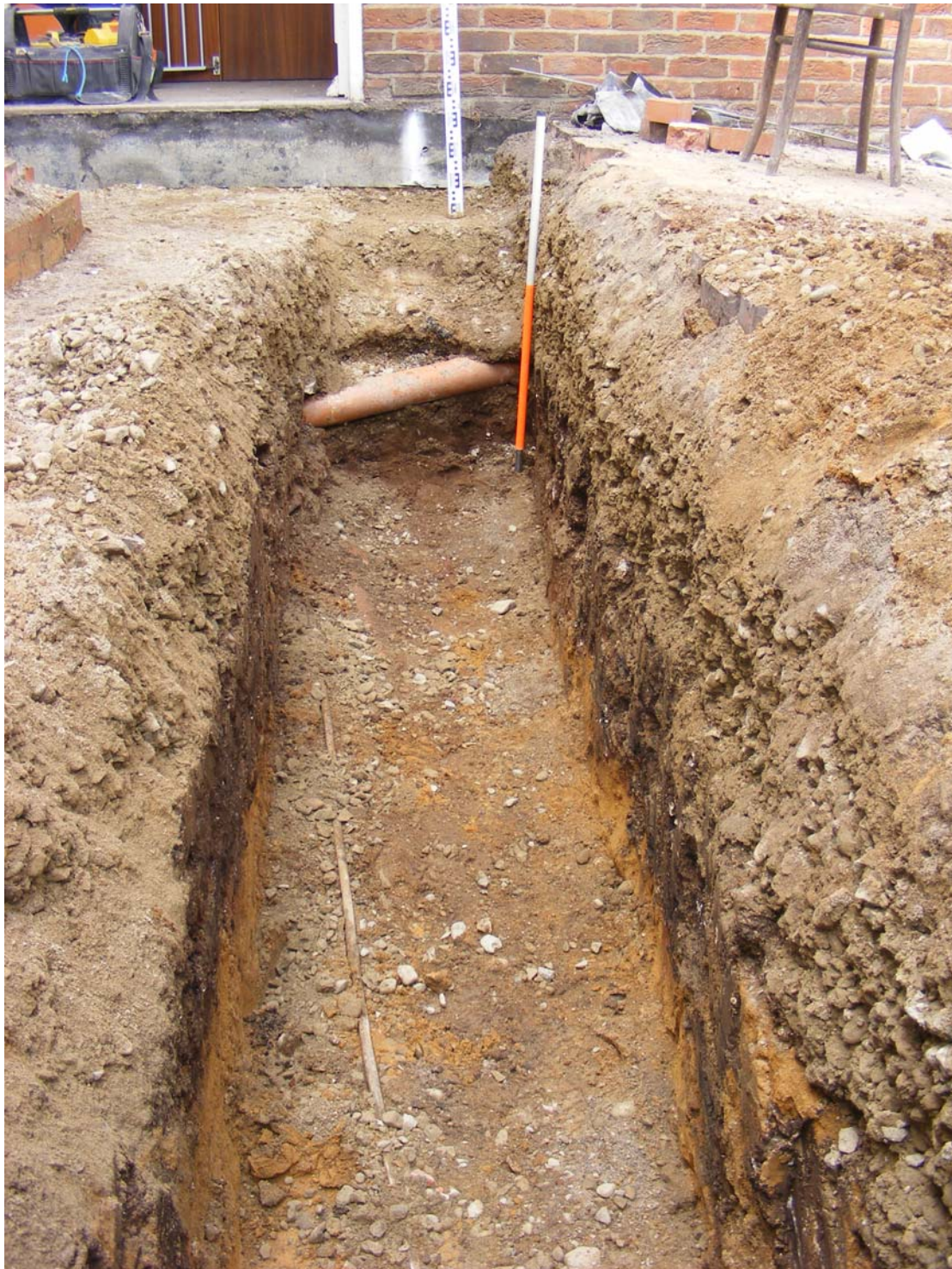
Plate 1. Services 3, 4 and 6 Within Foundation Trench. Facing West
