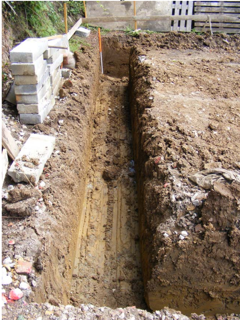
Plate 2. Foundation Trench. Facing East
