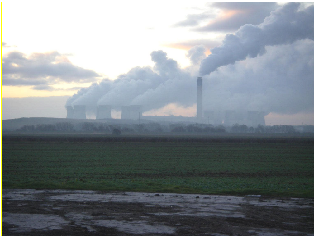
Photograph 10 – View across site from Cleek Hall, showing Drax power station
