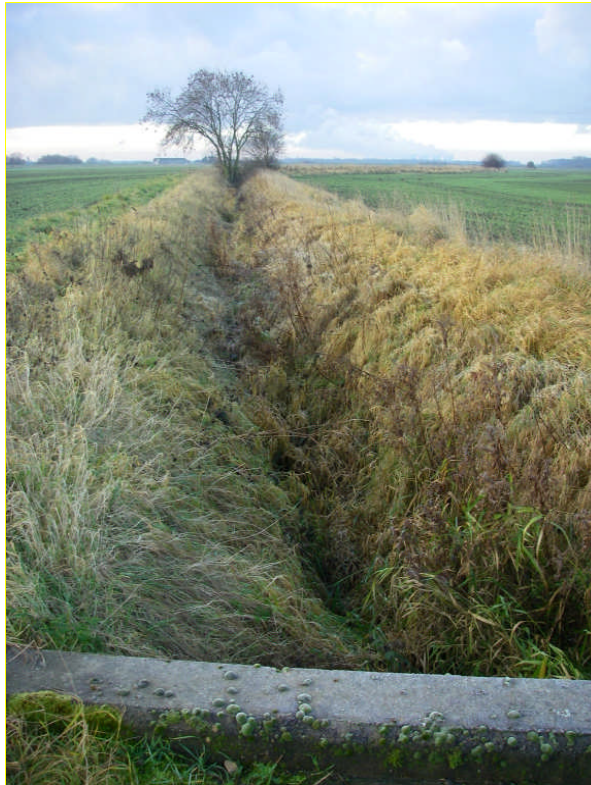
Photograph 3 – Southern drainage ditch running southwest from larger drain, viewed facing southwest
