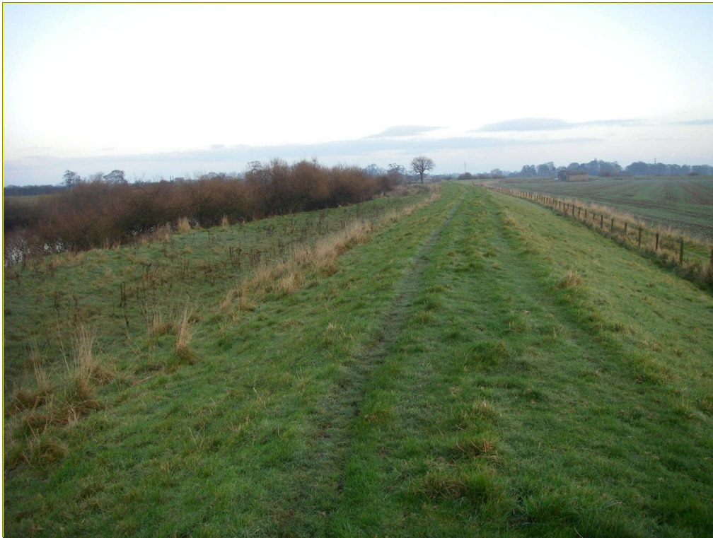
Photograph 9 – View northeast along embankment at Thief Lane End Reach
