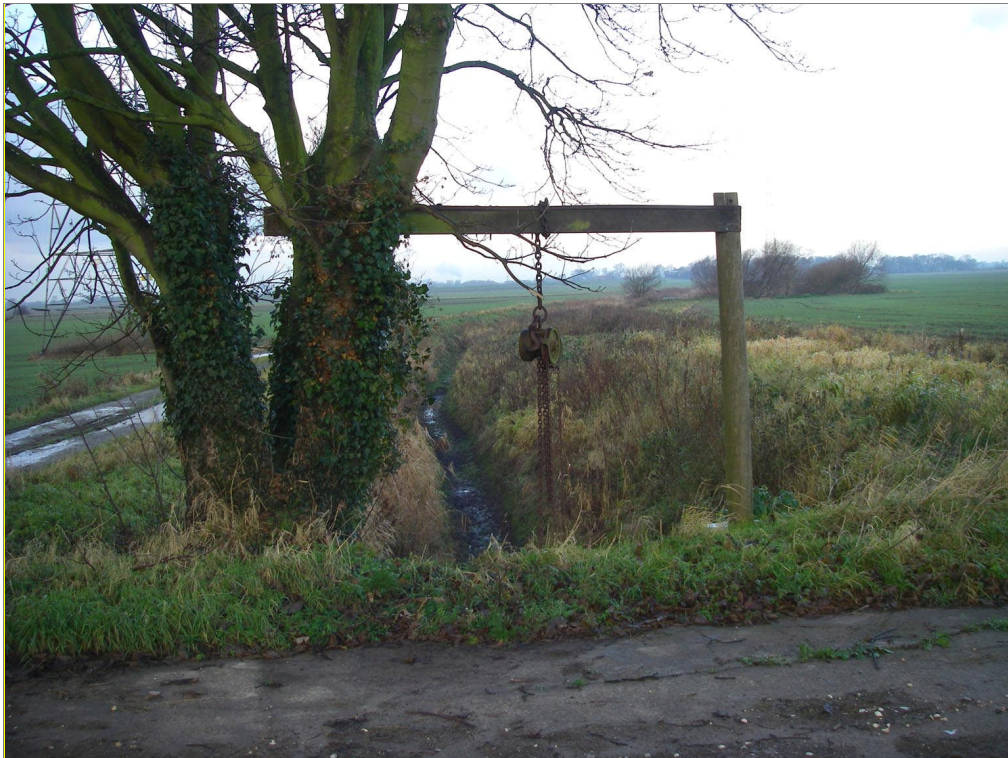
Photograph 5 – Larger drain along eastern boundary, sluice gate mechanism in foreground, viewed facing northwest
