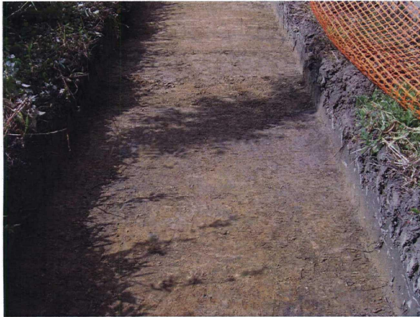
Plate 21. Trench 5 – General View. Facing North.
