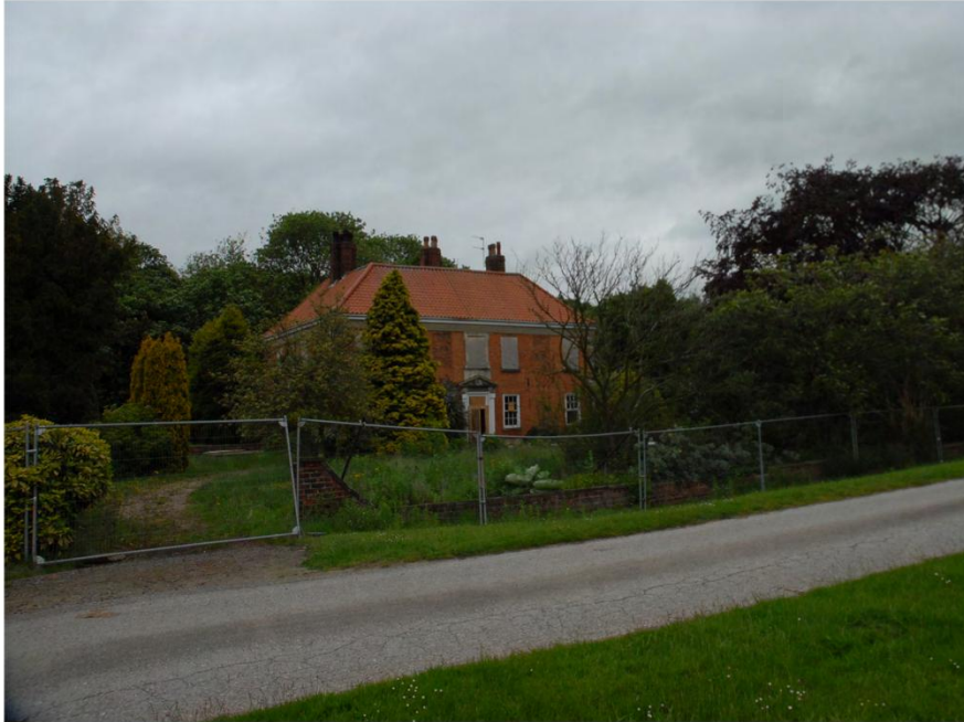
Plate 1. General view of Stanor Hall. Facing North-east.
