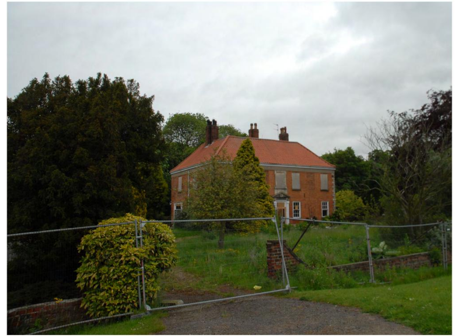
Plate 4. General View of Staynor Hall. Facing North-east.
