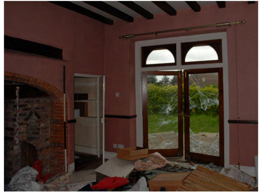
Plate 32. Staynor Hall: Interior Ground Floor. Facing South-west.
