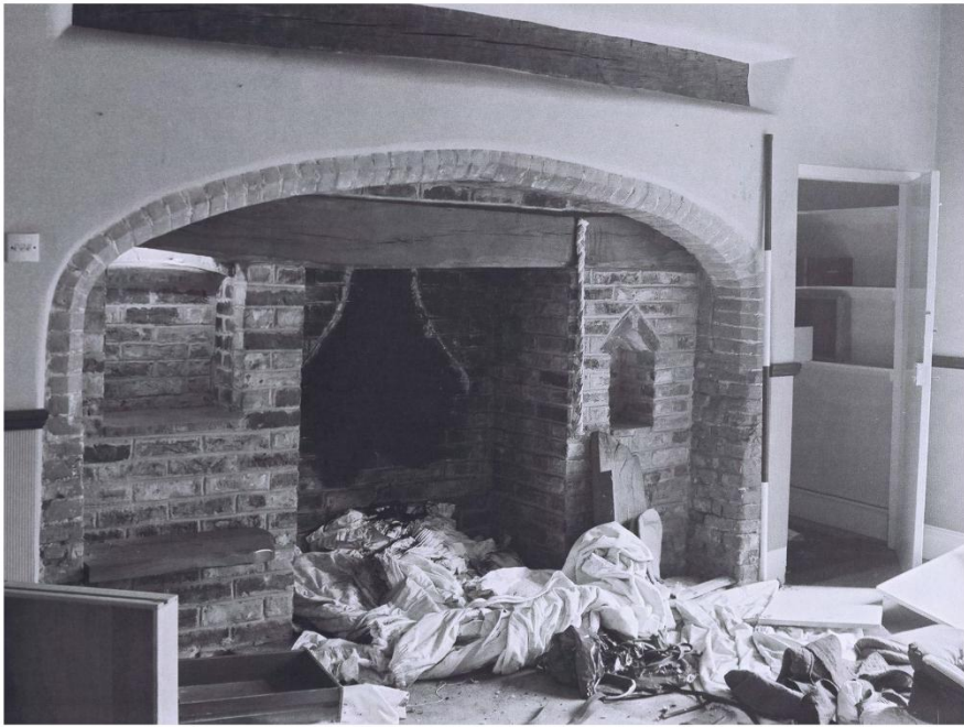
plate 31. Staynor Hall: Interior Ground Floor. Facing South.
