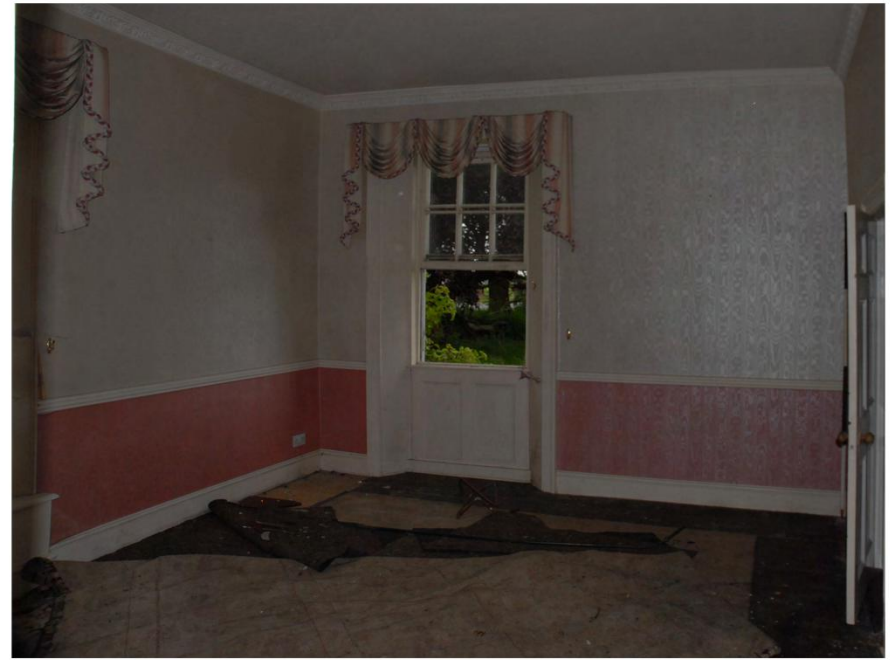
Plate 24. Staynor Hall: Interior Ground Floor. Facing South.
