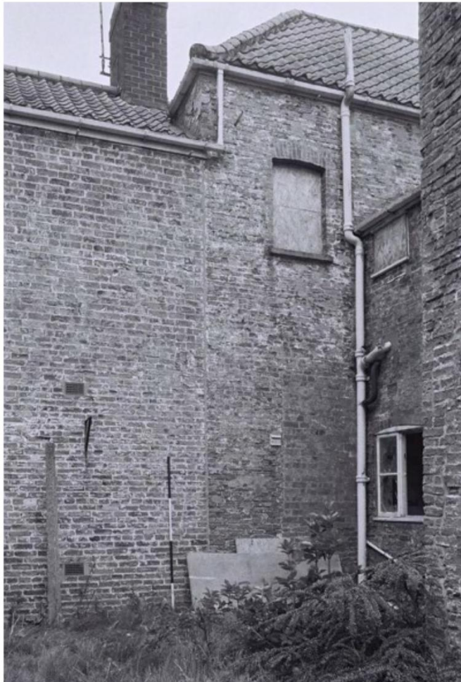
Plate 11. Staynor Hall: Exterior West Elevation East Wing. Facing East.
