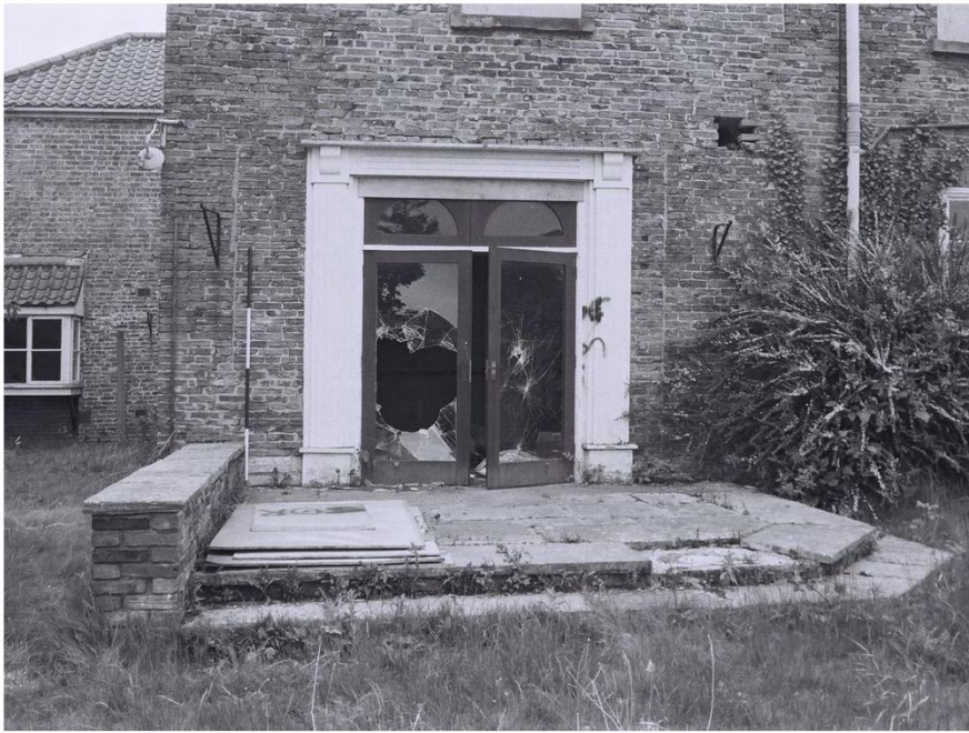
Plate 9. Staynor Hall: Exterior West Elevation. Facing East.
