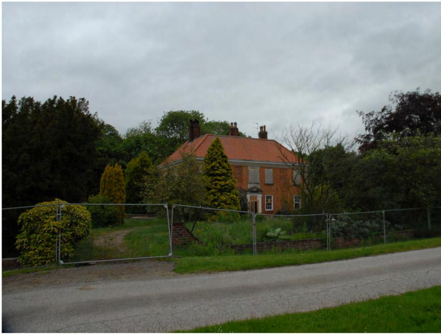
Plate 3. General View of Staynor Hall. Facing North-east.
