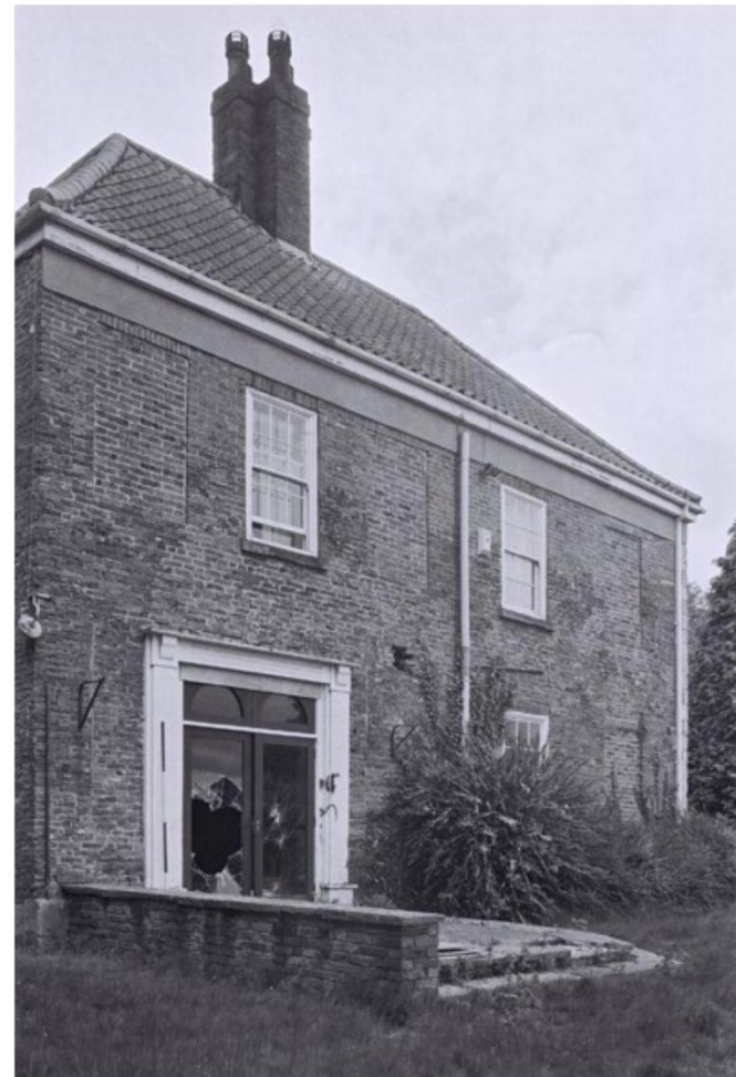
Plate 8. Staynor Hall: Exterior West Elevation. Facing South-east.
