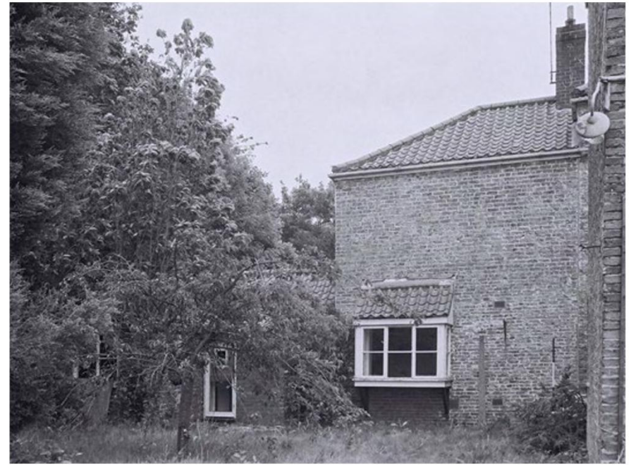
Plate 10. Staynor Hall: Exterior West Elevation East Wing. Facing East.
