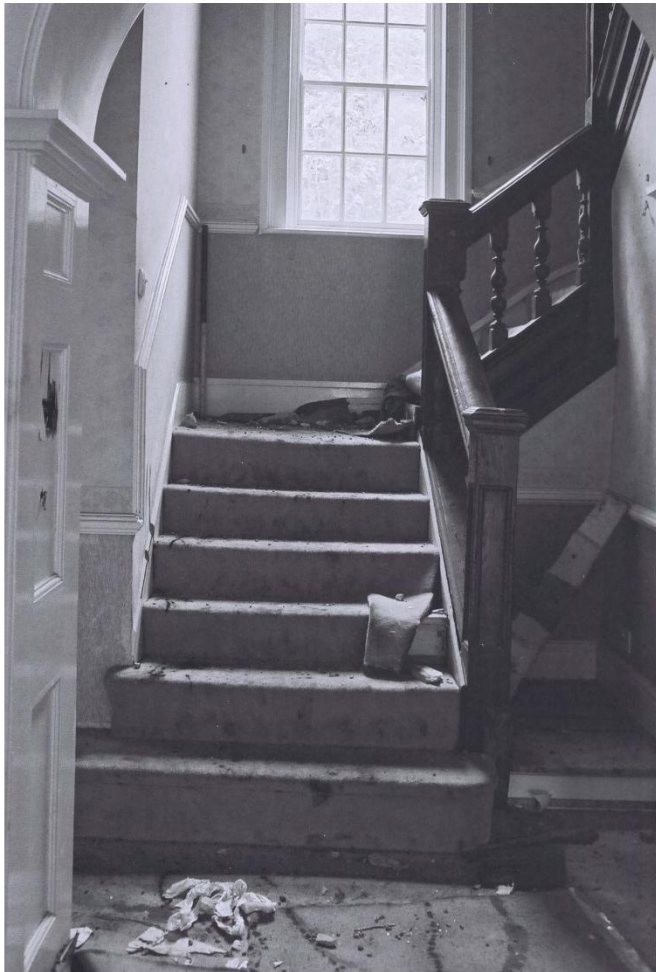
Plate 29. Staynor Hall: Interior Ground Floor. Facing North.
