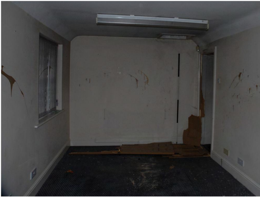
Plate 41. Staynor Hall: Interior First Floor. Facing South.
