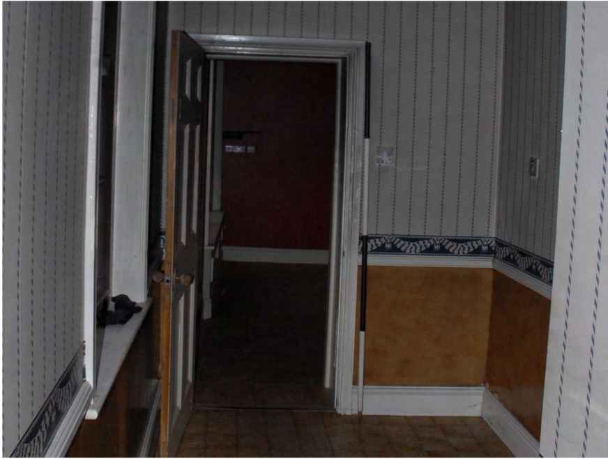
Plate 37. Staynor Hall: Interior Ground Floor. Facing North.
