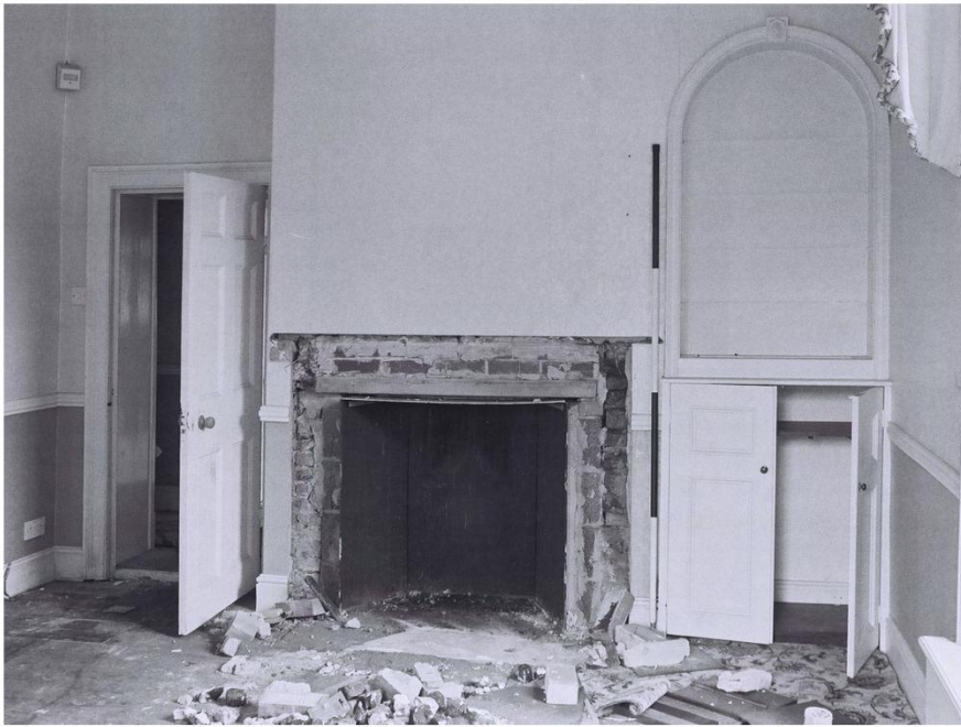
Plate 23. Staynor Hall: Interior Ground Floor. Facing North.
