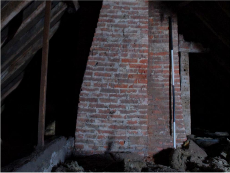
Plate 55. Staynor Hall: Interior Attic. Facing North.
