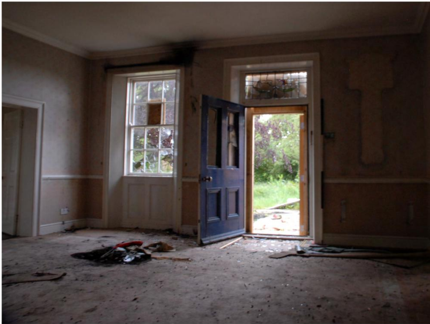
Plate 21. Staynor Hall: Interior Ground Floor. Facing South.
