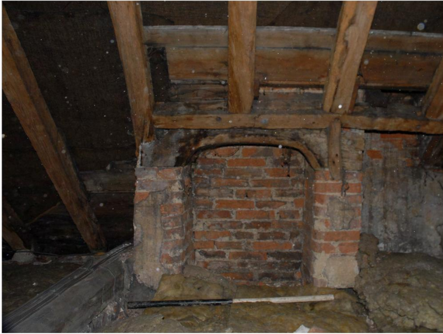
Plate 56. Staynor Hall: Interior Attic. Facing North.
