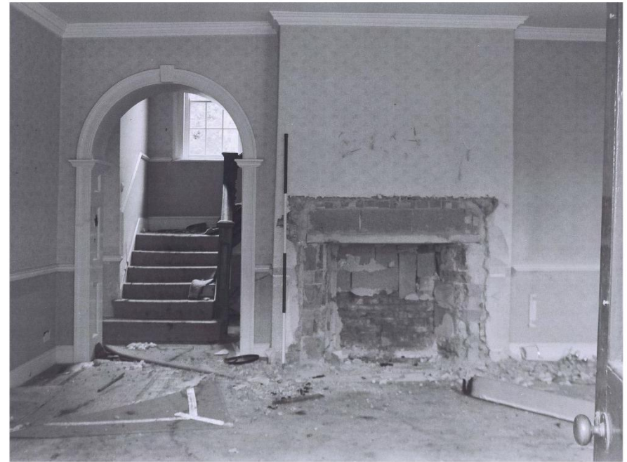
Plate 22. Staynor Hall: Interior Ground Floor. Facing North.
