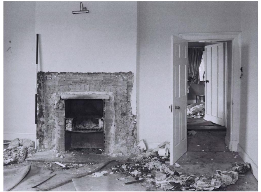
Plate 26. Staynor Hall: Interior Ground Floor. Facing North.
