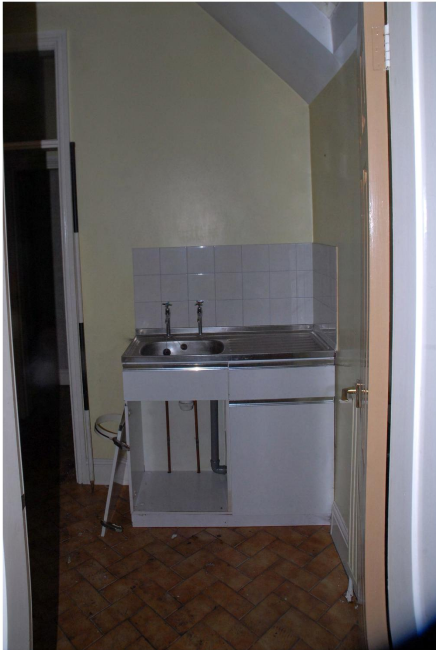
Plate 39. Staynor Hall: Interior Ground Floor. Facing North.
