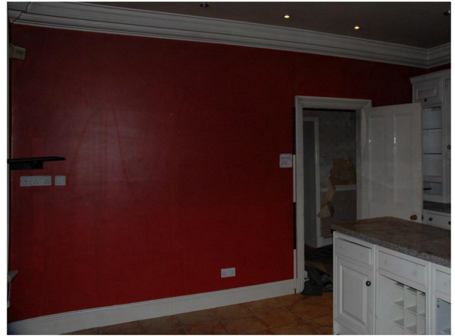
Plate 34. Staynor Hall: Interior Ground Floor. Facing South-west.
