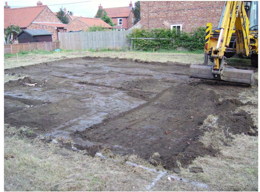
Plate 2. Topsoil Strip. Facing North-west.
