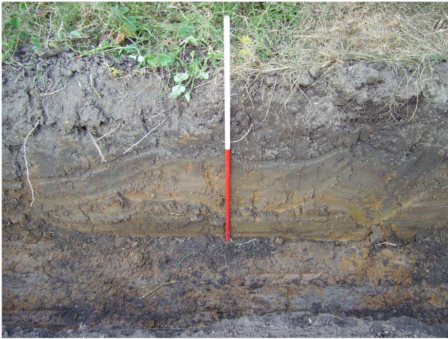
Plate 5. Garage Footings. Facing West.
