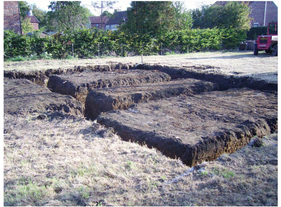
Plate 4. House Footings. Facing North-east.
