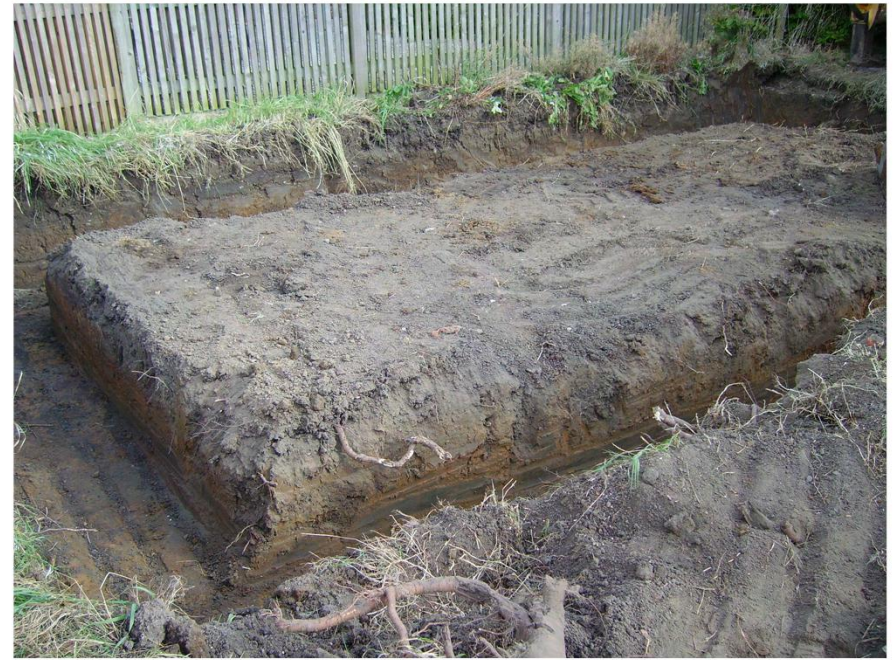
Plate 6. Garage Footings. Facing North-east.
