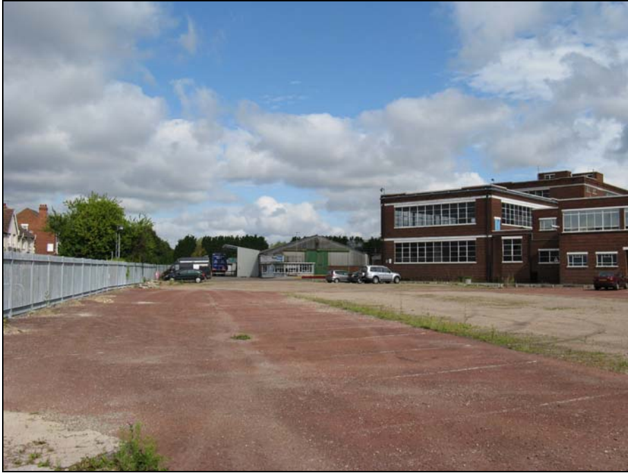
Figure 12 View westwards across the southern part of the site
