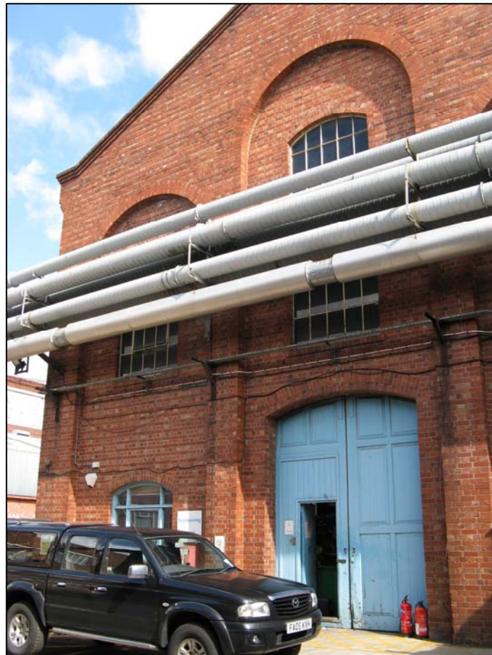
Figure 13 Brick buildings along the eastern boundary of the site
